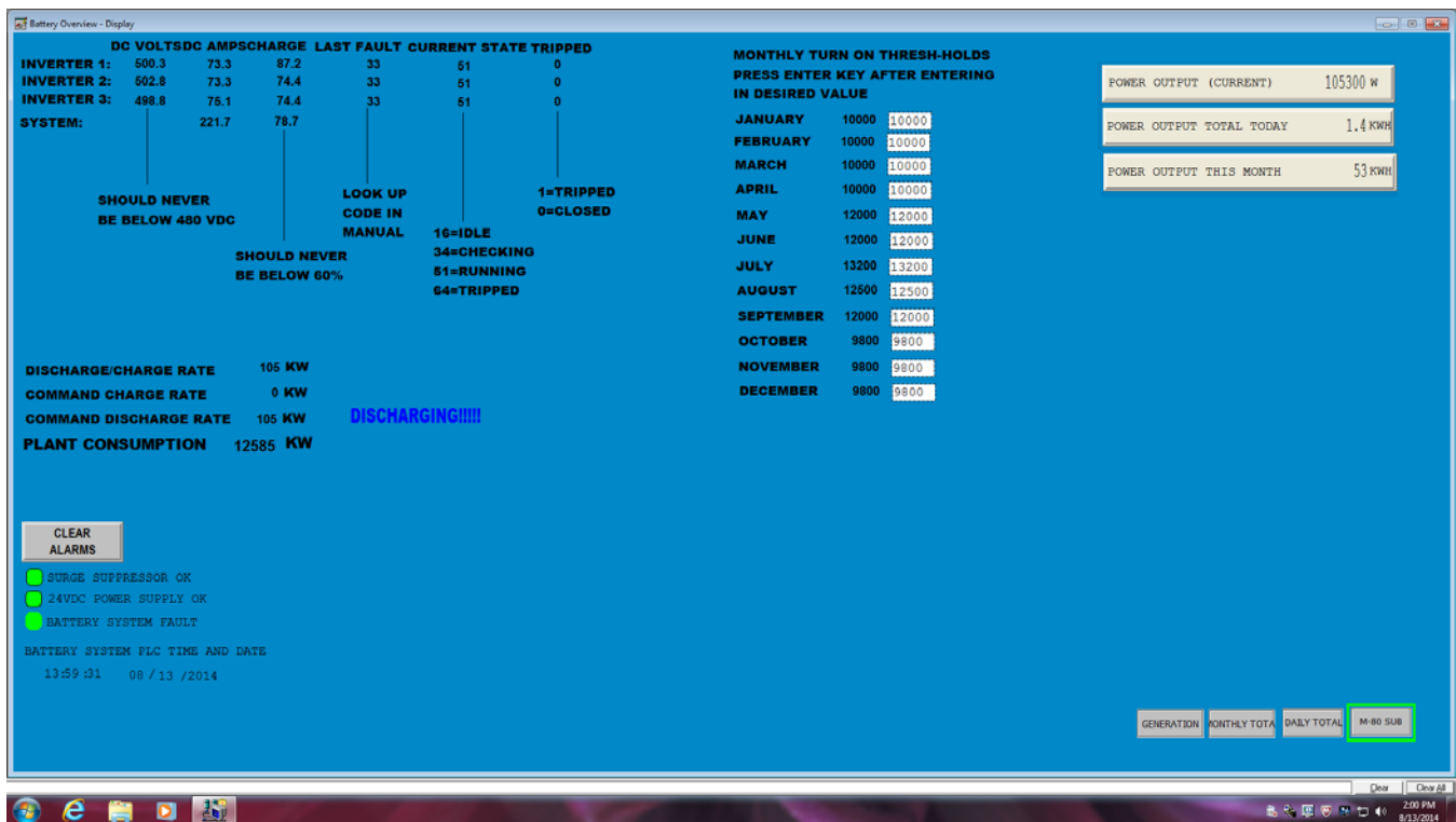
Figure 12 – Battery System Control Screen
