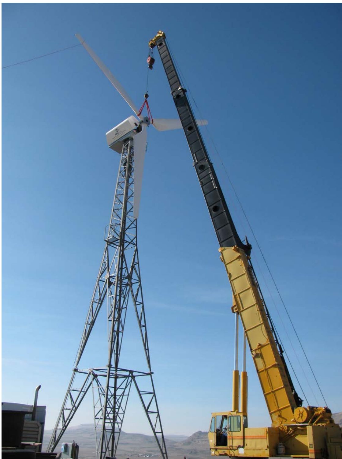
Figure 2 - Installation of 95 kW Wind Generator
