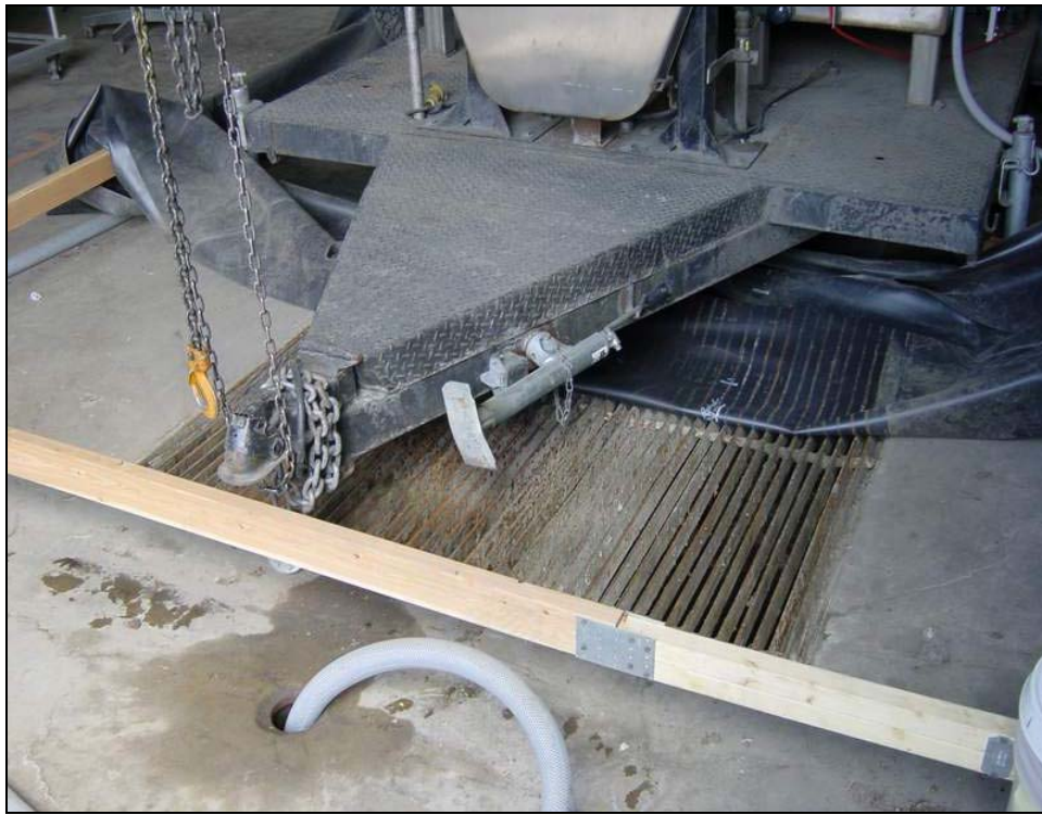
Figure 9. Steel grating covering sump. Regular discharge of the spent solution not containing cyanides bypasses the sump and is made directly to the sewer system. The Sump is located underneath the mobile unit. In emergency situations the sump serves as additional protection to prevent uncontrollable cyanide discharge to the sewer
