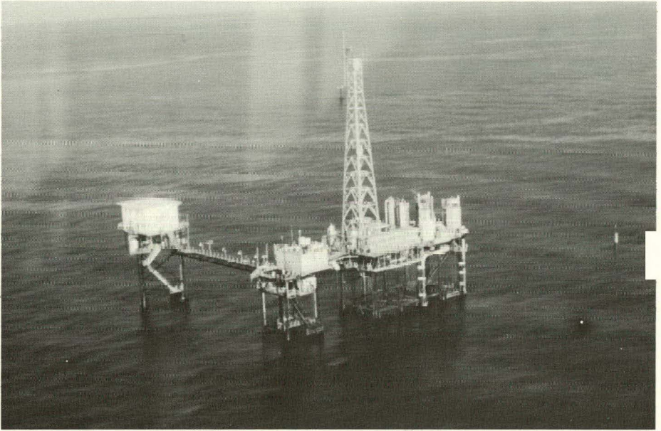
Figure 17. Facility installed in producing field offshore Louisiana.
