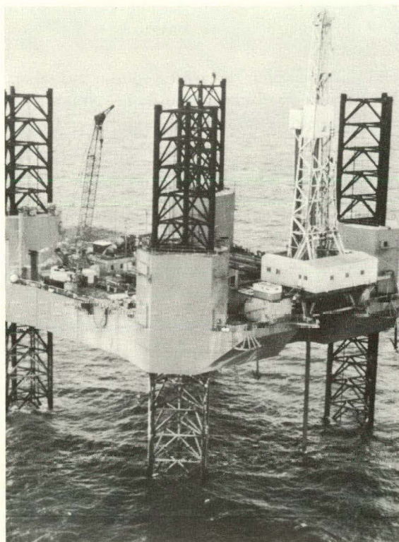
Figure 9. Jack-up rig in position.
