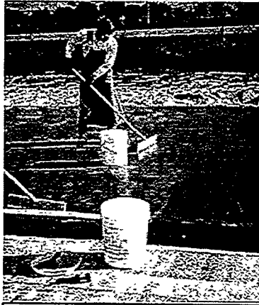
Figure 1. Worker applying PCRS to a surface using straight long-handled applicator.
