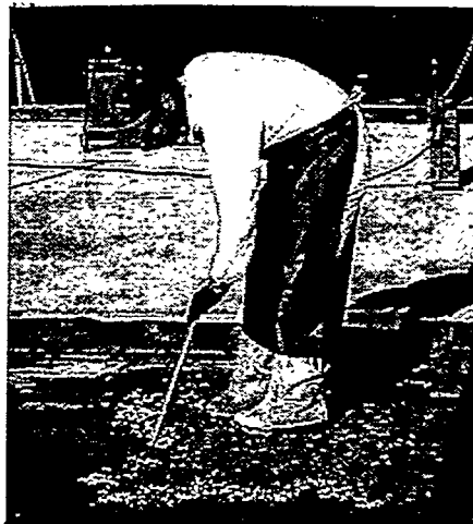
Figure 2. Worker using a long-handled paint scraper to remove chemical and surface coating.
