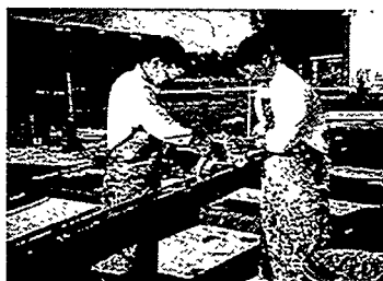
Figure 3. Workers removing chemical, laminated paper and coating from I-beams.
