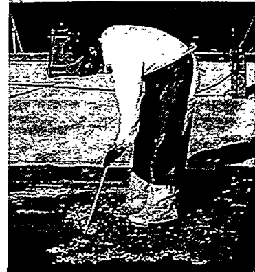
Figure 2. Worker using a long-handled paint scraper to remove chemical and surface coating.
