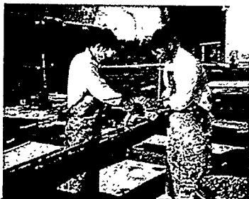
Figure 3. Workers removing chemical, laminated paper and coating from I-beams.
