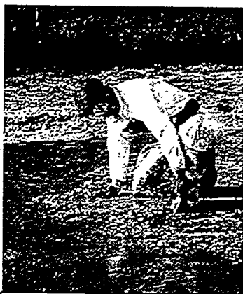
Figure 3. Worker kneeling on surface using a short-handled paint scraper to remove chemical and surface coating.
