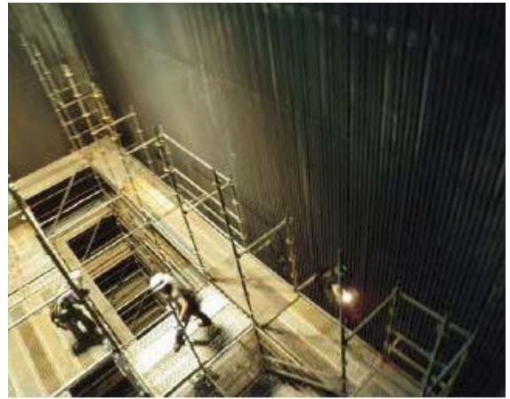
Figure 1: Hayden Unit 1 scaffolding for manual inspection and repair.
