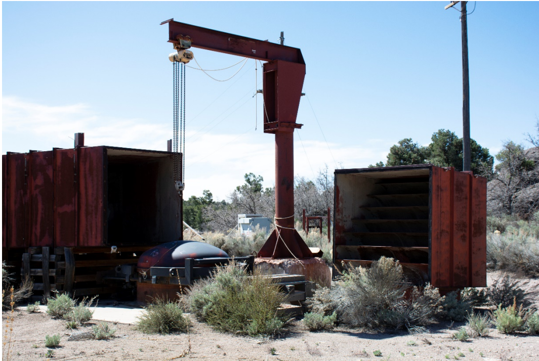
PHOTO NO. 5 PERSPECTIVE OF VENT CONDUIT, TUBE TURN CONTAINMENT DOOR, CRANE, AND CONDUIT ELBOW FACING THE SOUTHWEST
