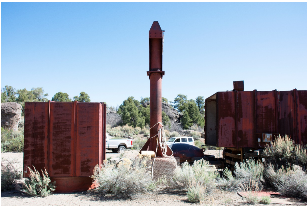
PHOTO NO. 2 GENERAL VIEW OF NORTH END WITH CONDUIT ELBOW, CRANE, TUBE TURN CONTAINMENT DOOR, AND VENT CONDUIT FACING THE NORTHEAST
