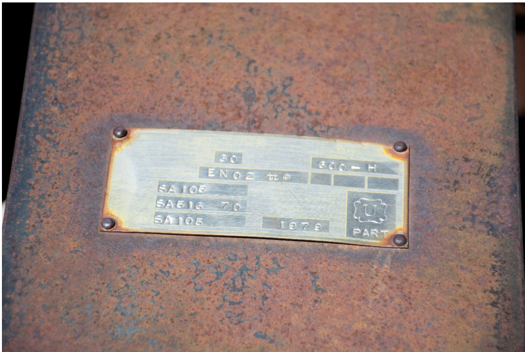
PHOTO NO. 10 CLOSER VIEW OF STEEL TAG ON CONTAINMENT DOOR FACING DOWN AND WEST
