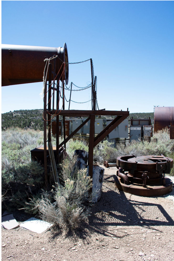
PHOTO NO. 4 CLOSER VIEW OF OVERHEAD WALKWAY AT WEST END OF VENT LINE FACING THE SOUTH
