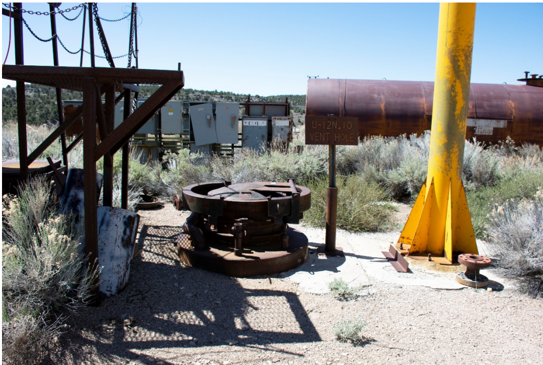
PHOTO NO. 2 CLOSER VIEW OF VENT PIPE AND TUBE TURN CONTAINMENT DOOR FACING THE SOUTH
