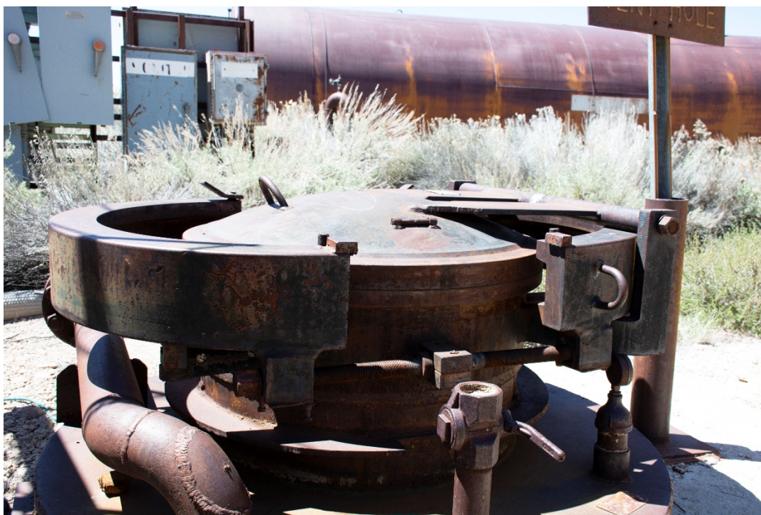
PHOTO NO. 8 CLOSER VIEW OF YOKE STYLE CLAMP CLOSURE MECHANISM FACING THE SOUTHWEST
