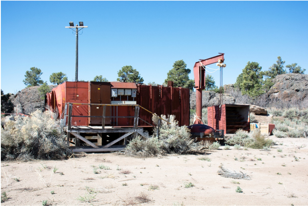
PHOTO NO. 1 GENERAL VIEW FACING THE WEST
