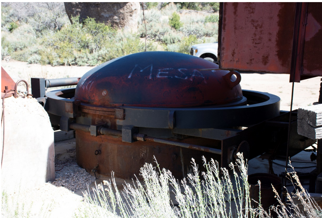
PHOTO NO. 14 CLOSER VIEW OF VENT PIPE AND CONTAINMENT DOOR YOKE STYLE CLAMP CLOSURE MECHANISM FACING THE NORTH
