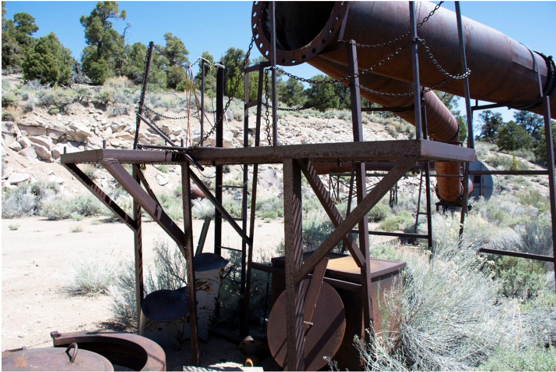
PHOTO NO. 5 PERSPECTIVE VIEW OF OVERHEAD PLATFORM FACING THE NORTHEAST
