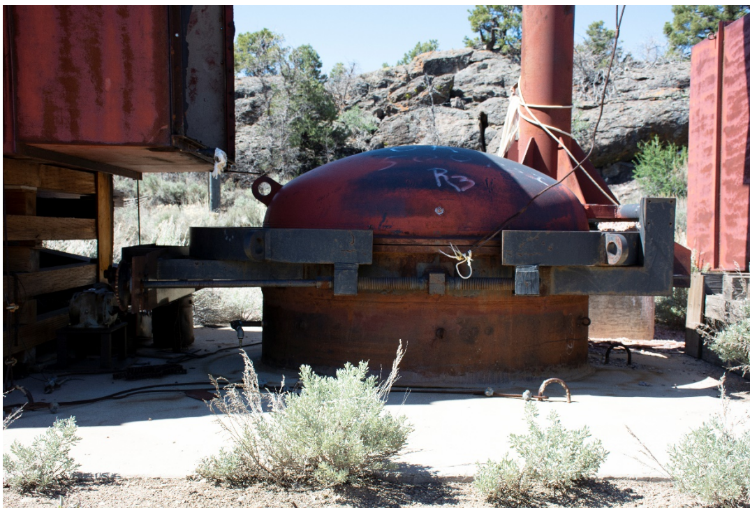
PHOTO NO. 9 CLOSER VIEW OF TUBE TURN CONTAINMENT DOOR WITH YOKE STYLE CLOSURE MECHANISM FACING THE SOUTHWEST
