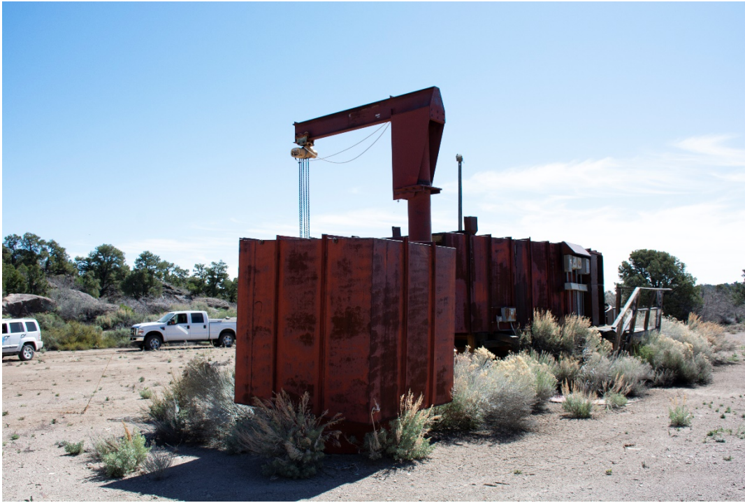
PHOTO NO. 3 PERSPECTIVE OF CONDUIT ELBOW, CRANE AND VENT CONDUIT FACING THE EAST
