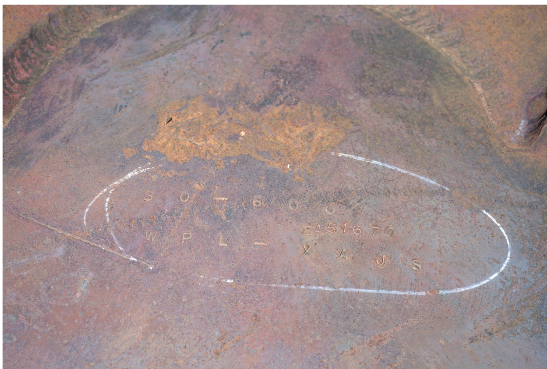
PHOTO NO. 9 CLOSER VIEW OF TUBE TURN CONTAINMENT DOOR FACING DOWN AND WEST
