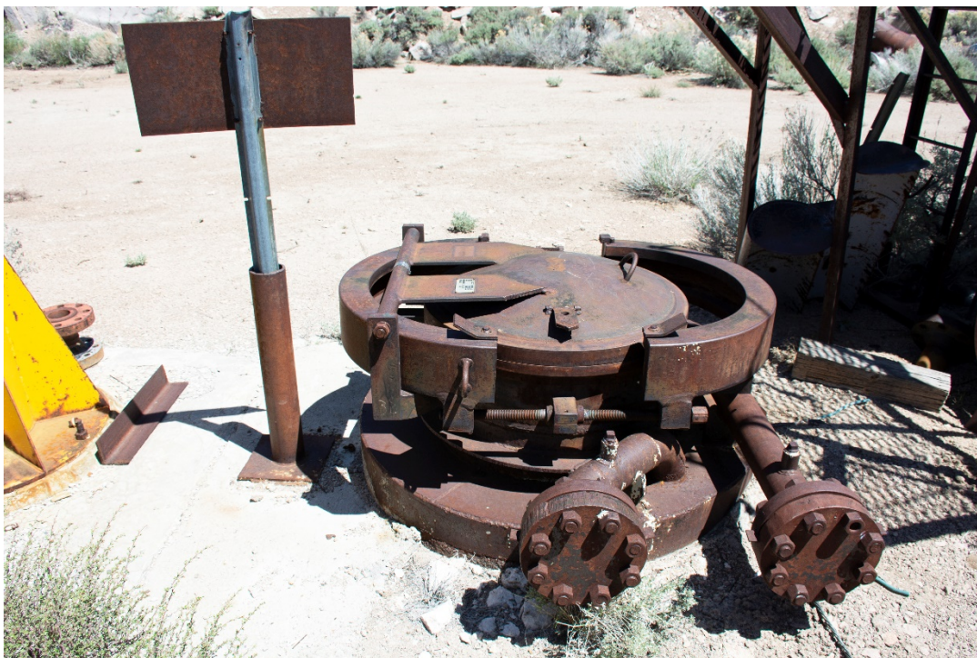
PHOTO NO. 11 CLOSER VIEW OF TUBE TURN CONTAINMENT DOOR WITH CHILLED WATER LINES EXTENDING SOUTH, FACING THE NORTH
