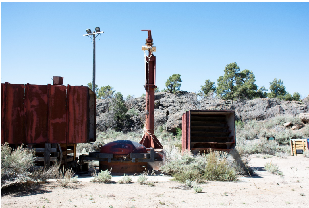
PHOTO NO. 6 GENERAL VIEW OF NORTH END WITH VENT CONDUIT, TUBE TURN CONTAINMENT DOOR AND VENT PIPE, CRANE, AND CONDUIT ELBOW FACING THE SOUTHWEST
