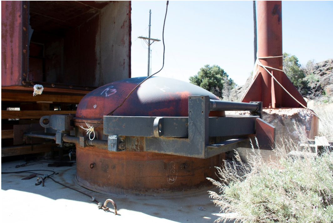
PHOTO NO. 13 CLOSER VIEW OF YOKE STYLE CLAMP CLOSURE MECHANISM FACING THE SOUTH
