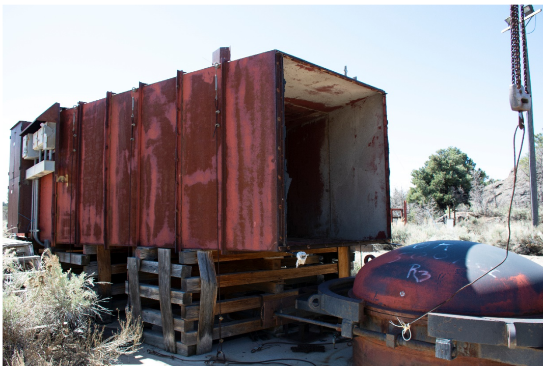
PHOTO NO. 7 CLOSER VIEW OF VENT CONDUIT AND WOOD CRIBBING SUPPORTS FACING THE SOUTHWEST
