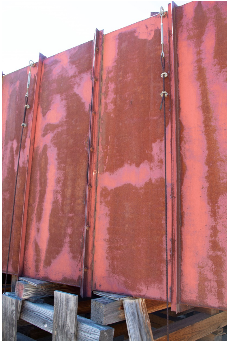
PHOTO NO. 8 CLOSER VIEW OF TIE DOWNS AND CONSTRUCTION DETAILS OF VENT CONDUIT FACING THE SOUTHWEST
