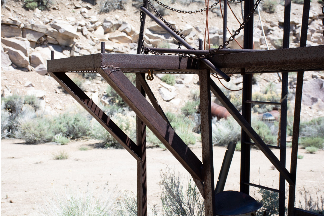
PHOTO NO. 6 CLOSER VIEW OF OVERHEAD WALKWAY EXTENSION TO THE WEST FACING THE NORTHEAST
