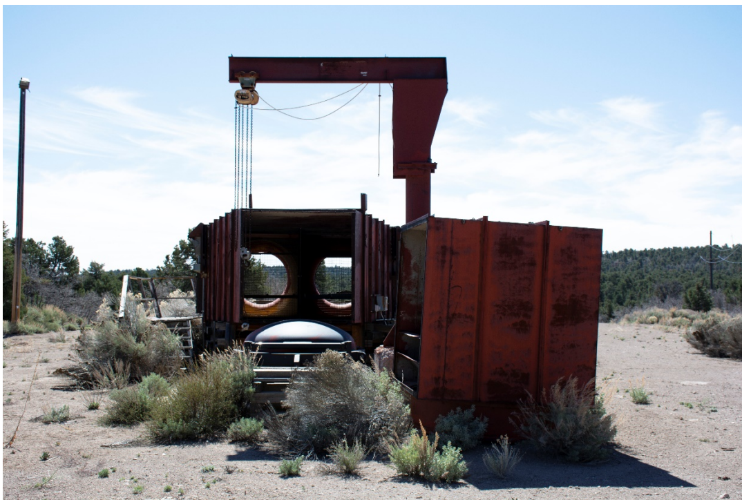
PHOTO NO. 4 GENERAL VIEW OF NORTH END WITH CONDUIT ELBOW, CRANE, TUBE TURN CONTAINMENT DOOR, AND VENT CONDUIT FACING THE SOUTHEAST
