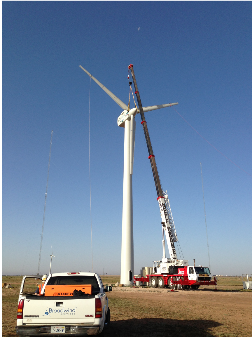
Figure 1.1. Installation of OEM rotor during SWiFT facility construction
