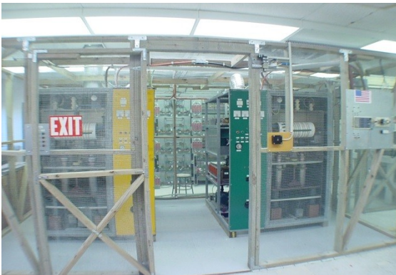
800 kW RF Power Generators
