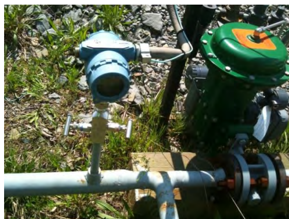
Figure 22. MH-20 CO 2 vapor injection line (flow right-to-left) detailing the control valve and flow meter locations.
