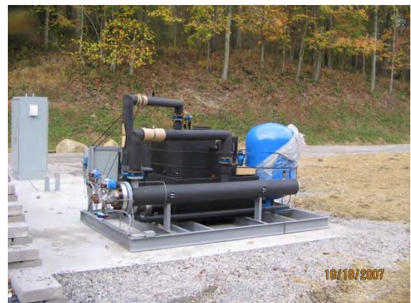
Figure 20. CO 2 vaporizer skid with the shell-in-tube heat exchanger in the foreground.
