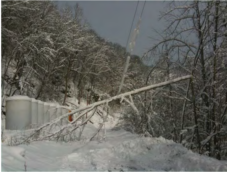
Figure 54. Inclement weather, downed trees, frequent site inaccessibility, and electrical service interruptions were limiting factors for the injection rate.
