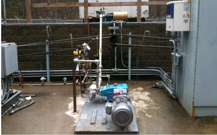
Figure 23. The replacement triplex pump (blue in foreground) with booster pump (gold in background), shortly after installation.
