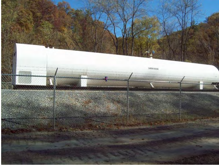
Figure 18. The 50-ton CO 2 storage tank, following installation.
