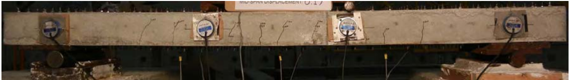
(a) flexure cracks at Total Load of 15-kips
