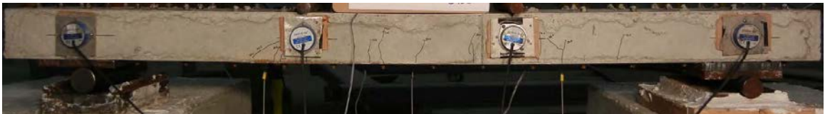
(b) Shear Cracks at Total Load of 25-kips
