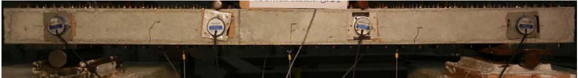
(a) flexure cracks at Total Load of 10-kips
