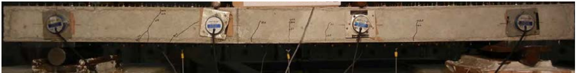
(b) Shear Cracks at Total Load of 20-kips
