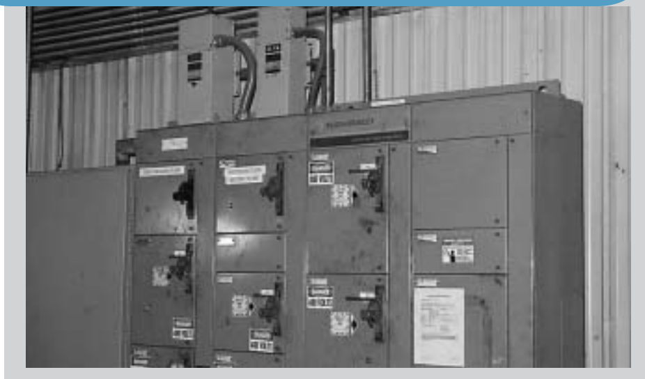
CAPACITORS INSTALLED AT LOMA SAW MOTOR CONTROL CENTER
