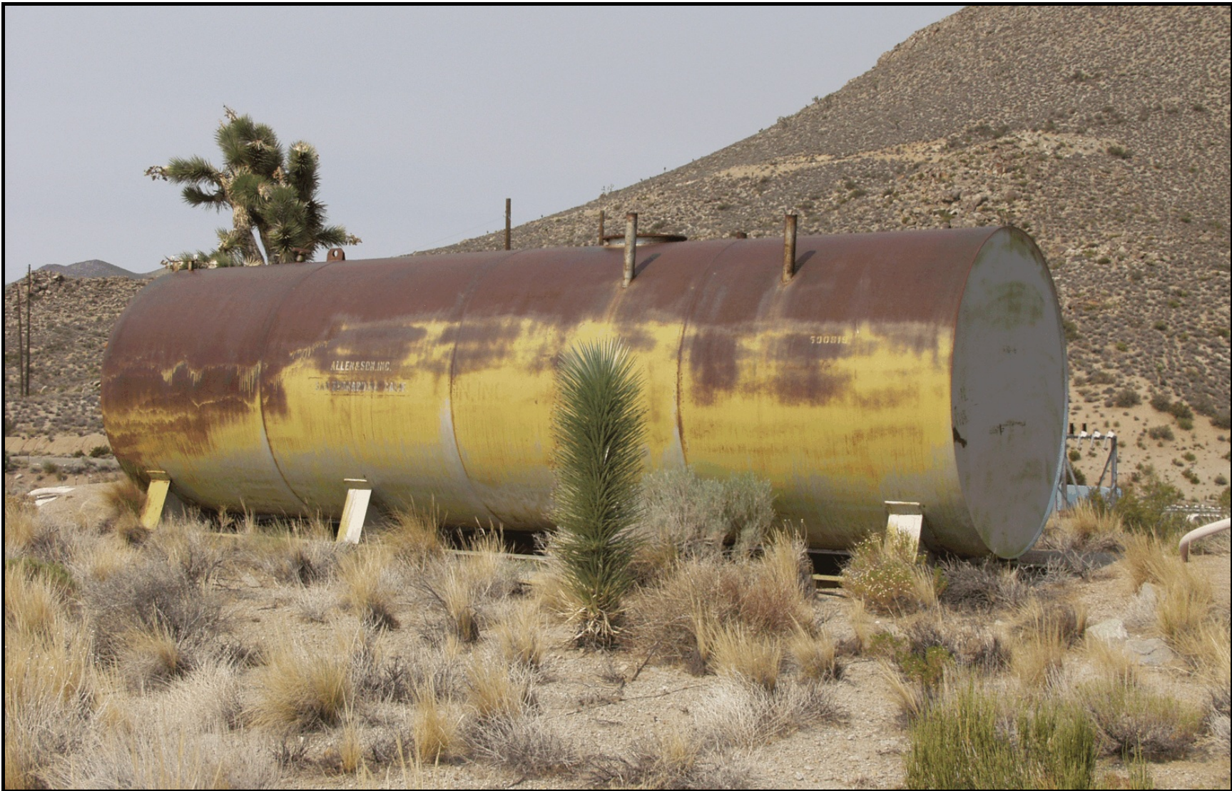
Figure 208. Feature 52, south water tank, view southwest (2013).
