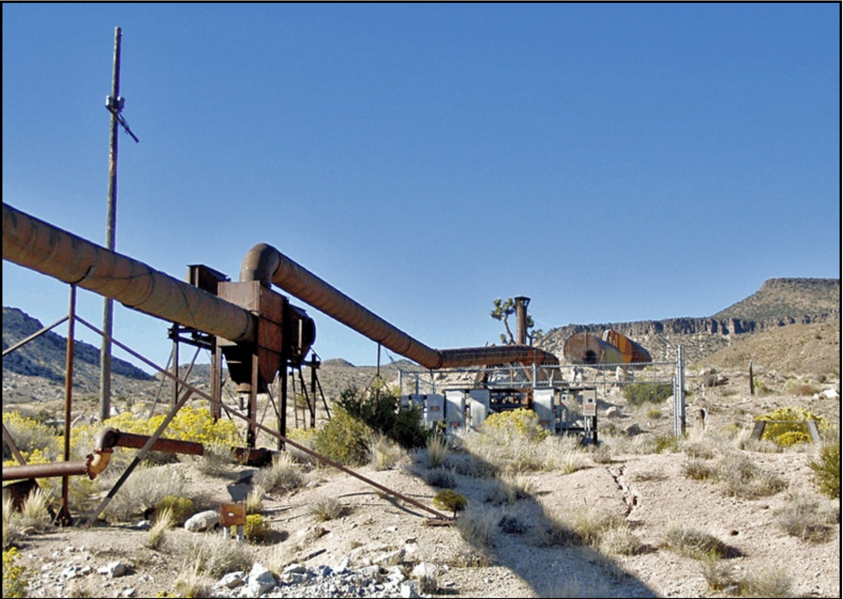
Figure 183. Feature 34, electric substation, view north (photograph on file).
