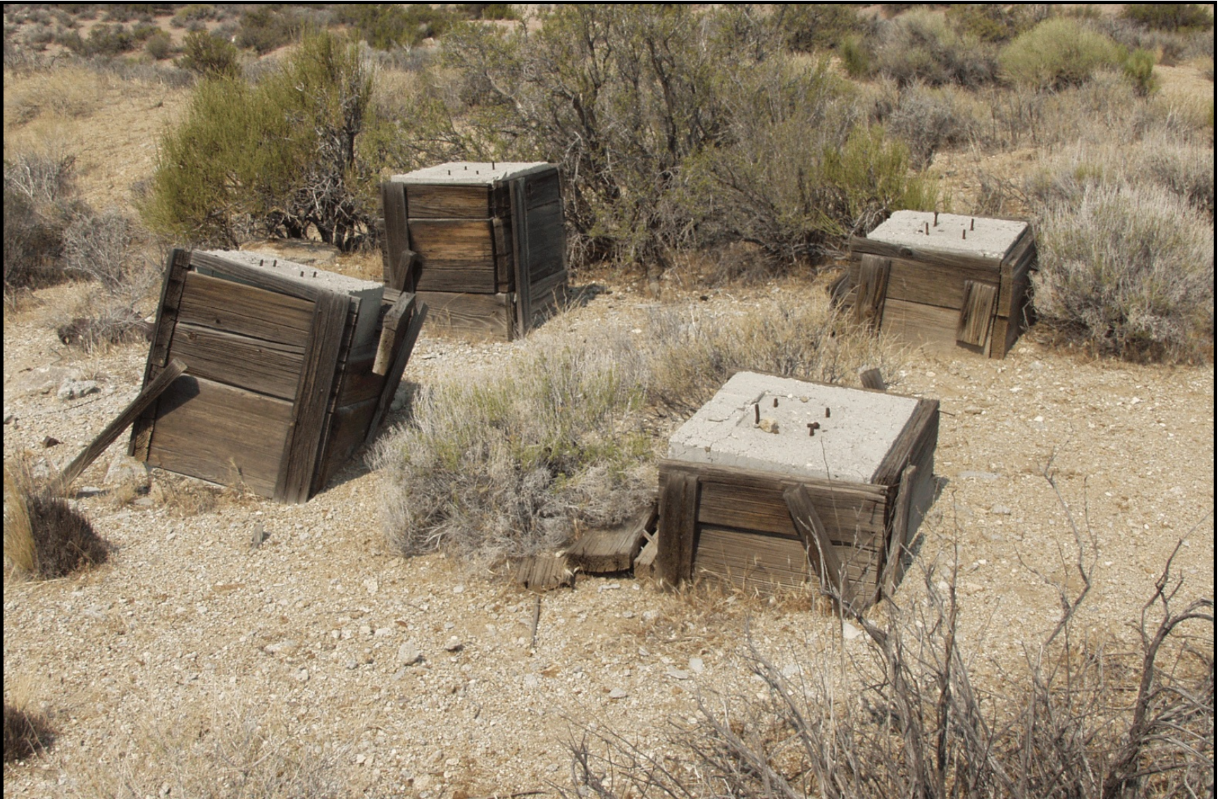
Figure 215. Feature 56, concrete piers, view northwest (2013).
