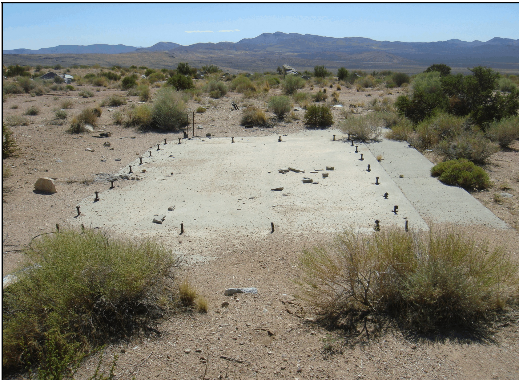
Figure 158. Feature 13, concrete pad for the U15e hoist house, view southeast (2011).
