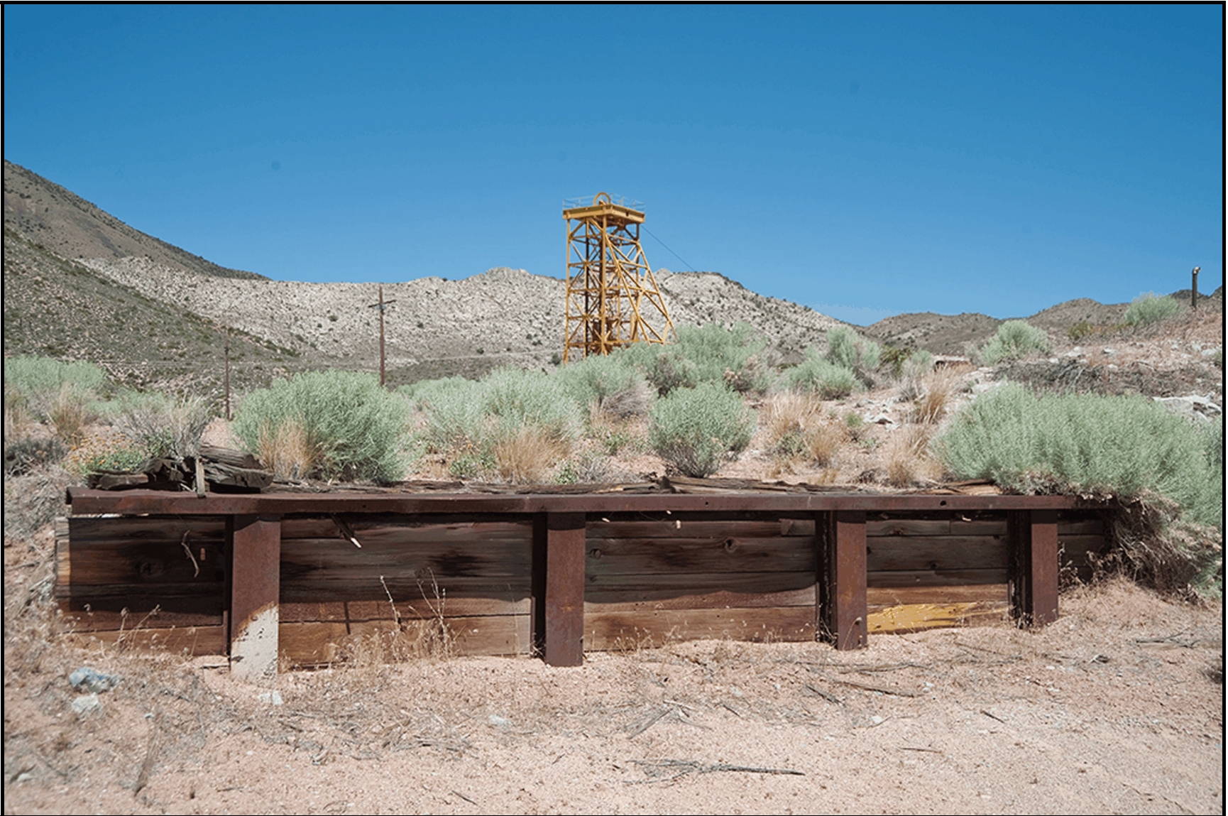
Figure 160. Feature 15, loading ramp, view northwest (photograph D10-2882, dated 2010, on file at the Remote Sensing Laboratory).
