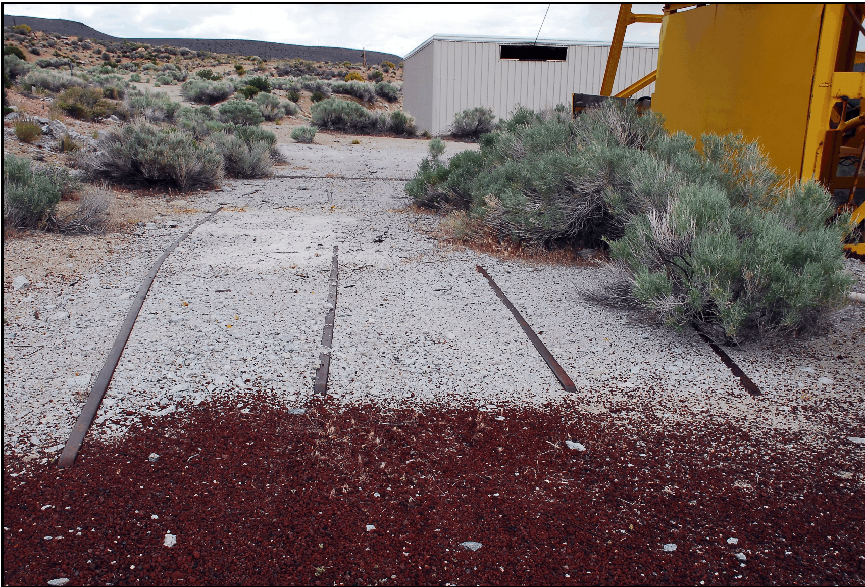
Figure 179. Feature 32, rail lines on north side of Structure 1, view east (2013).
