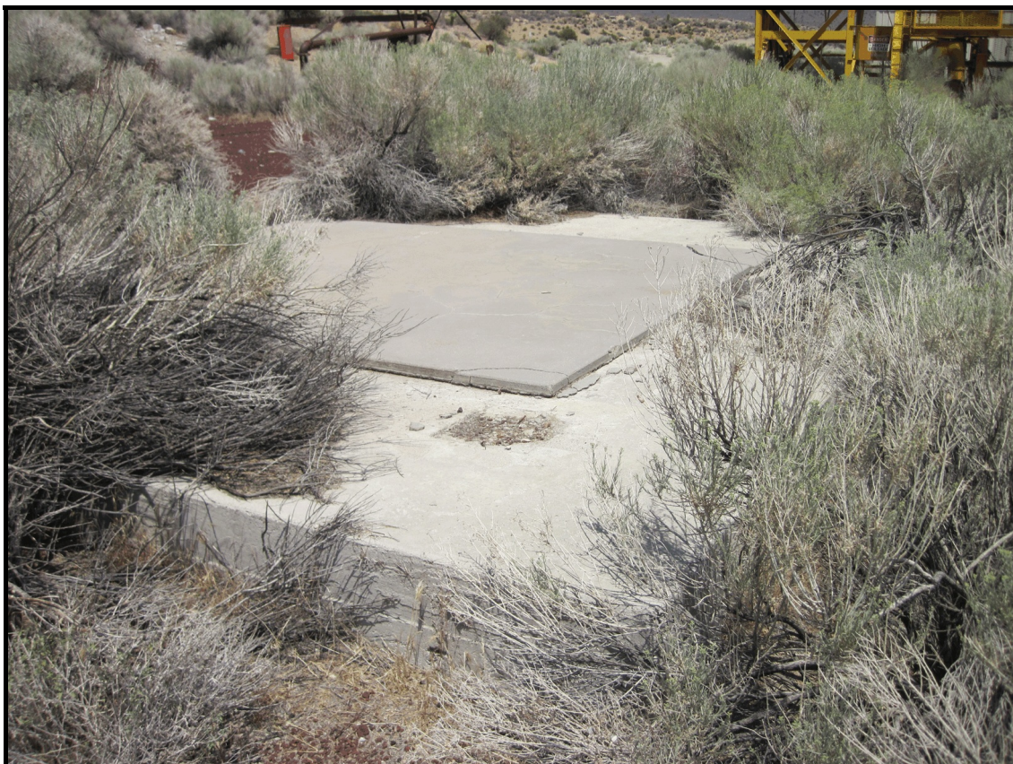
Figure 178. Feature 31, concrete pads, view northeast (2013).
