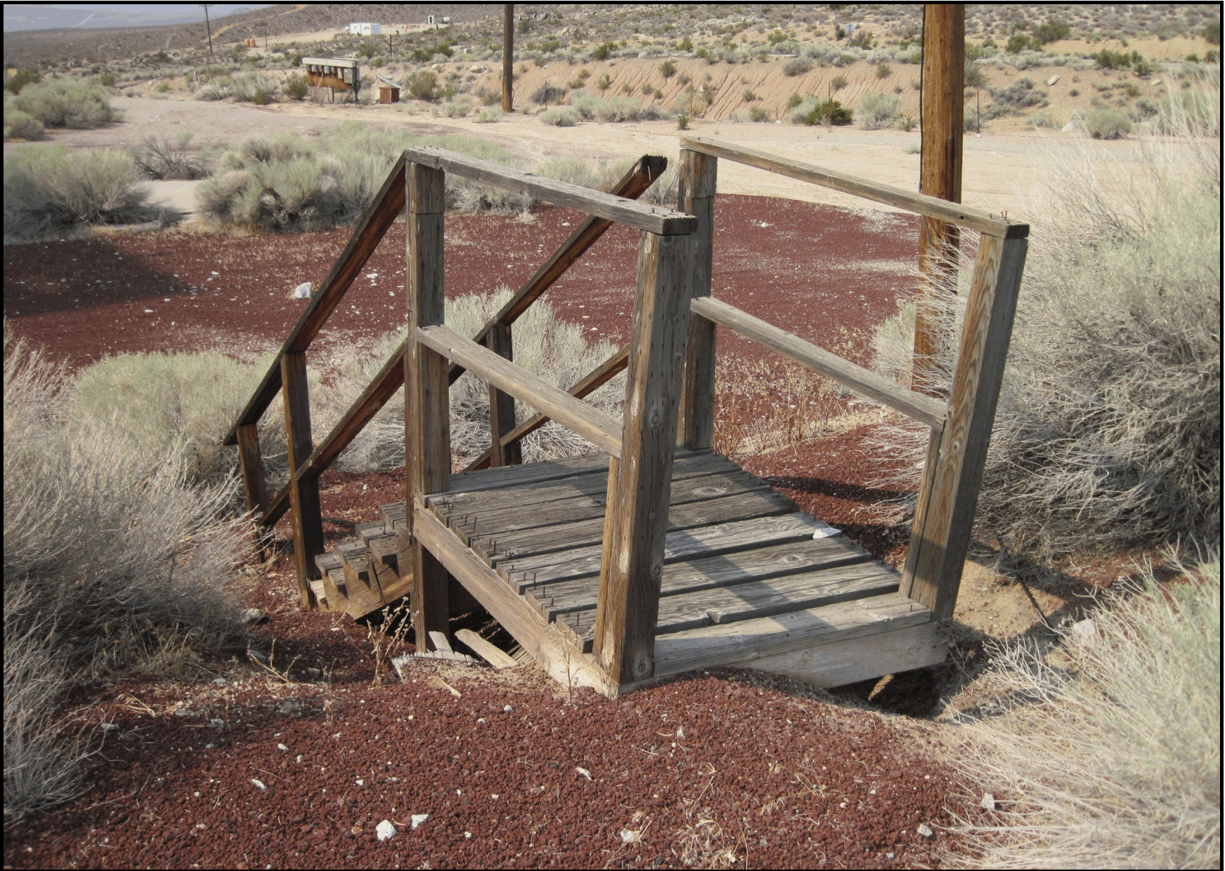
Figure 193. Feature 41, wooden stairs, view southwest (2013).
