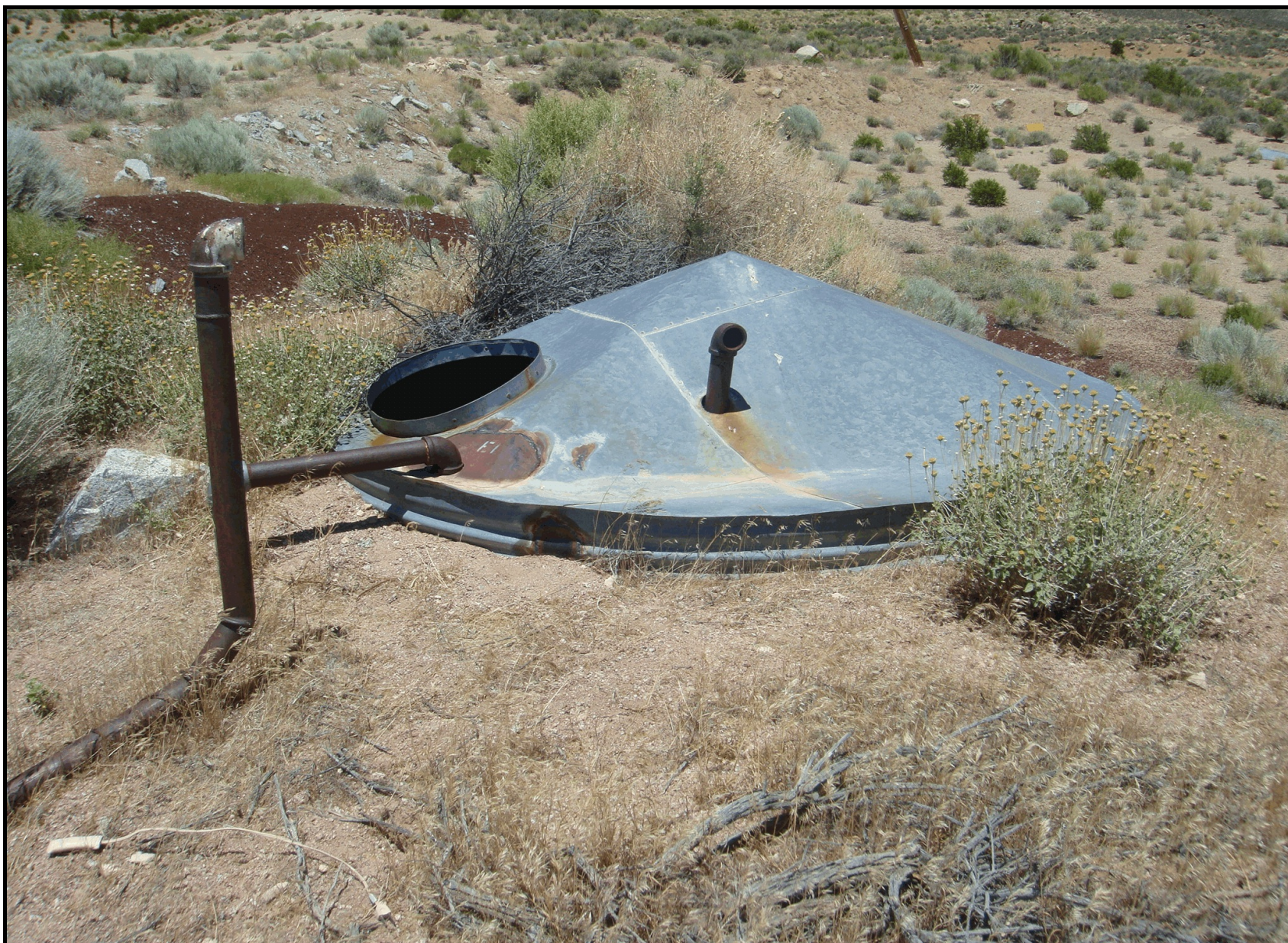
Figure 162. Feature 16, leaching tank for the Tiny Tot nuclear test, view northeast (2011).
