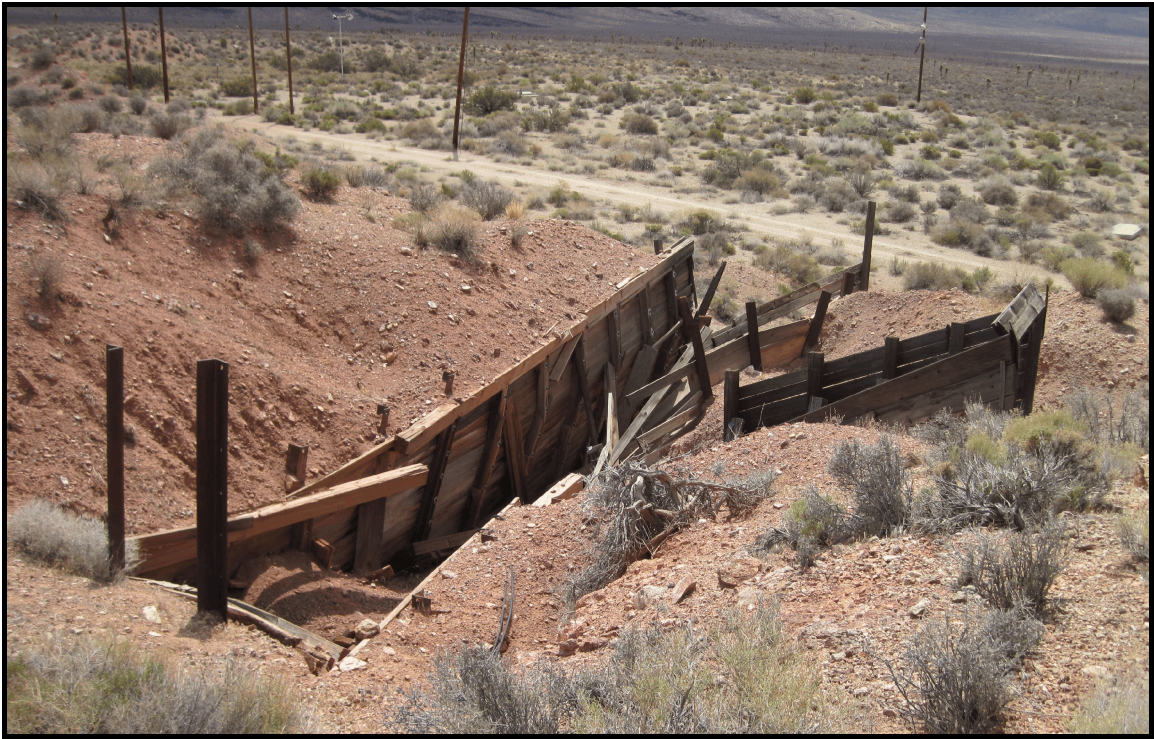
Figure 134. Structure 3, revetment trench, view southeast (2013).
