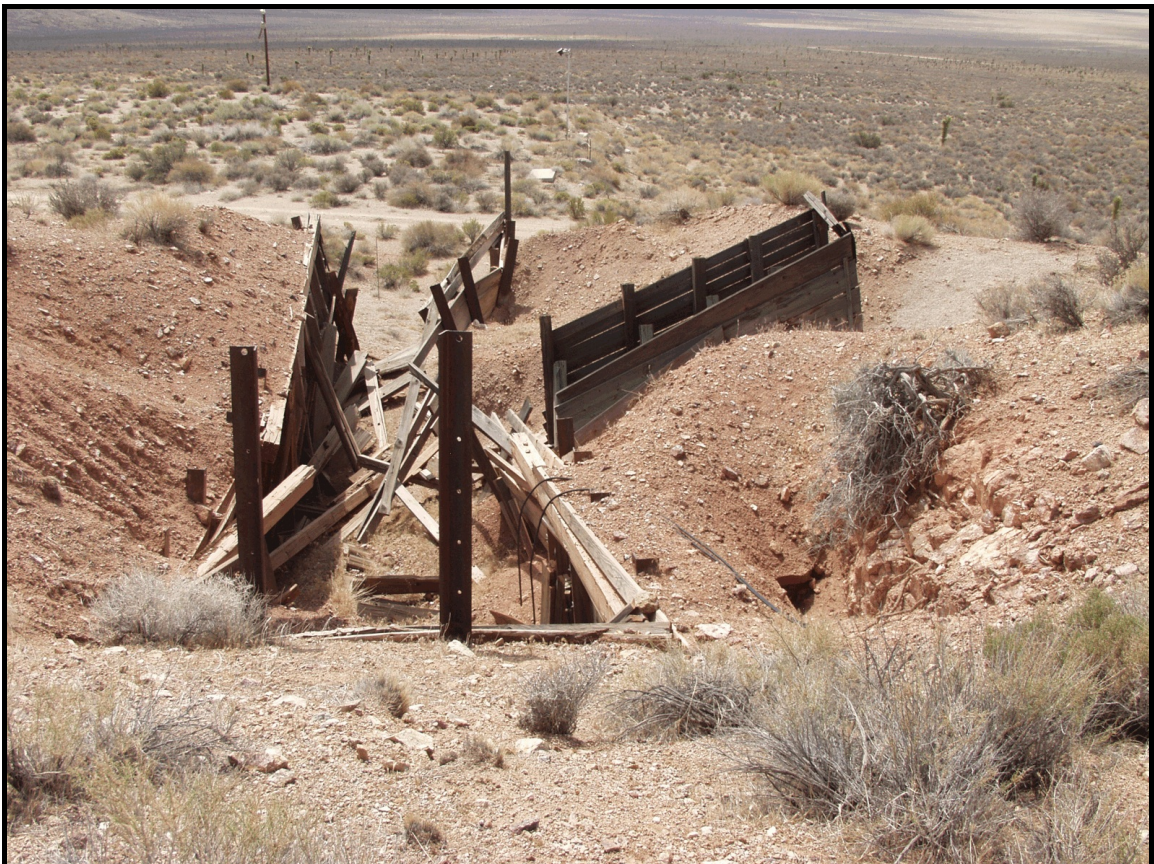
Figure 135. Structure 3, revetment trench, view south (2013).
