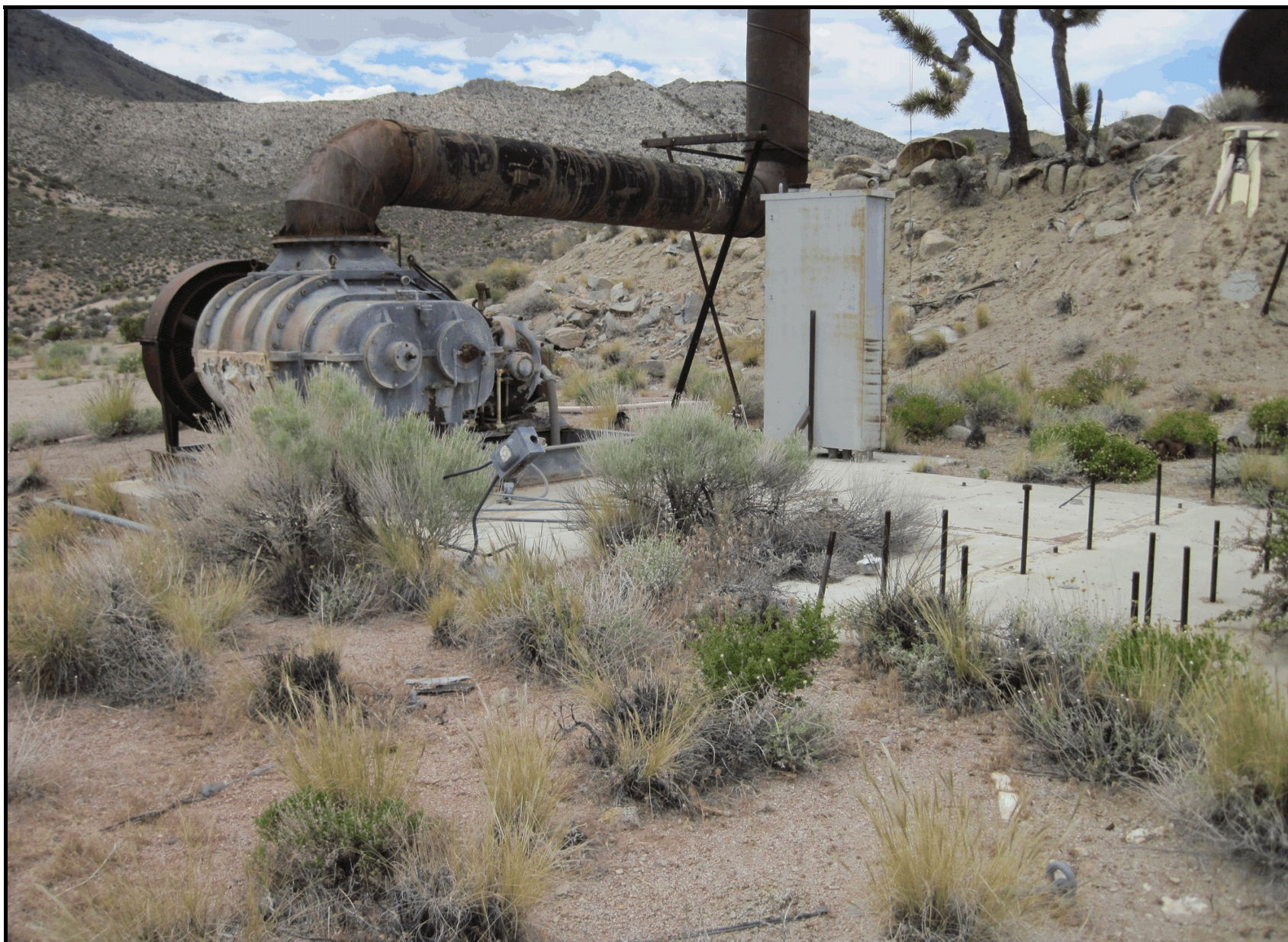
Figure 190. Feature 38, blower pad, view northwest (2013).
