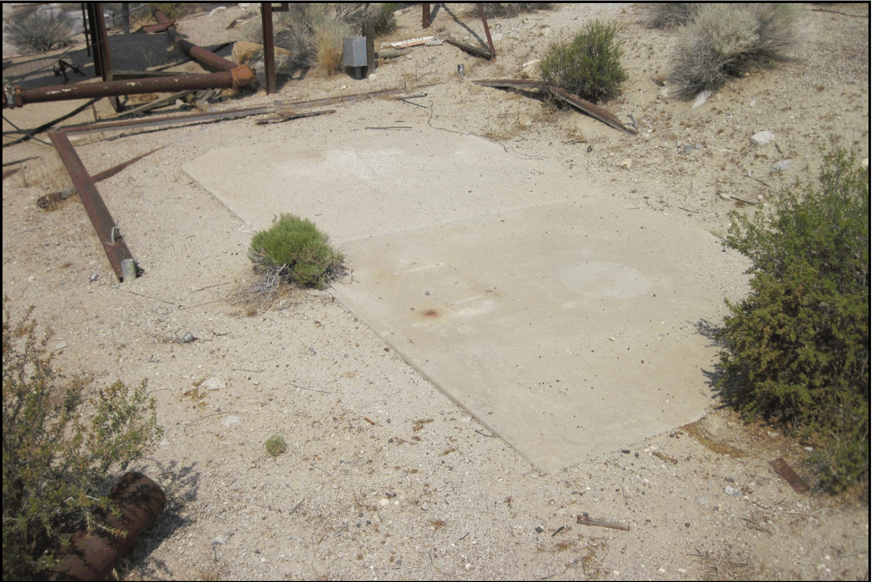
Figure 182. Feature 34, electric substation, view west (2013).
