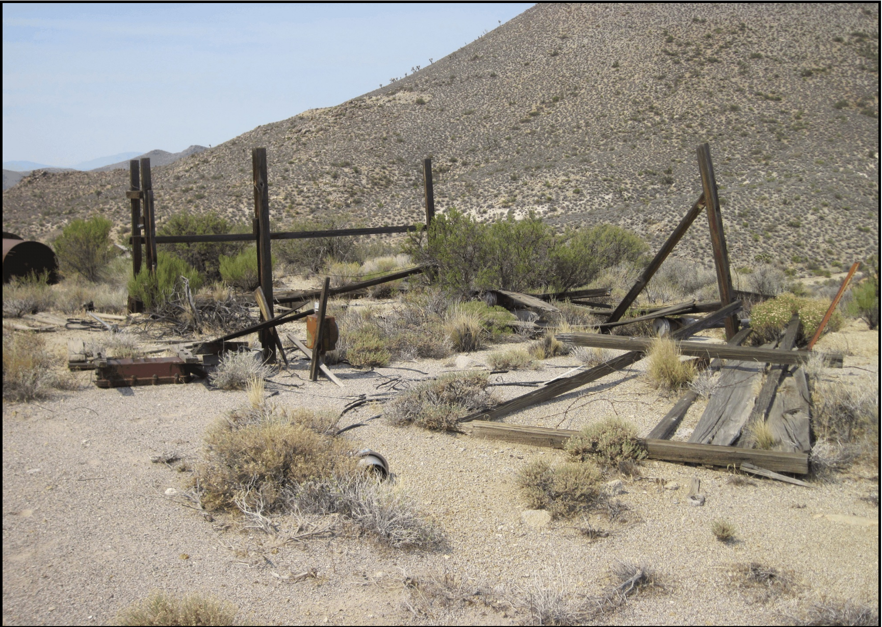
Figure 213. Feature 54, electric substation in U15a area, view southwest (2013).
