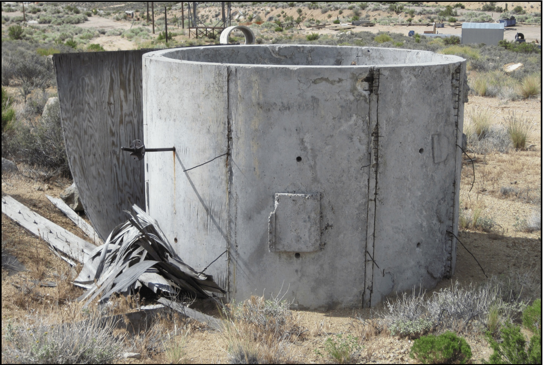
Figure 207. Feature 51, concrete experiment section, view southwest (2013).
