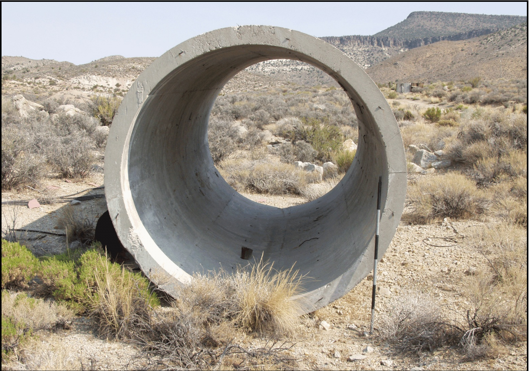
Figure 205. Feature 50, concrete experiment section, view northwest (2013).
