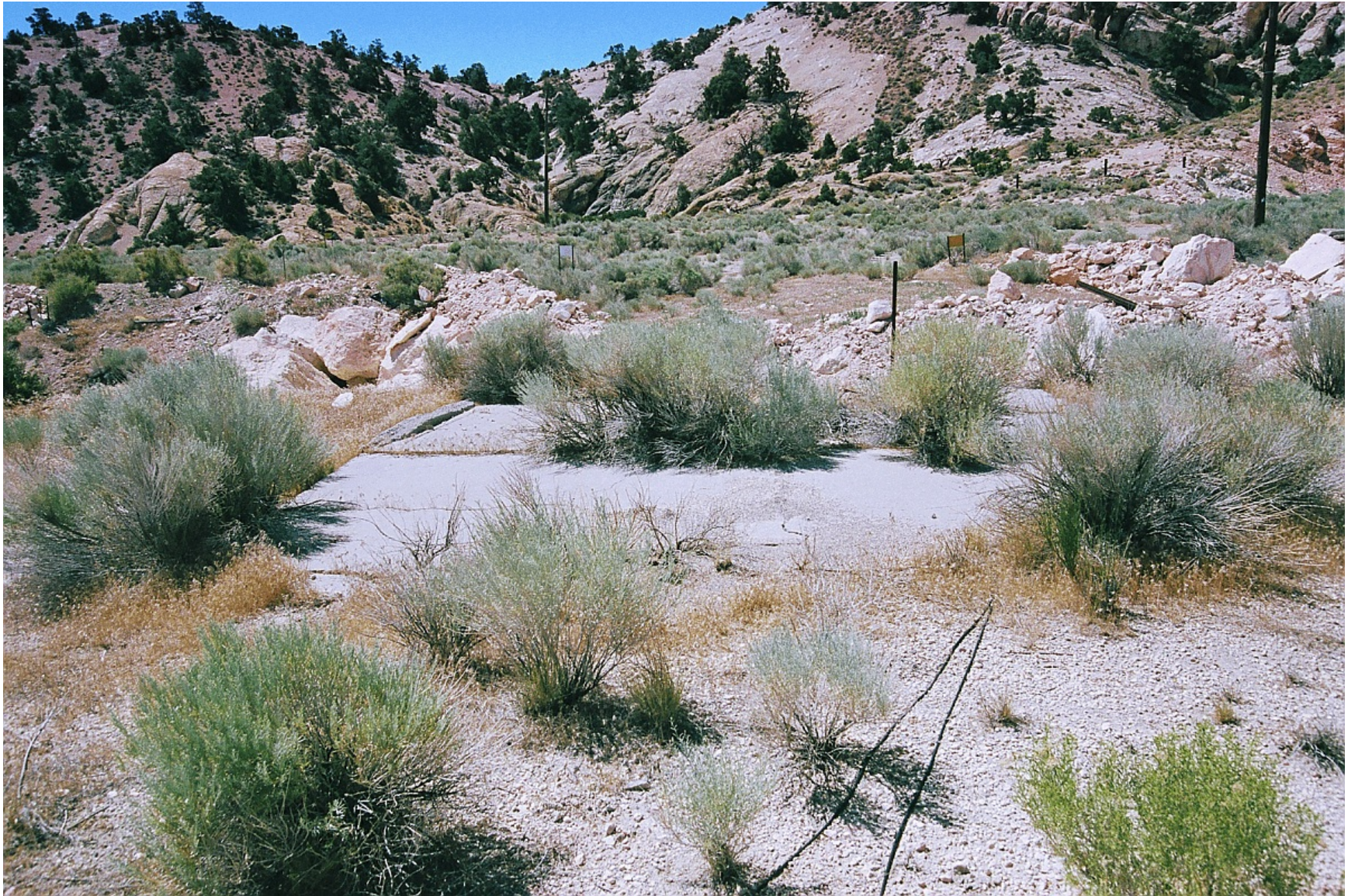
Figure 54. U16a Tunnel Feature 12 construction shop pad, view southwest (2011).
