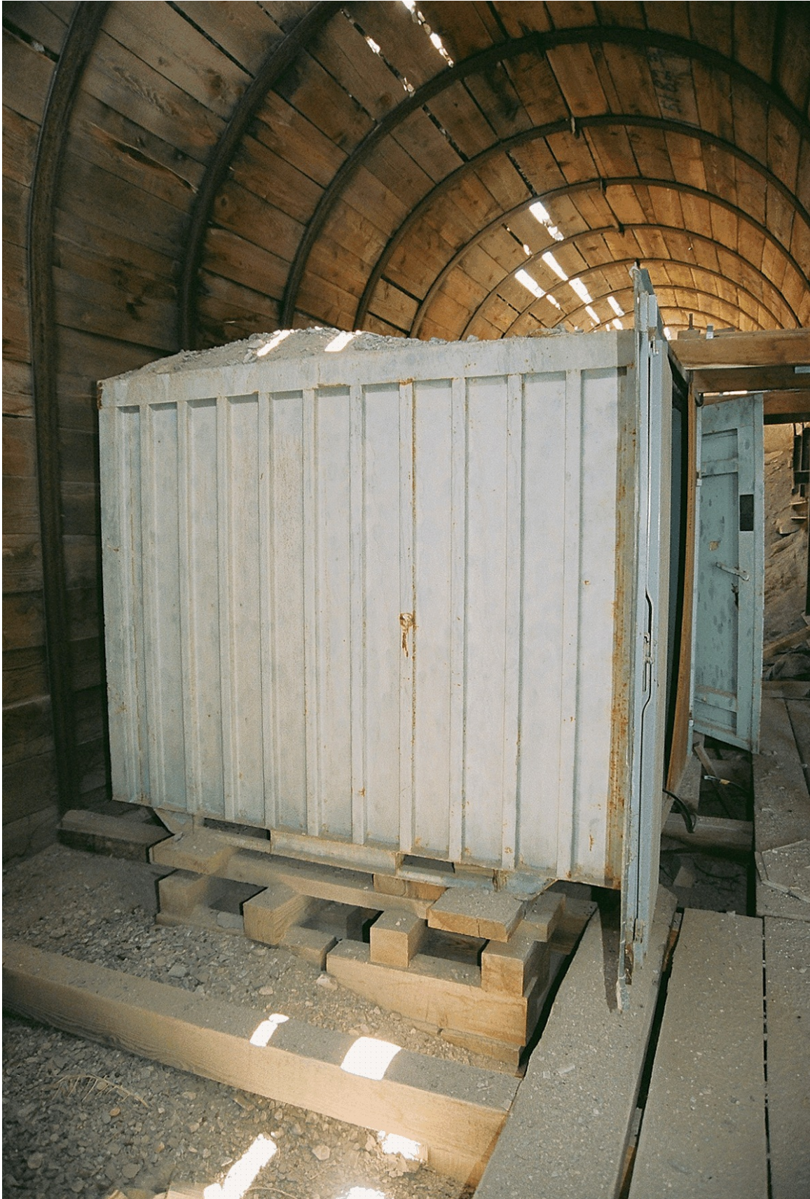
Figure 96. U16a Tunnel Feature 39 Structure 10, containers, view southwest (2011).
