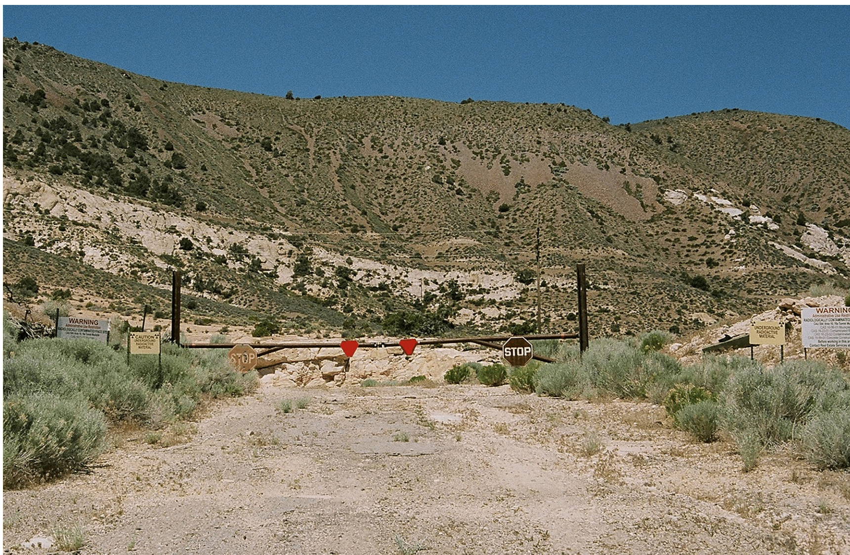
Figure 56. U16a Tunnel Feature 14, barricade (2011).
