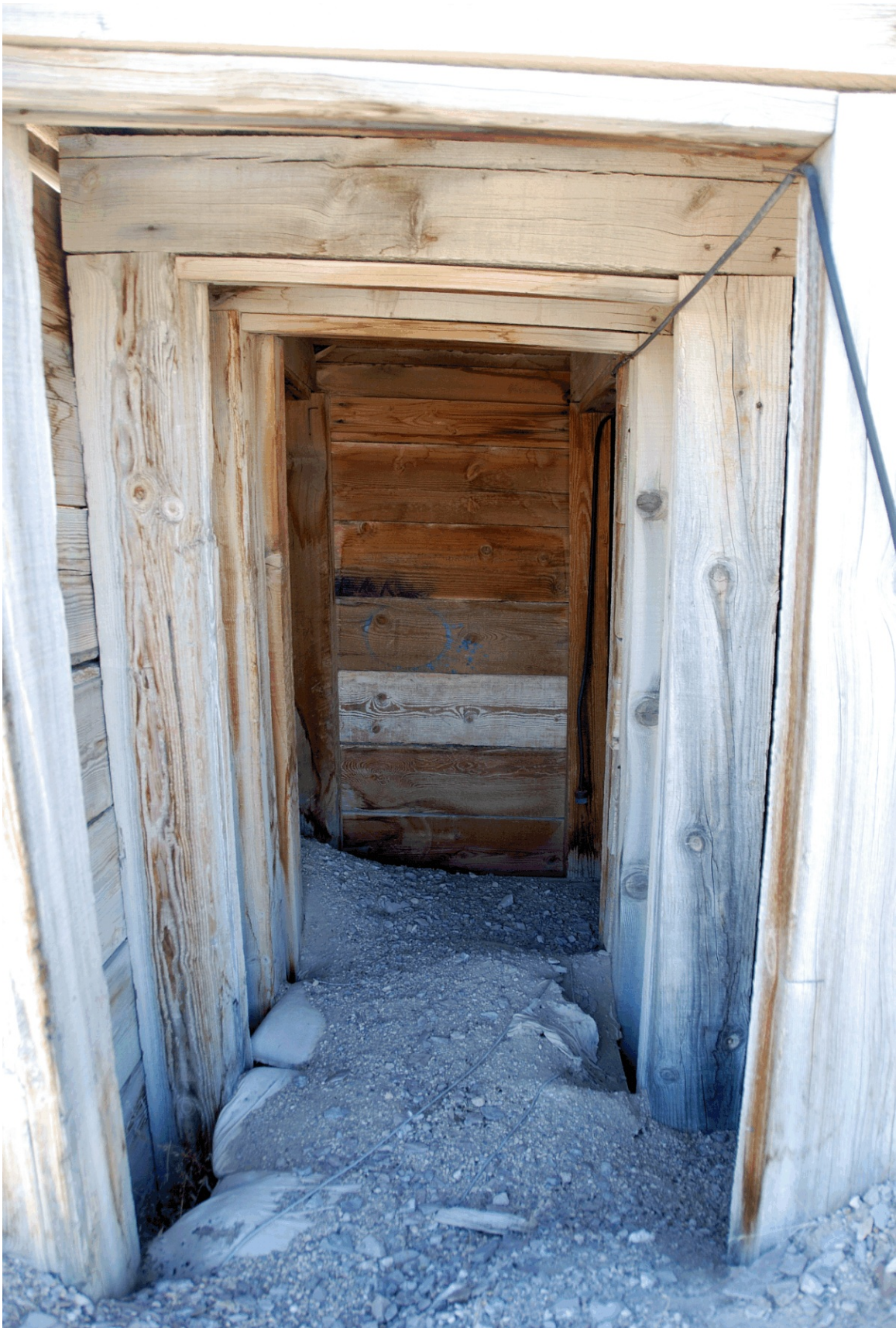
Figure 95. U16a Tunnel Feature 39 Structure 10, entry, view southwest (2011).
