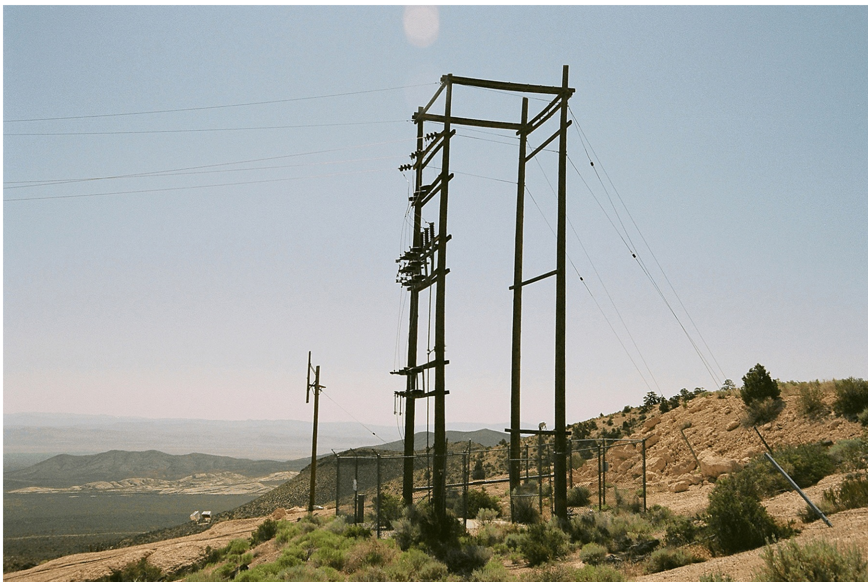
Figure 67. U16a Tunnel Feature 24, electrical substation, view southeast (2011).
