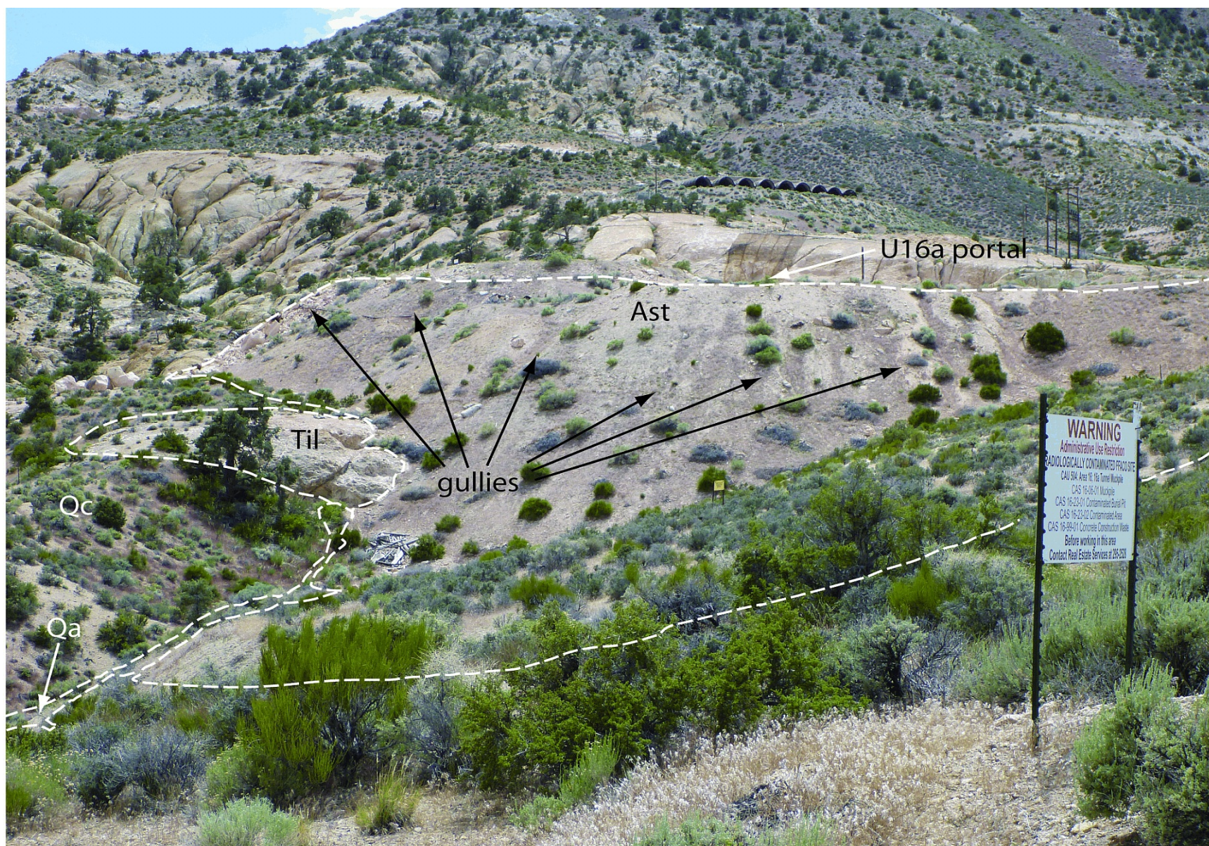
Figure 35. View west from the access road toward the U16a Tunnel portal. In the middle of the photograph the rilled and gullied tailings slope (Ast) is visible. Debris and tailings are visible in the stream along the base of the tailings slope.
