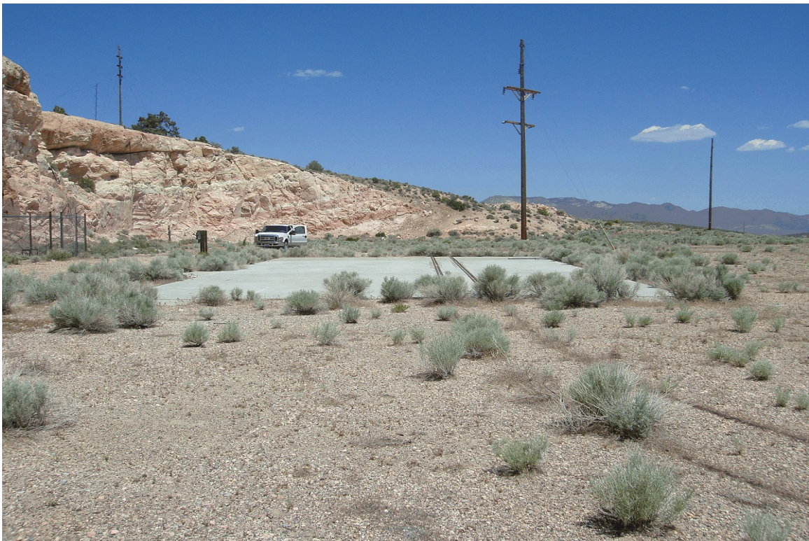
Figure 60. U16a Tunnel Feature 18, plan map and photograph of foundation for Assembly Building 16-101, view southeast (2011).
