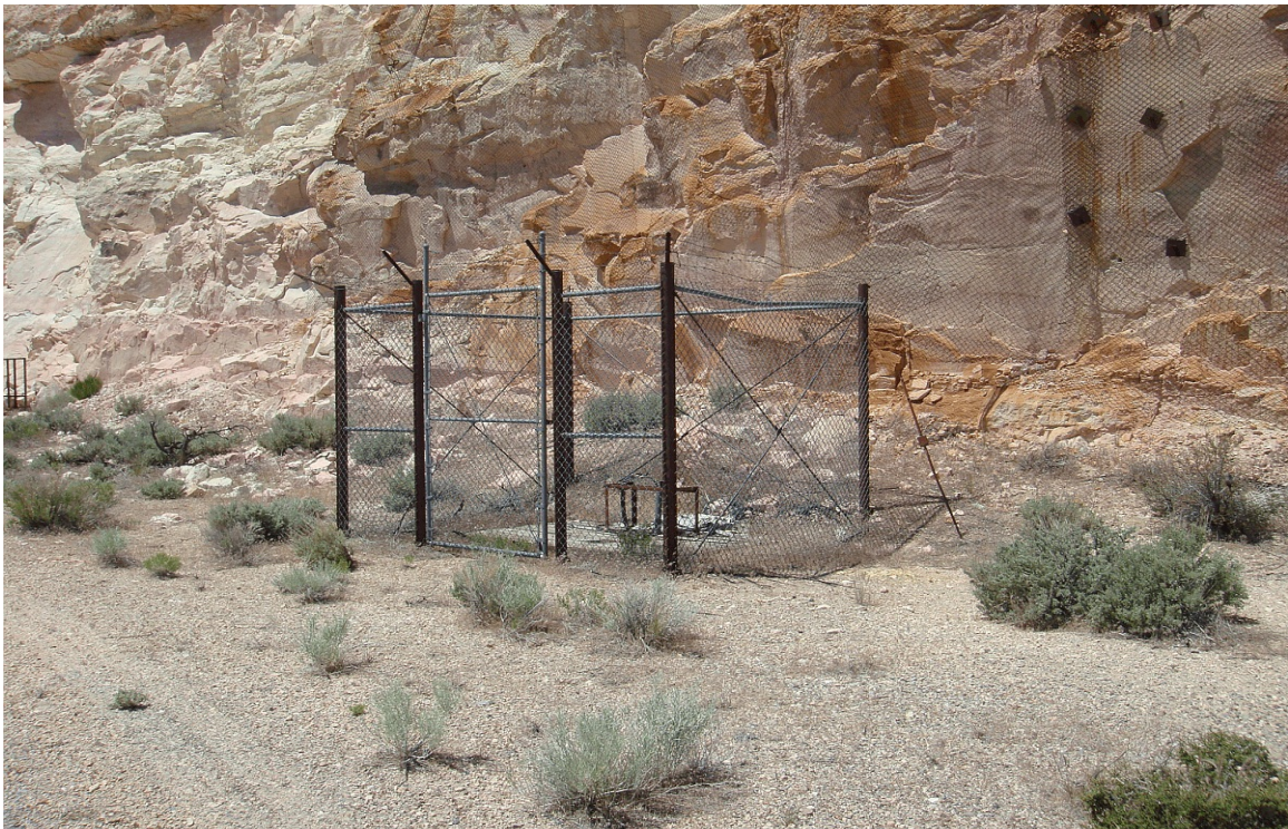
Figure 59. U16a Tunnel Feature 17, plan map and photograph of transformer station, view southwest (2011).
