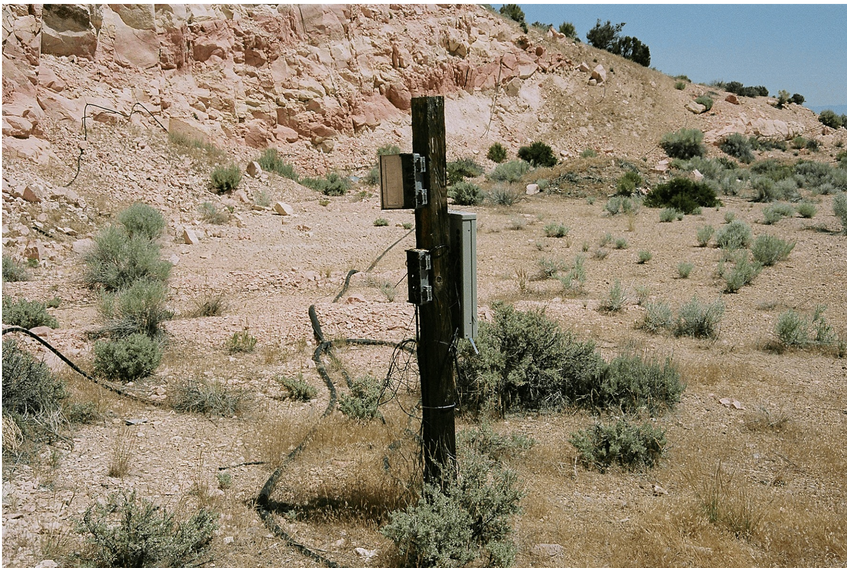
Figure 58. U16a Tunnel Feature 16, post and communications panel boxes, view north (2011).
