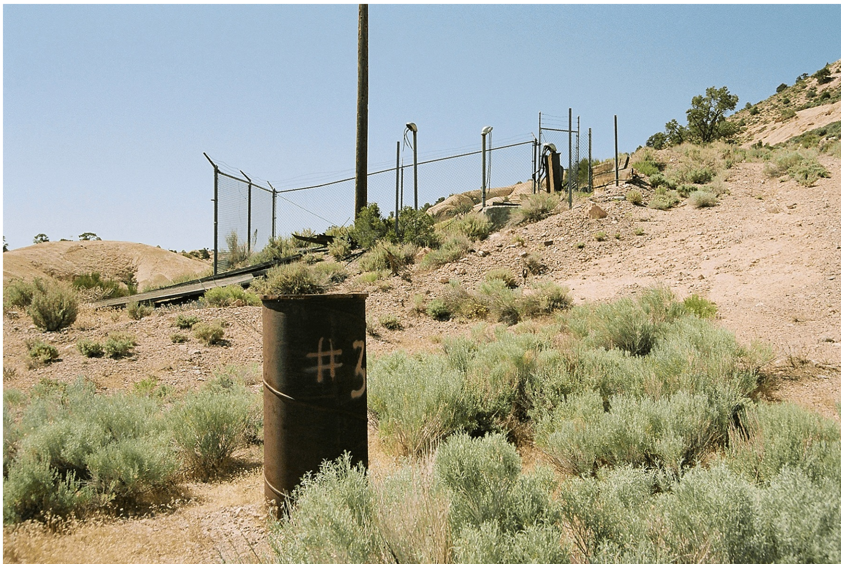
Figure 76. U16a Tunnel Feature 33, pipe, view south (2011).
