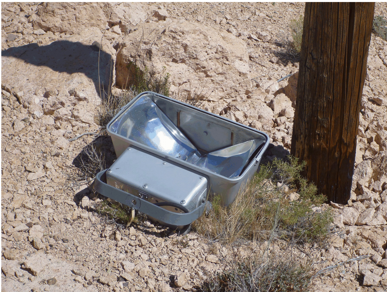
Figure 68. U16a Tunnel Feature 25, light, view northeast (2011).
