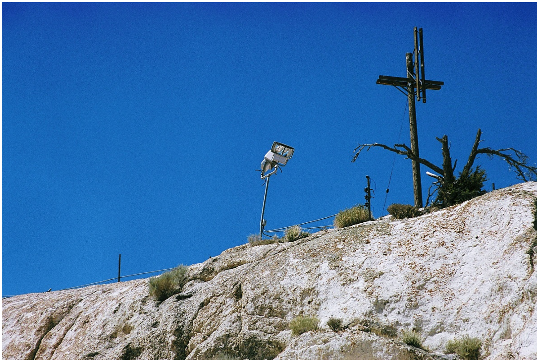
Figure 69. U16a Tunnel Feature 26, light fixture, view southwest (2011).
