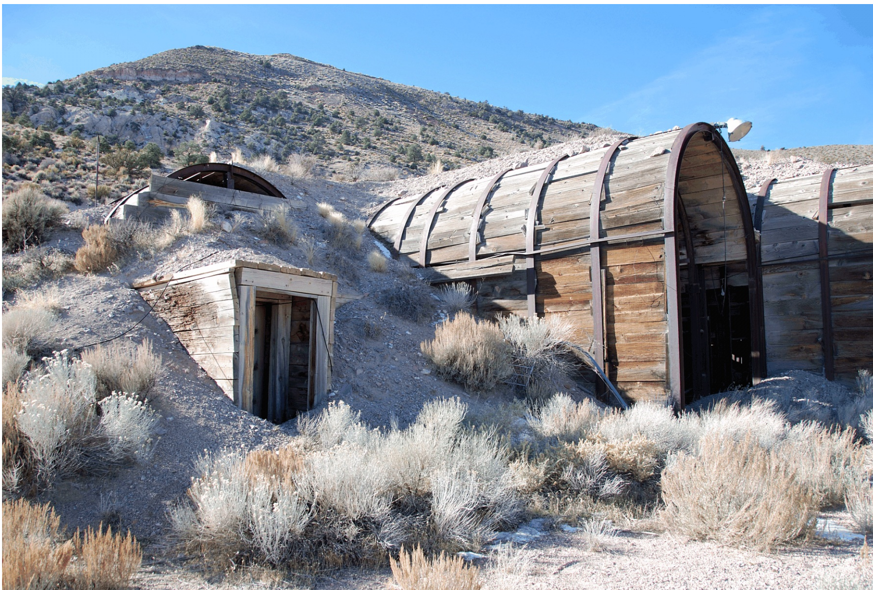
Figure 94. U16a Tunnel Feature 39 Structure 10, view northwest (2010).
