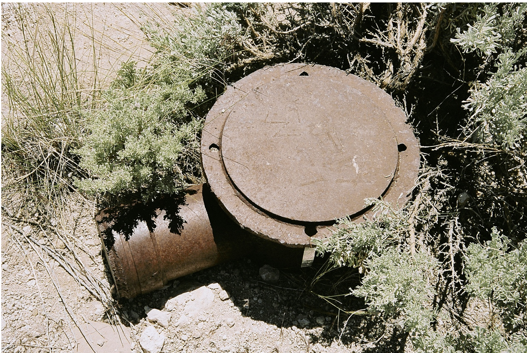
Figure 103. U16a Tunnel Feature 46, U16a PS #2 W/S drill hole, view southeast (2011).
