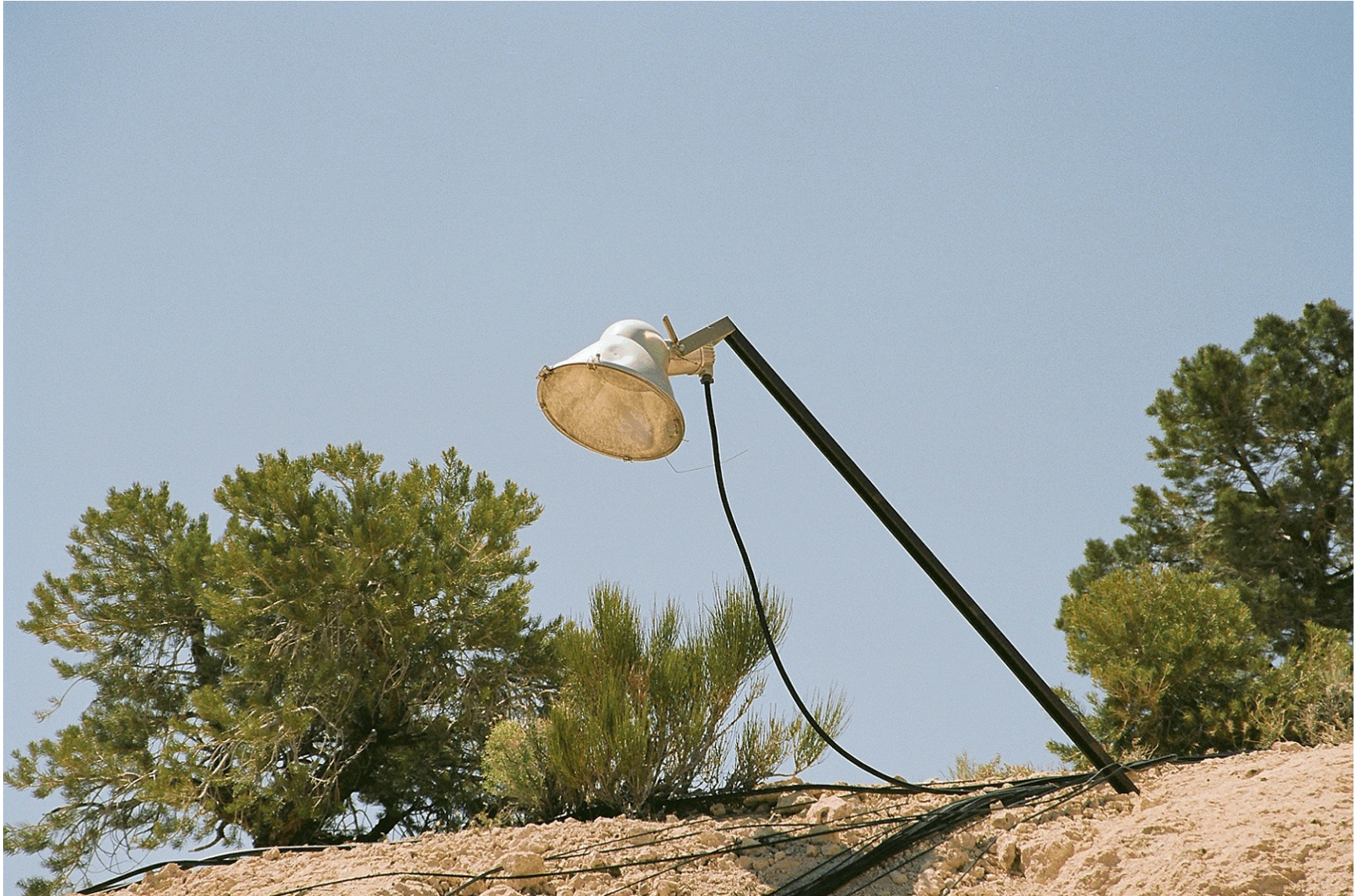
Figure 73. U16a Tunnel Feature 30, light fixture, view south (2011),
