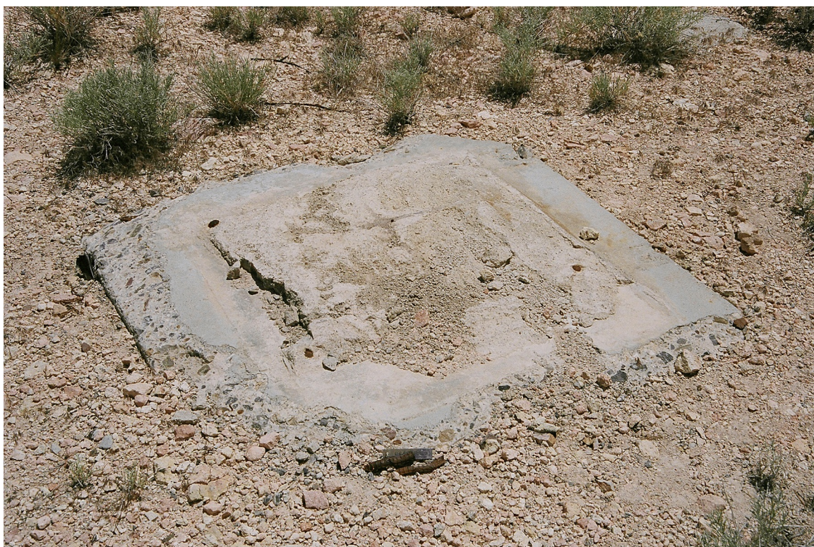
Figure 42. U16a Tunnel Feature 2, plan map and photograph of concrete pads, view northeast (2011).
