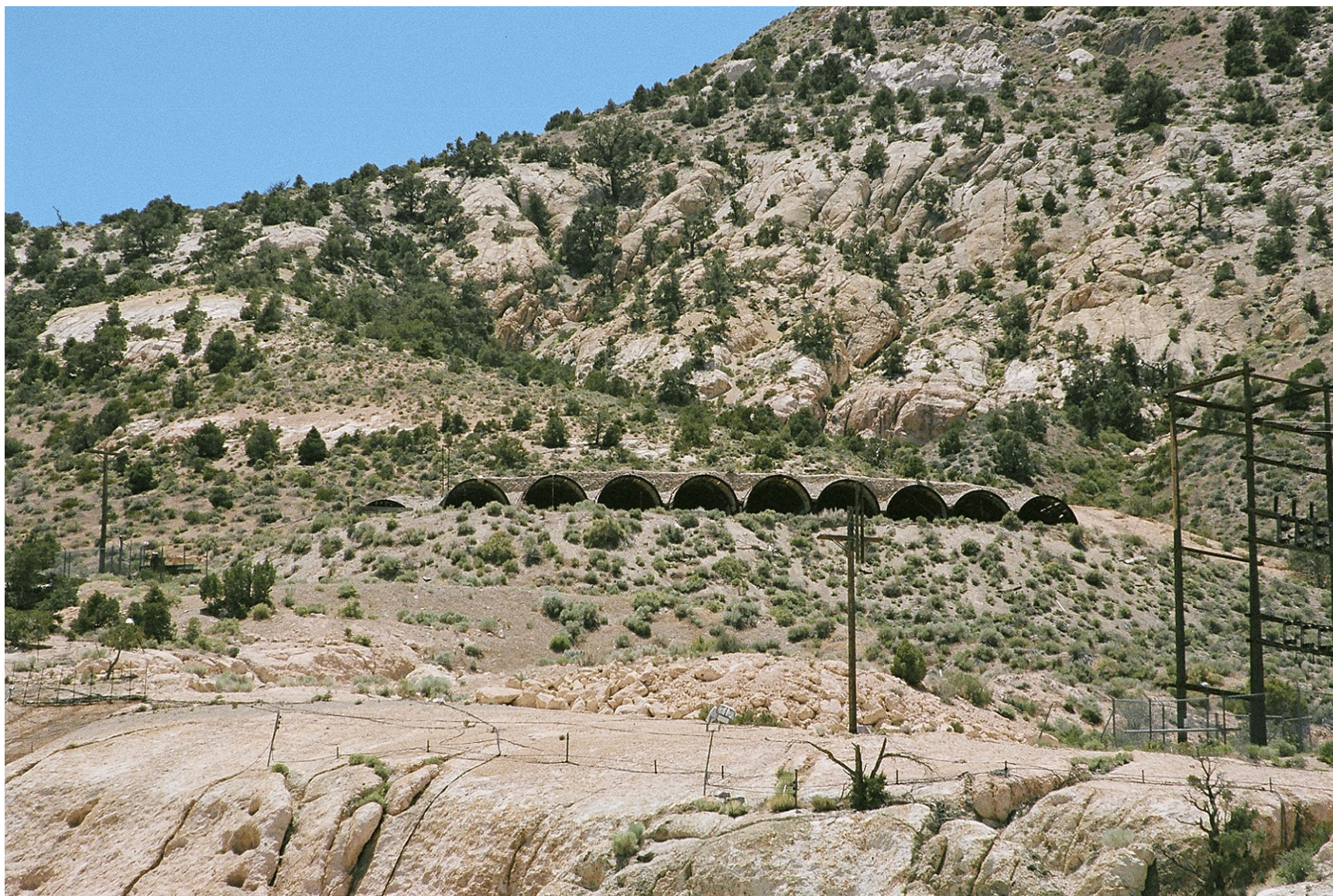
Figure 84. U16a Tunnel Feature 39, Fort Morgan, view southwest (2011).
