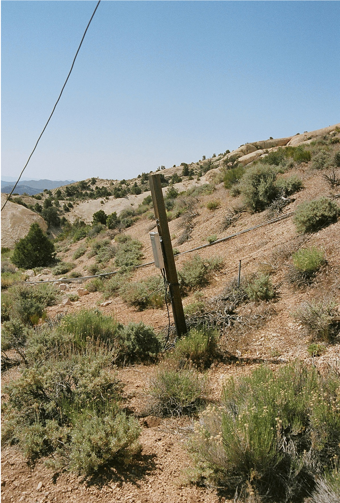
Figure 79. U-16a Tunnel Feature 36, post and communications panel, view south (2011).
