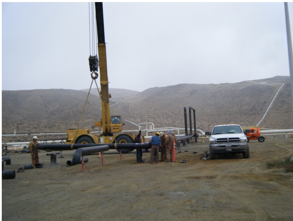
Figure 28 Installation of Brine Lines
