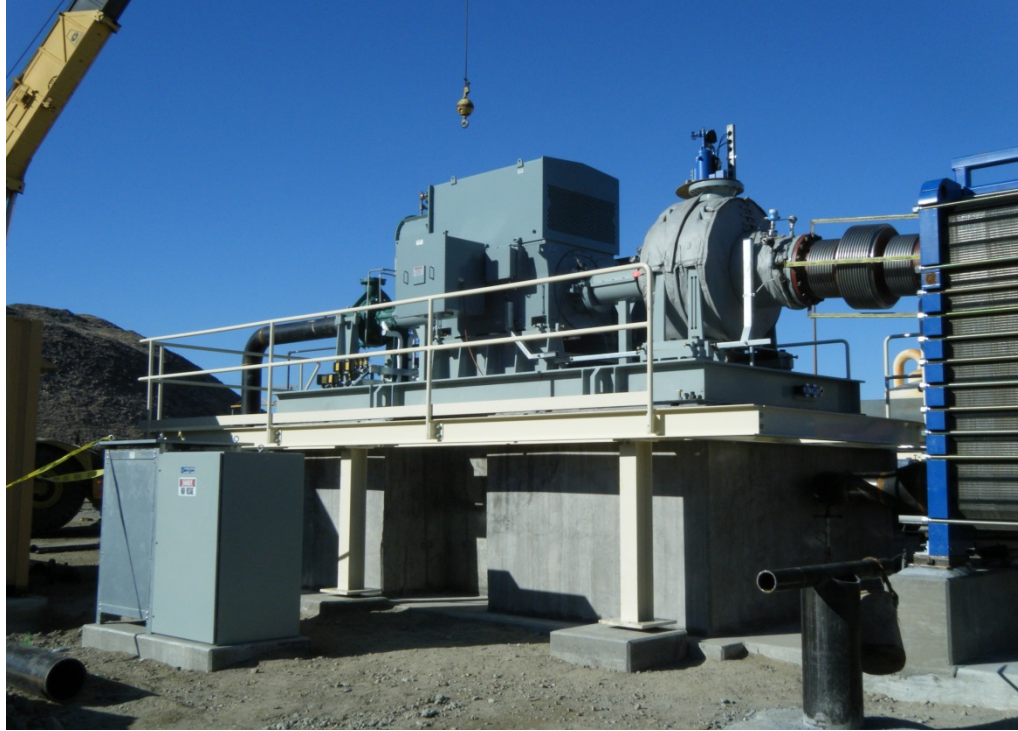
Figure 31 Turbine Pedestal
