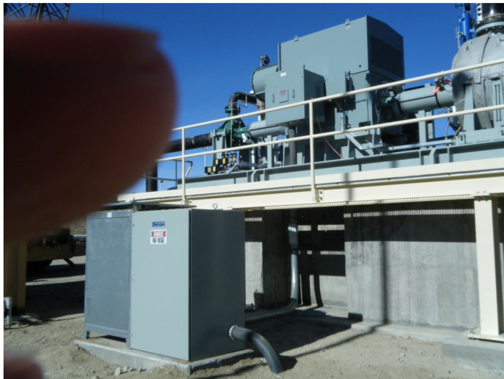
Figure 30 Completed Electrical Connection to Soft Starter
