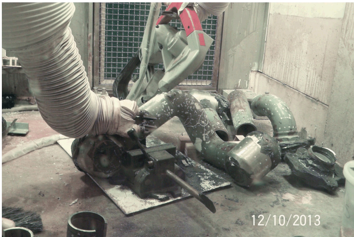
Figure 2-8. Photo of the Initial Cut on Jumper B – 2 Using a Portable Band Saw in a Hot Cell.
