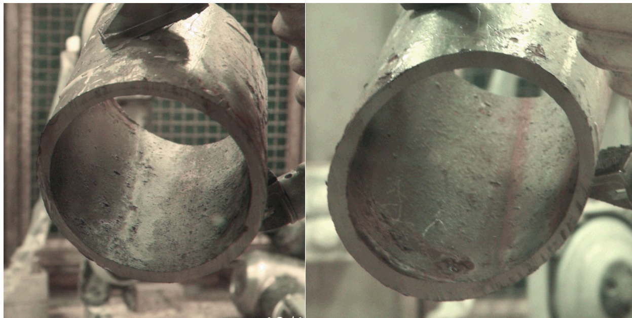
Figure 2-11. Photos of the Inner Surface of a Straight Section of Pipe from Jumper B – 2.
