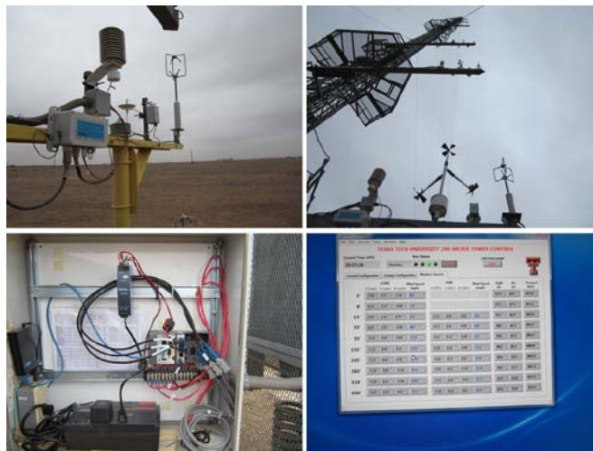
Figure 1.1.1. Collection of TTU 200 m tower hardware and software upgrades.
