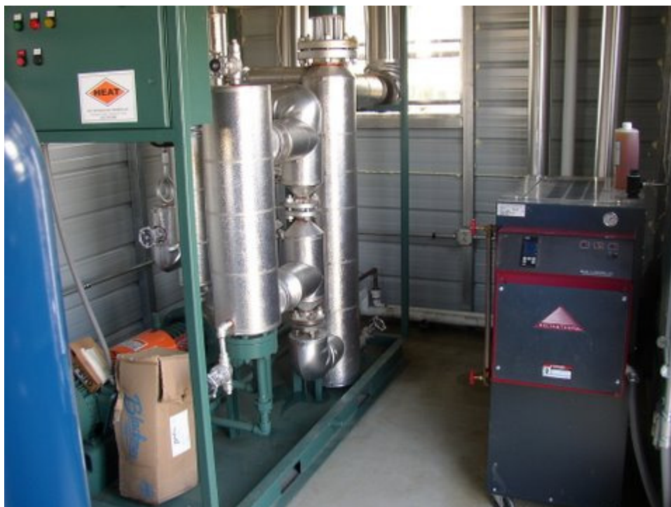
Figure 5.5: Hot oil unit and Delta T condenser control unit.
