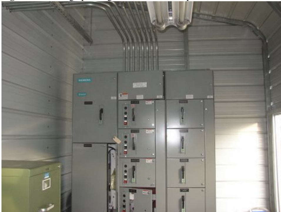
Figure 5.4: Motor control center.
