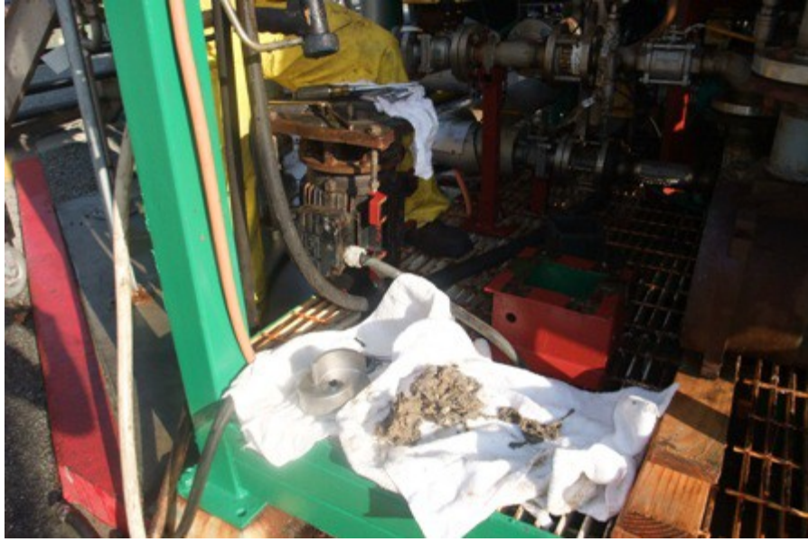
Figure 5: Material Removed During Rebuilding of Transfer Pump
