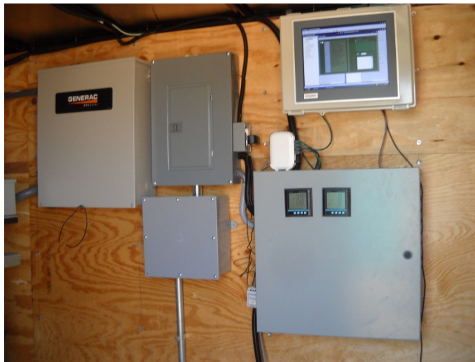
Figure 10. PLC Controller and LabView™ Computer
