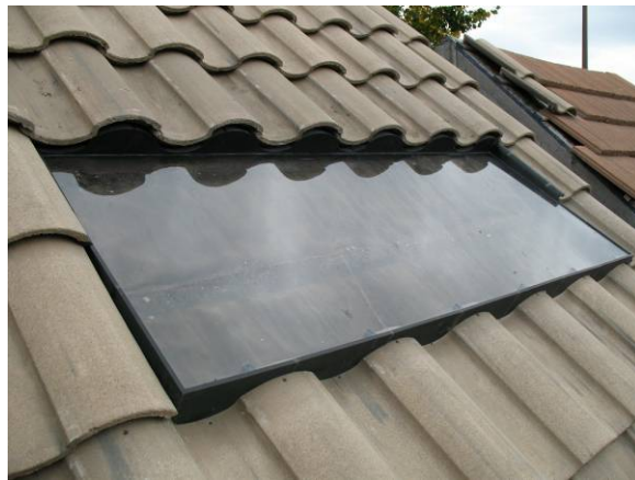
Figure 5.41: Test Installation of Rapid Prototype Module on Small Roof
