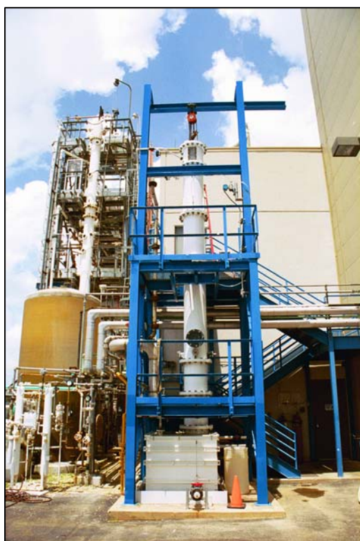
Figure 1a/b. Photograph and Schematic of the SRP Air/Water Contacting Device
