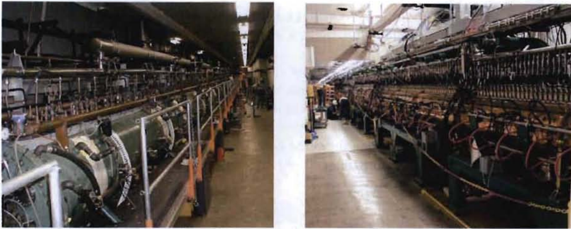
Fig. 4. Photograph of (a) the LANSCE-DTL water-cooling systems and (b) similar SNS-DTL systems.
