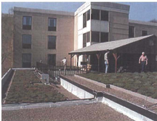
Figure 18: Accessible green roof combined with inverted ballasted roof in Tyrone, Pennsylvania (Extensive Green Roofs)
