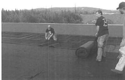
Figure 4: Installation of protective layer in Fairbanks, Alaska (CCHRC)
