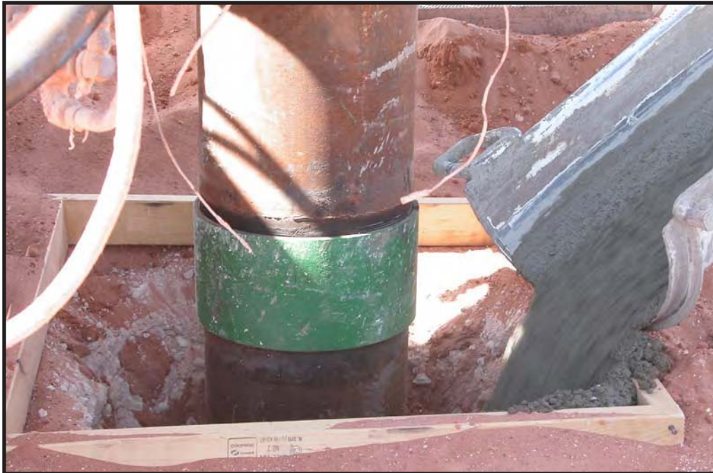
Above: Conductor casing being cemented in place at SNL-18 on June 19, 2006. The top of the green connector is the reference point for logging.
