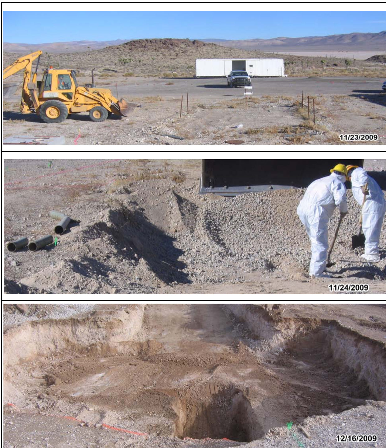
Figure D.1-8 CAS 06-05-04: Before, during, and after Removal of Leach Bed Materials
