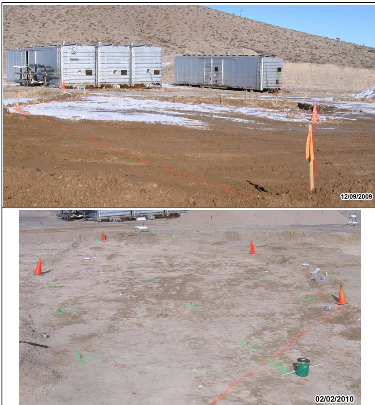
Figure D.1-10 CAS 06-05-04: Top: Larger TSCA-Level Soil Area before Removal; Bottom: Larger TSCA-Level Soil Area after Removal of 2.5-ft Soil Lift with Verification Sample Grids Plotted
