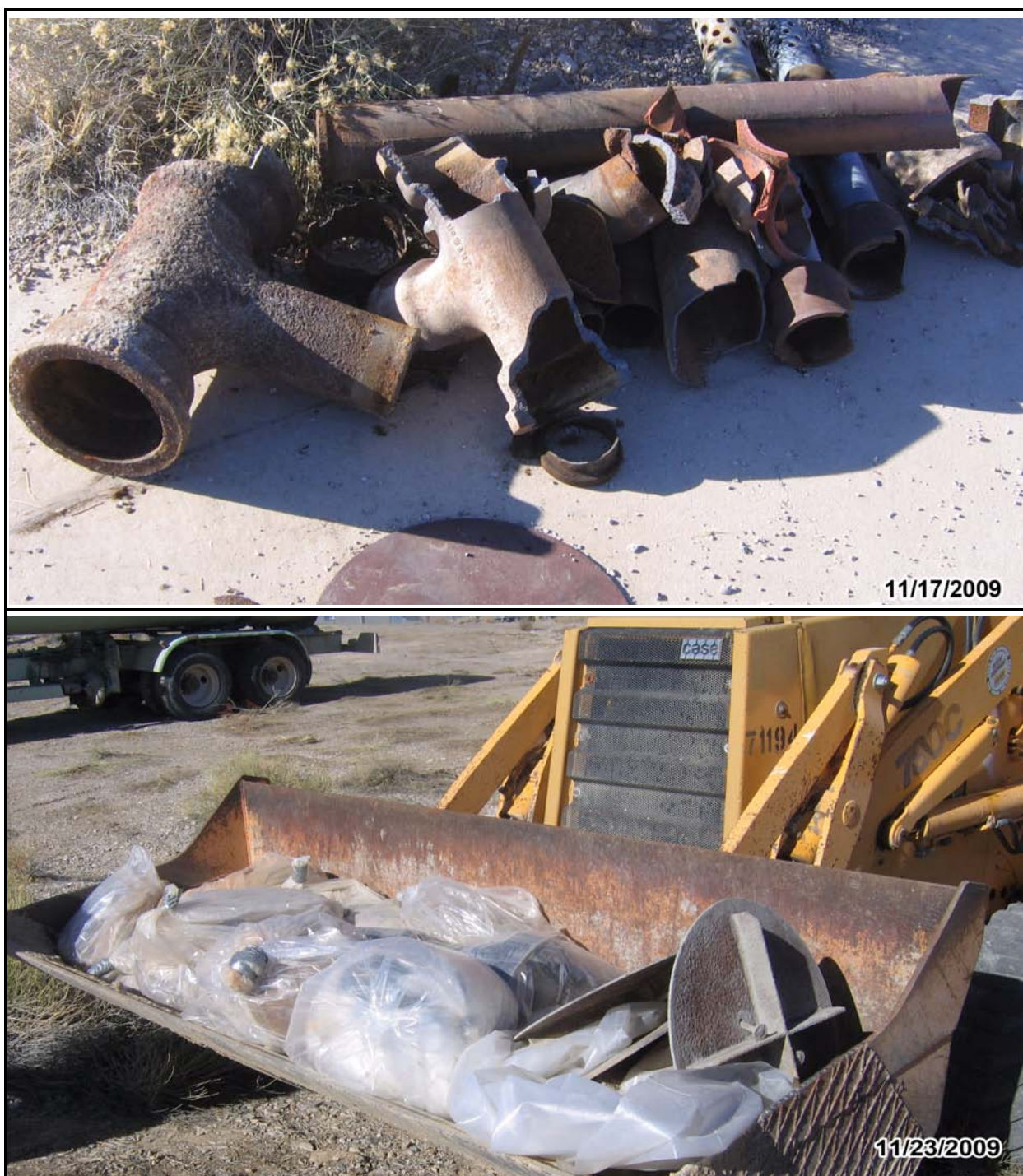
Figure D.1-17 CAS 06-59-05: Top: Piping Debris Staged for Disposal after the Lead-Containing Joint Seals Were Separated; Bottom: Septic Tank Sludge and Metal Lids Being Loaded for Disposal
