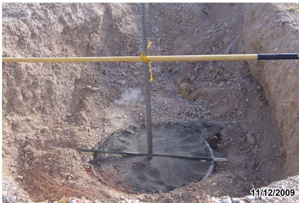
Figure D.1-6 CAS 06-05-03: Grouting of Leach Pit Chamber and Emplacement of UR Post
