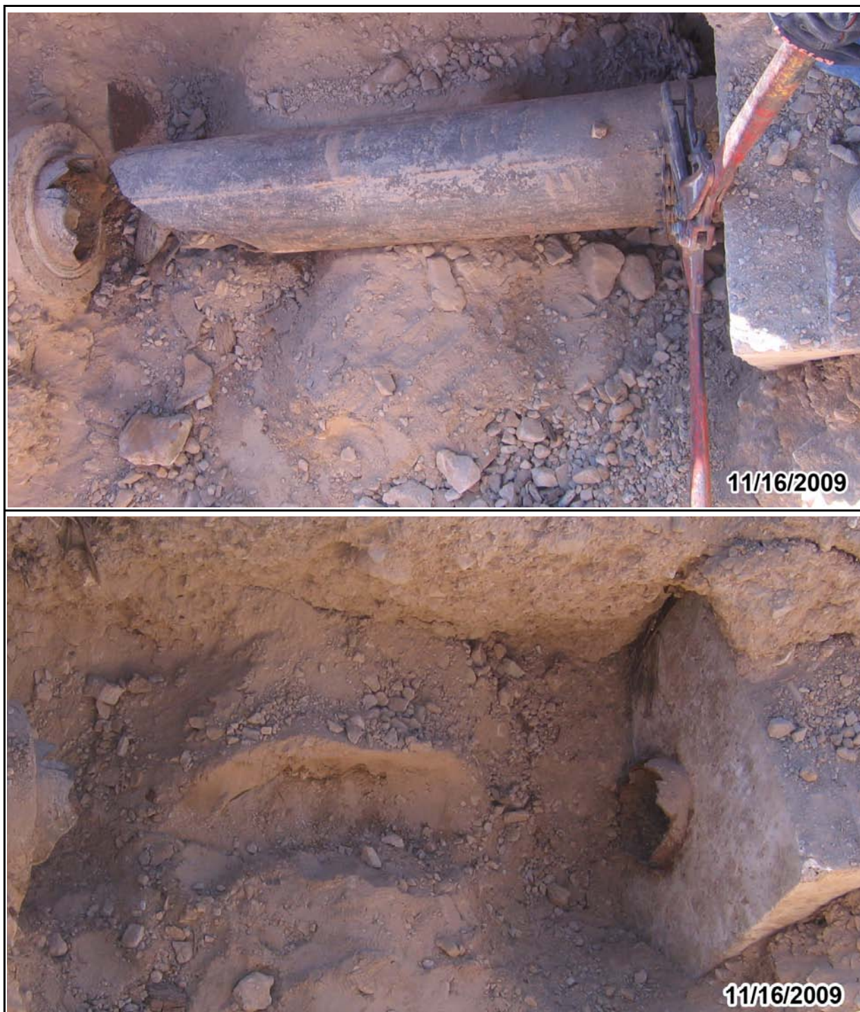
Figure D.1-16 CAS 06-59-05: Removal of the Inlet End Piping and PSM
