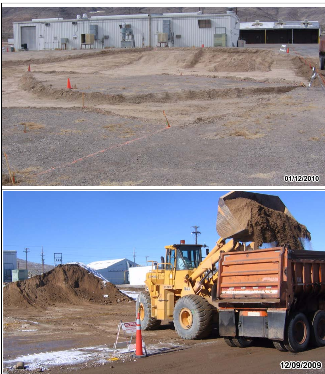
Figure D.1-9 CAS 06-05-04: Top: Post-Removal View of Non-TSCA Soil Area; Bottom: Non-TSCA Soil Waste Loading for Disposal
