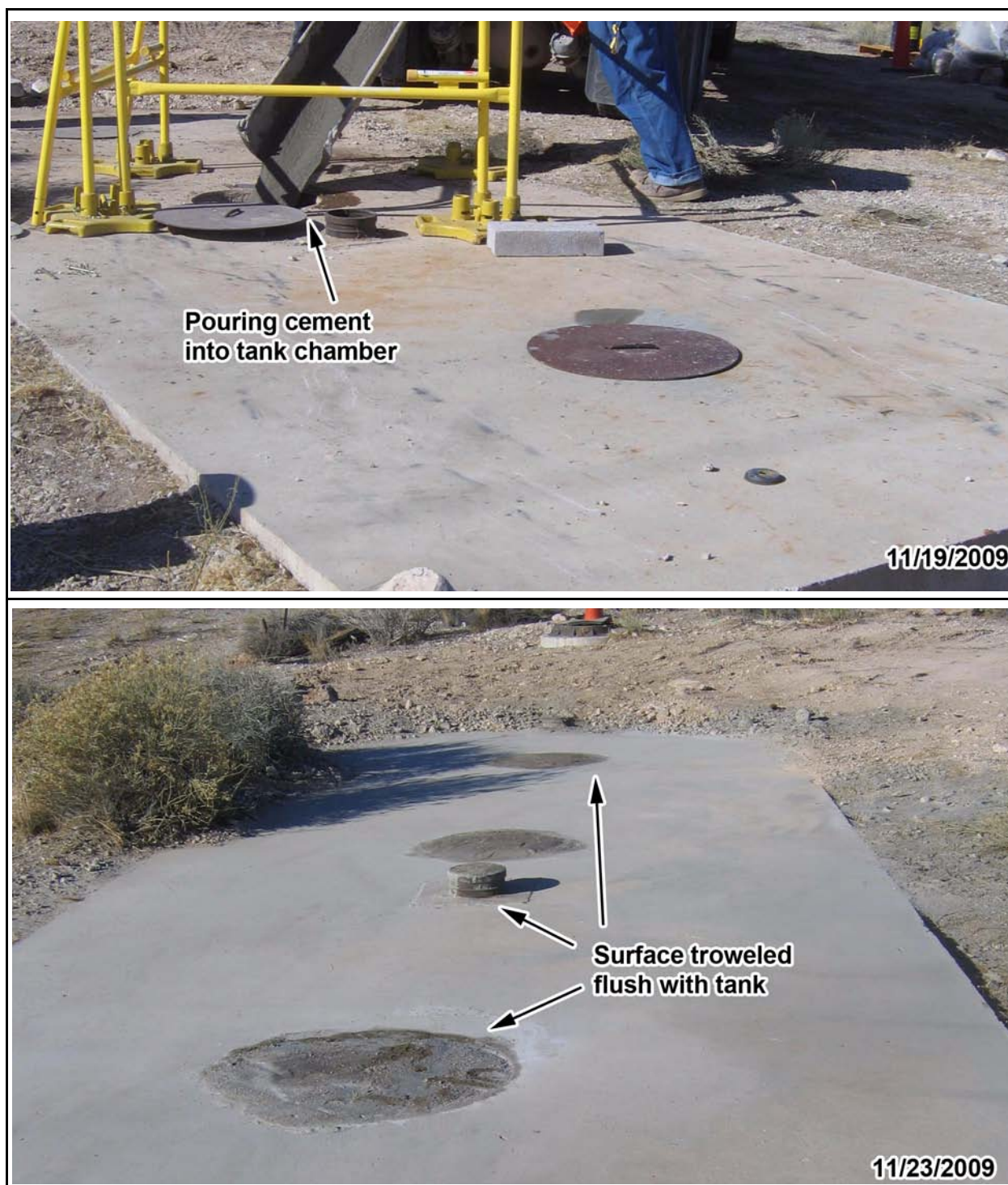
Figure D.1-19 CAS 06-59-05: Septic Tank during and after Grouting
