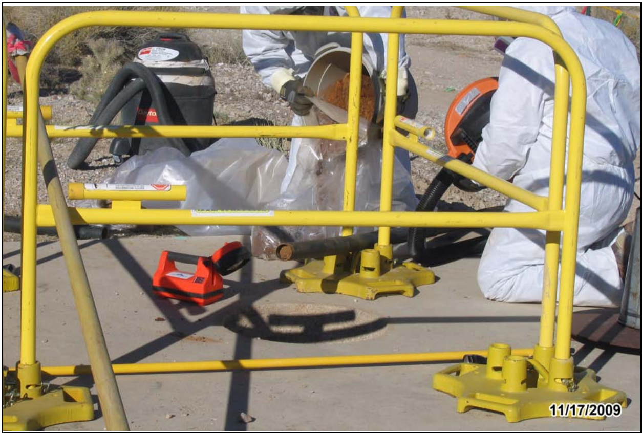
Figure D.1-18 CAS 06-59-05: Removal of COC-Impacted Sludge from the Septic Tank
