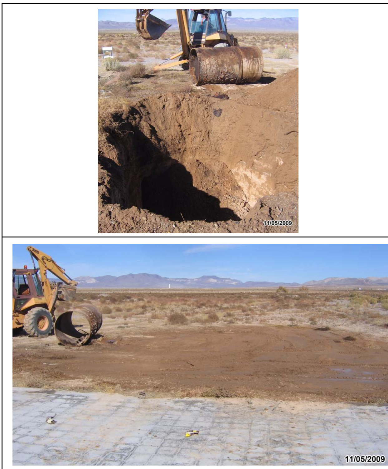
Figure D.1-1 CAS 03-51-01: BMP Activities during and after Leach Pit Casing Removal
