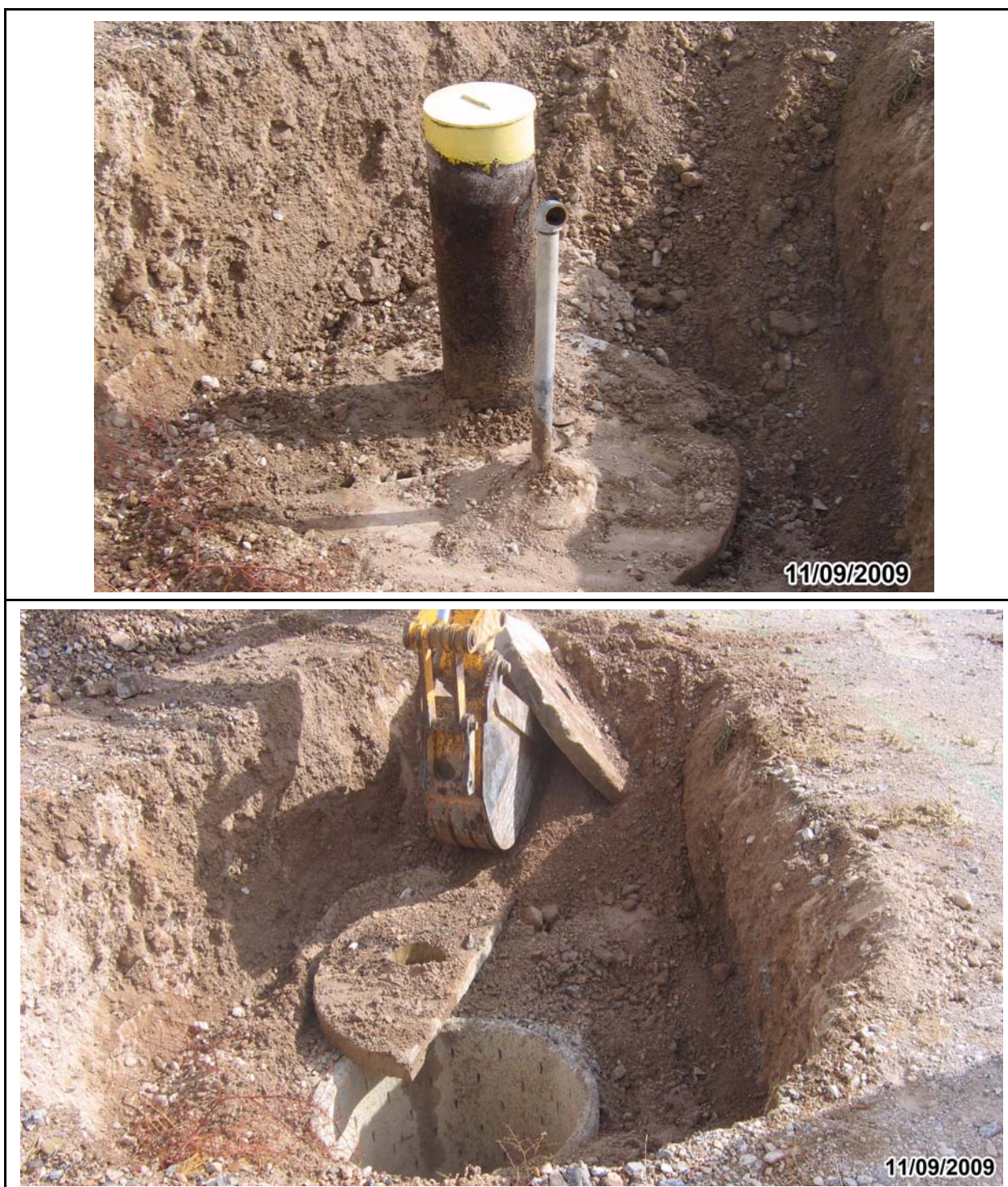
Figure D.1-5 CAS 06-05-03: Accessing and Removing Leach Pit Chamber Lid and Riser Pipes
