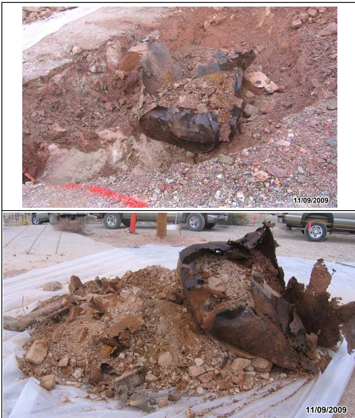
Figure D.1-12 CAS 06-59-03: Excavation of Septic Tank in Process and Stockpiled Soil, PSM, and Tank Debris before Disposal
