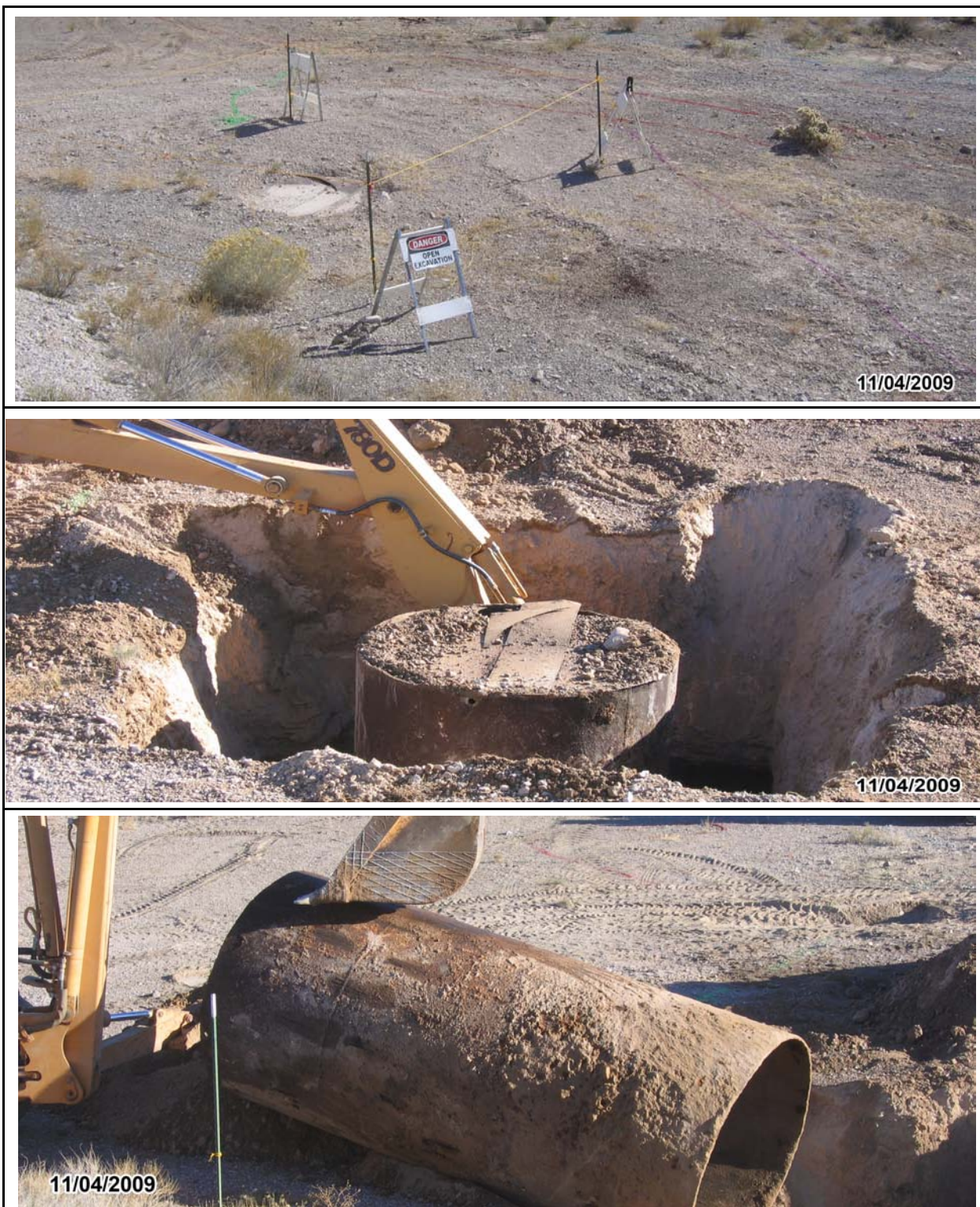
Figure D.1-2 CAS 06-04-02: BMP Activities before, during, and after Leach Pit Casing Removal
