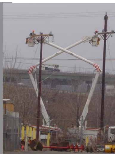
Tie-in to Line 27 and Pulling Overhead Conductor
