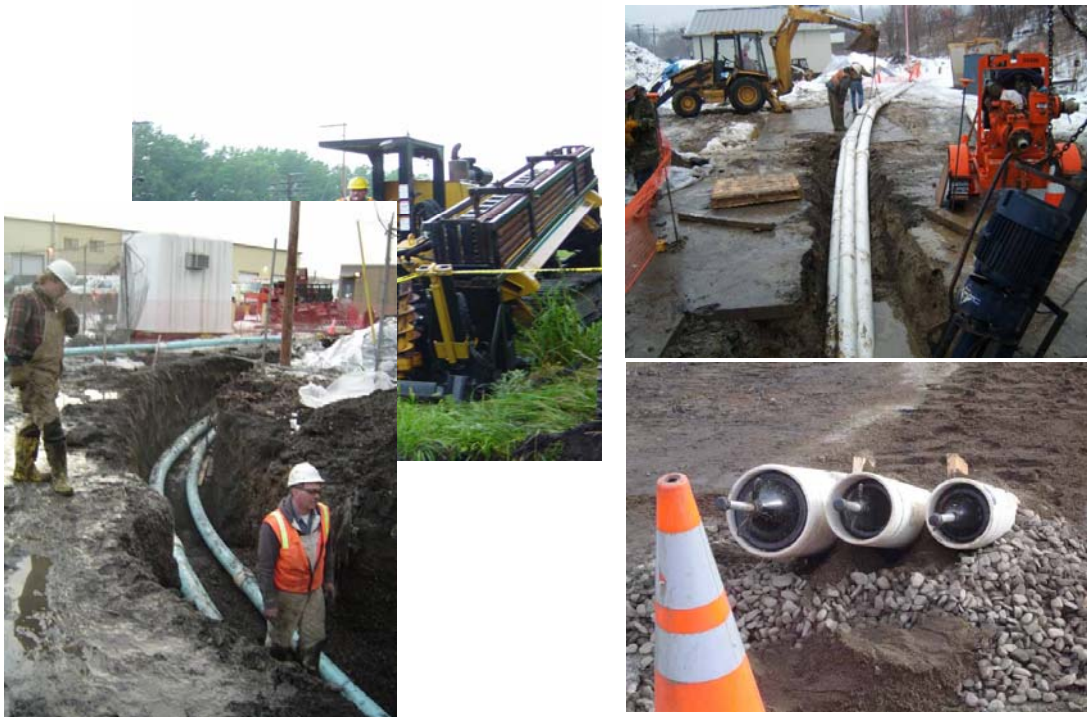
Figure 6 Conduit Installation.
