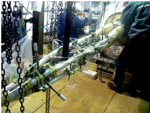
Spread three cable cores.
