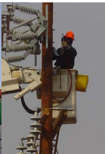
Installation of Disconnect Switches
