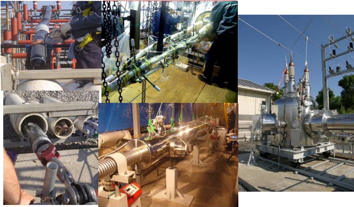
Figure 32 BSCCO Cable, Terminations and Joint Installation.
