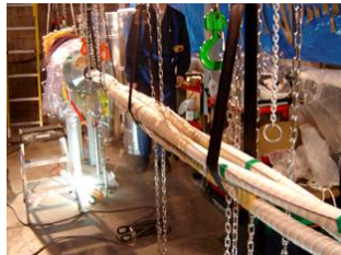
3 Cable cores after connecting
