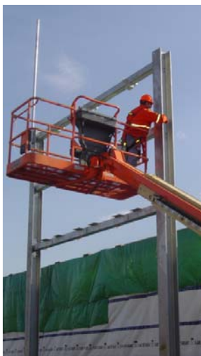
Take-Off Structure Installation
