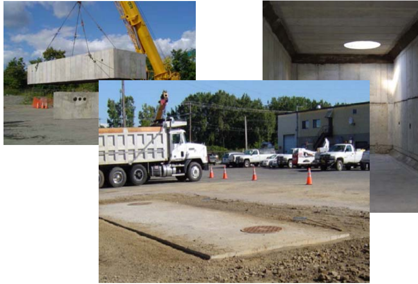
Figure 7 Underground Vault Installation for Cable-to-Cable Joint.
