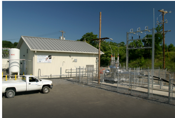
Figure 8 Cryogenic Refrigeration System Building, LN 2 Storage Tank and South Termination.
