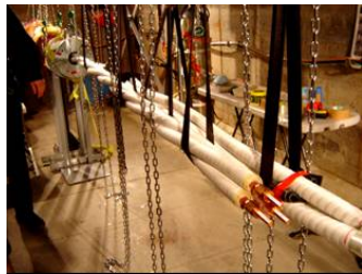
3 Cable cores before connecting
