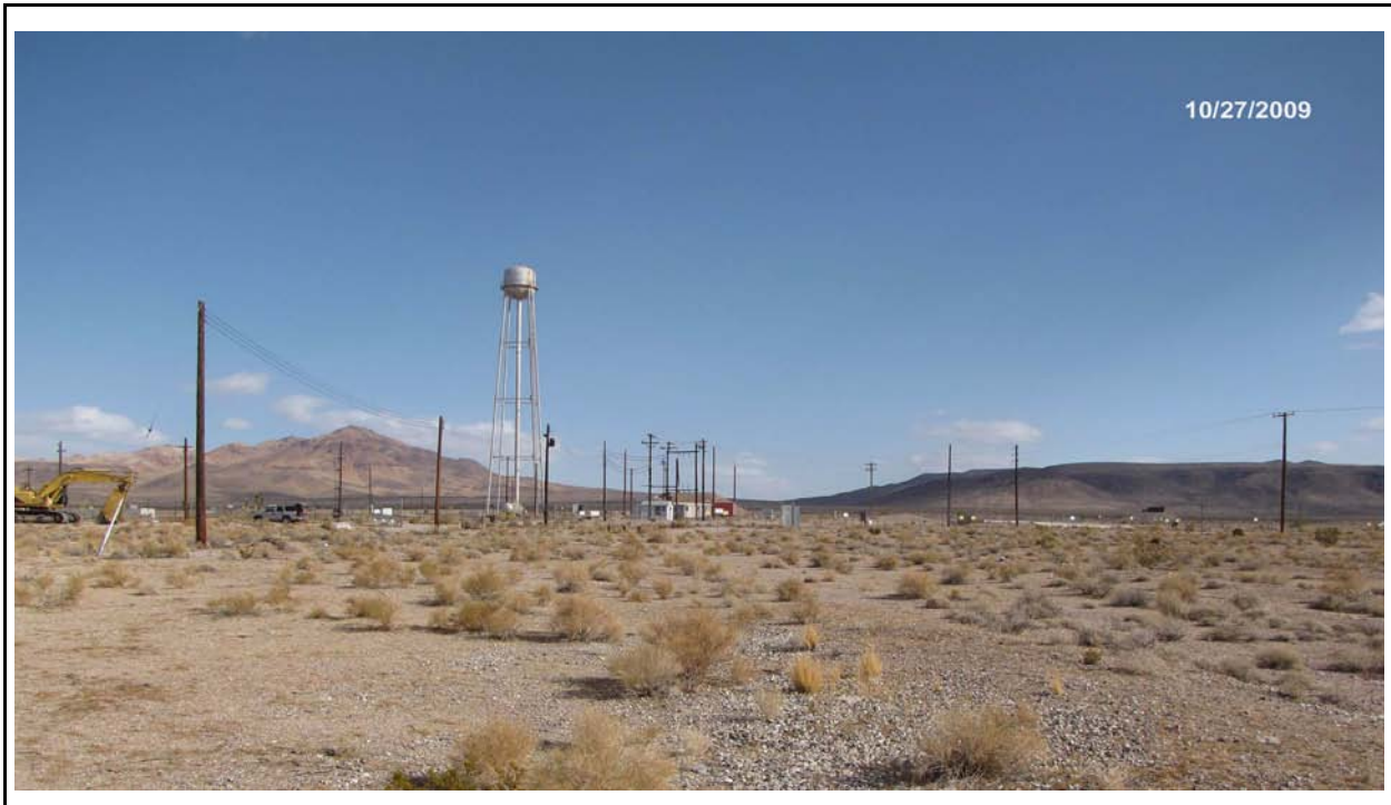
Figure 2-1 Test Cell A Area - Current Ground View
