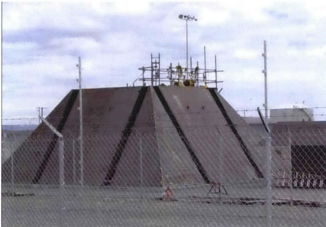
Outside Storage Unit for Slightly Irradiated Fuel
