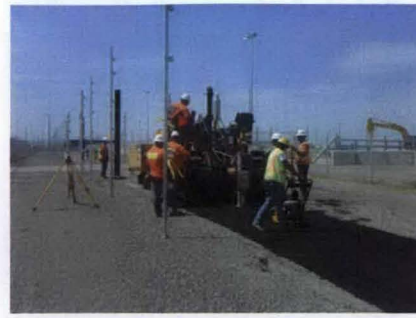
Intrusion Detection System Paving
