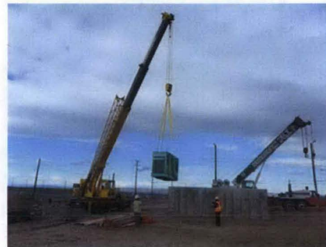
Auxiliary Generator Placement
