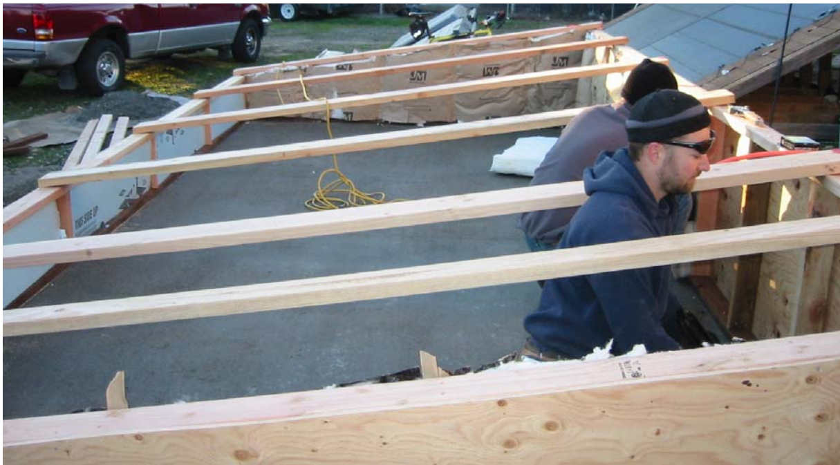
Figure 21: Framing of Above Grade Insulated Walls
