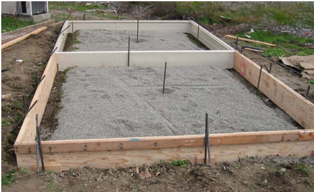
Figure 18: Formed Slab Prior to Pour
