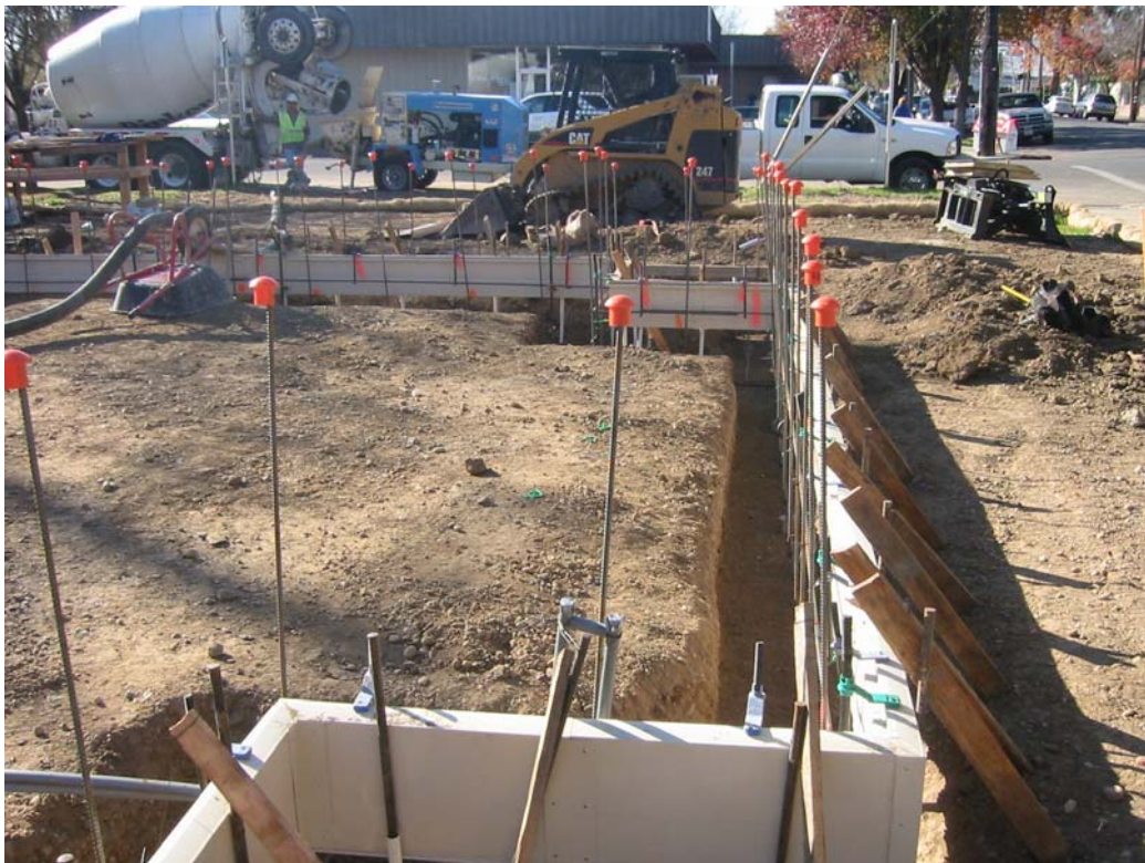
Figure 27: Staked Formulate Prior to Pour
