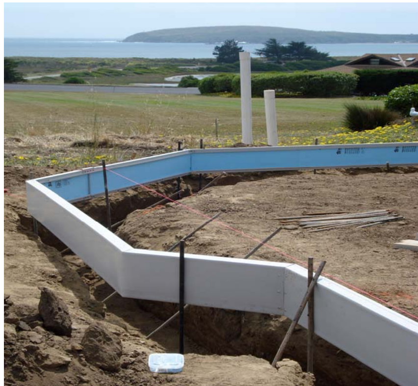
Figure 30: Perimeter with 45° and 135° Angled Formboards
