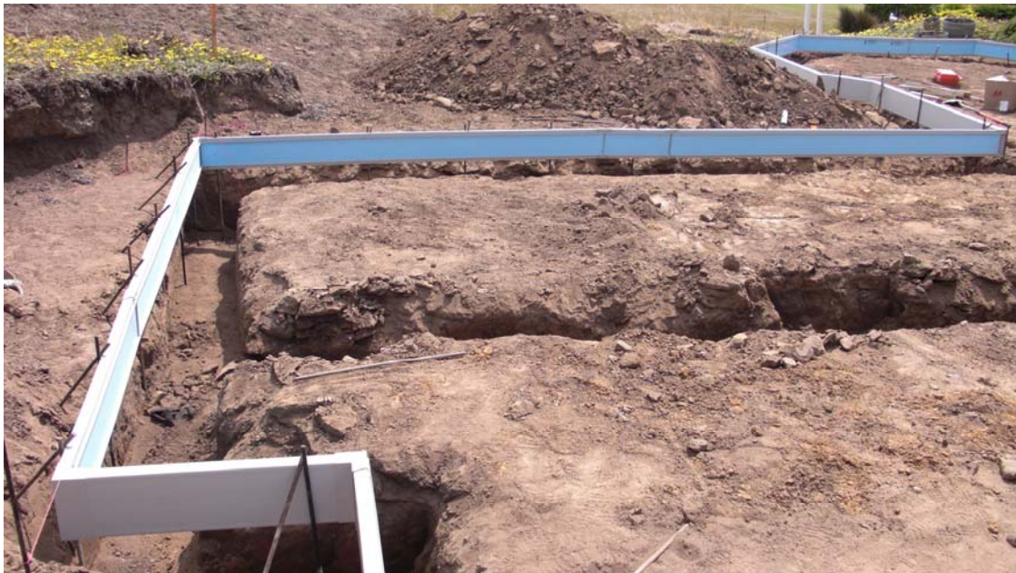
Figure 32: Completed Formboard Installation
