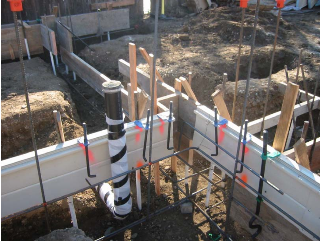
Figure 28: J-Bolt and Rebar Installation Details
