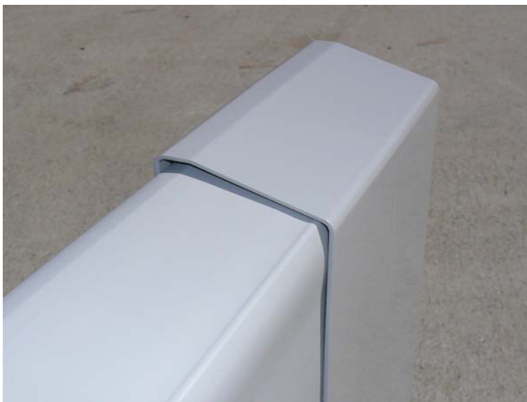
Figure 12: Excessive Gap at Extrusion/Coupler Interface
