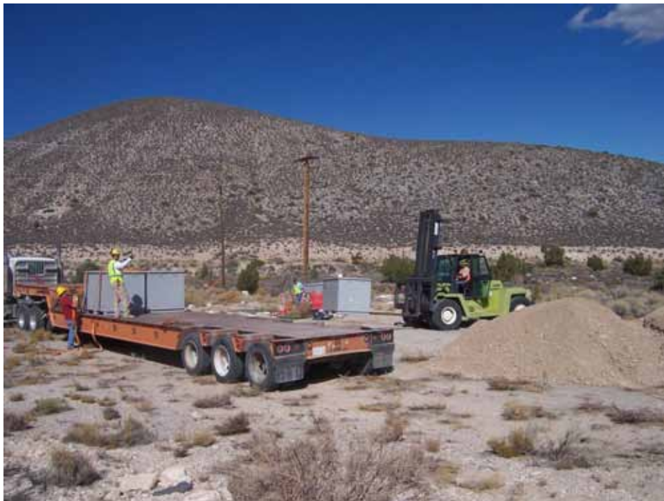
Photograph 24: CAS 12-59-01, Loading Chlordane-Impacted Soil for Disposal, 10/15/2009
