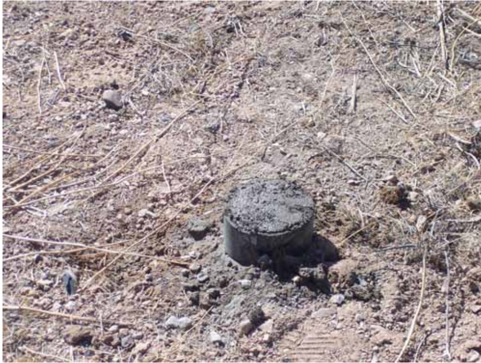
Photograph 13: CAS 03-59-05, Grouted Pipe Opening, 09/21/2009
