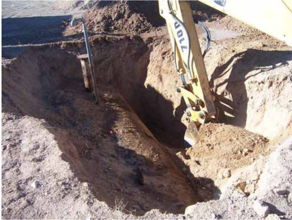
Photograph 17: CAS 03-04-02, Excavation of Septic Tank, 09/22/2009
