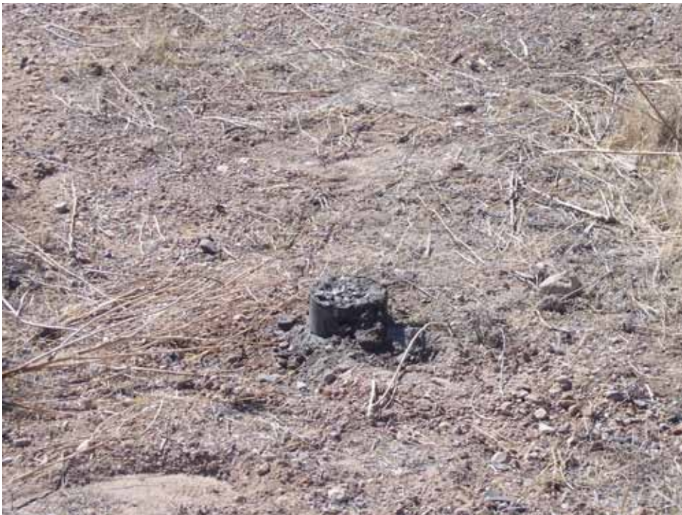
Photograph 12: CAS 03-04-02, Grouted Pipe Opening, 09/21/2009
