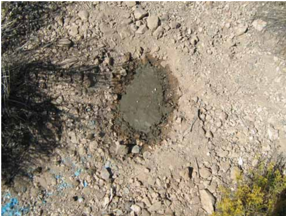
Photograph 6: CAS 12-59-01, Grouted Riser Pipe Openings, 09/17/2009
