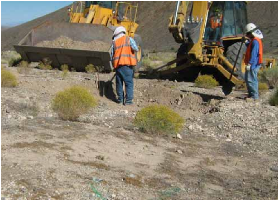
Photograph 2: CAS 12-59-01, Excavation of Arsenic- and Chromium-Impacted Soil, 09/16/2009
