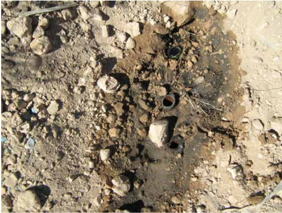
Photograph 5: CAS 12-59-01, Riser Pipes Cut At Grade, 09/17/2009
