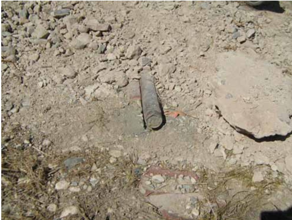
Photograph 9: CAS 12-60-01, Grouted Drain Pipe Opening, 09/17/2009
