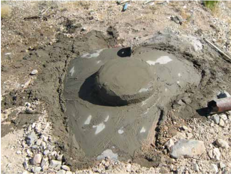
Photograph 21: CAS 12-59-01, Grouted South Tank, 09/24/2009
