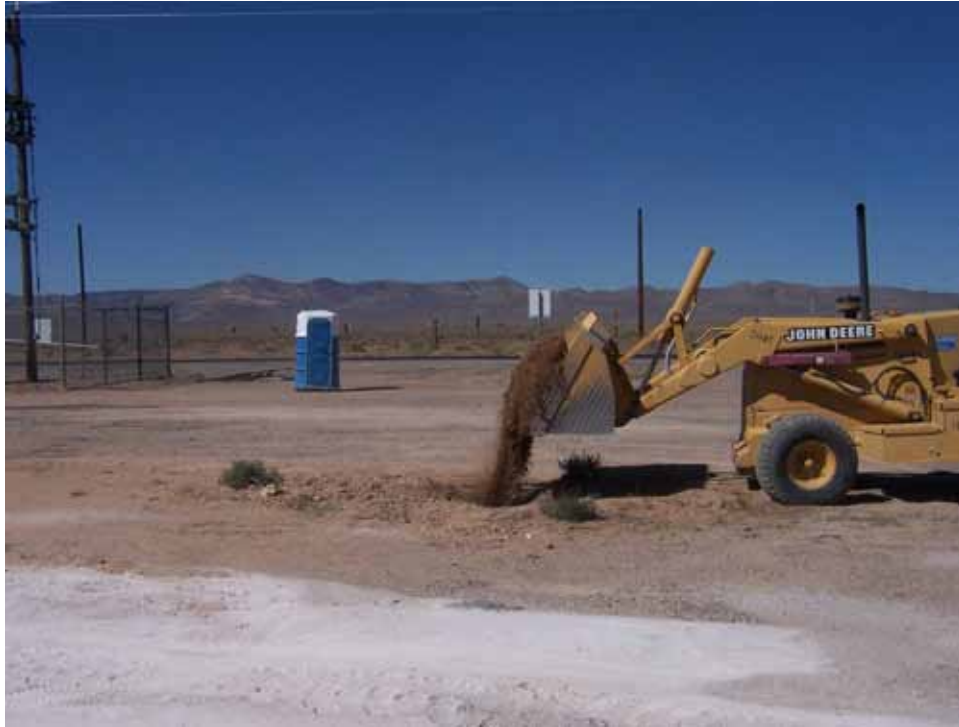
Photograph 15: CAS 03-59-05, Filling Cesspool with Soil, 09/21/2009
