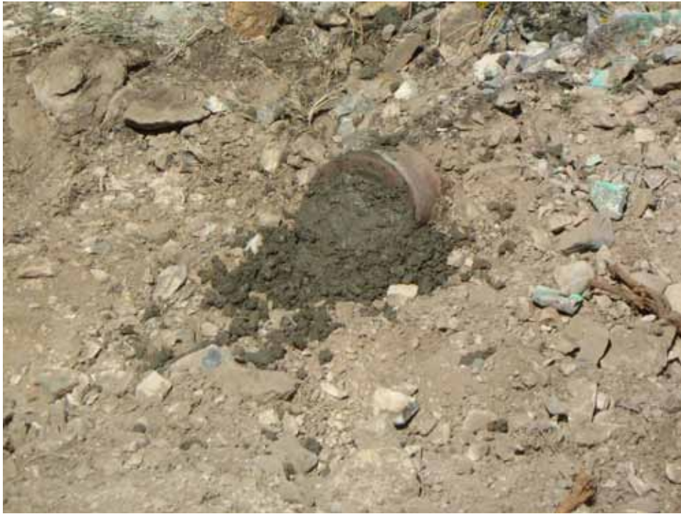
Photograph 3: CAS 12-59-01, Grouted Outfall Pipe, 09/16/2009
