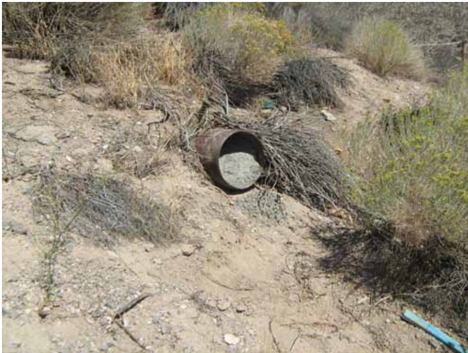
Photograph 8: CAS 12-60-01, Grouted Drain Pipe Opening, 09/17/2009
