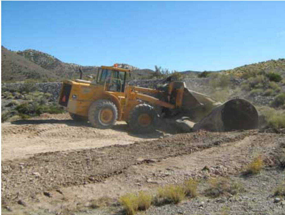
Photograph 11: CAS 12-59-01, Size Reduction of North Tank, 09/17/2009
