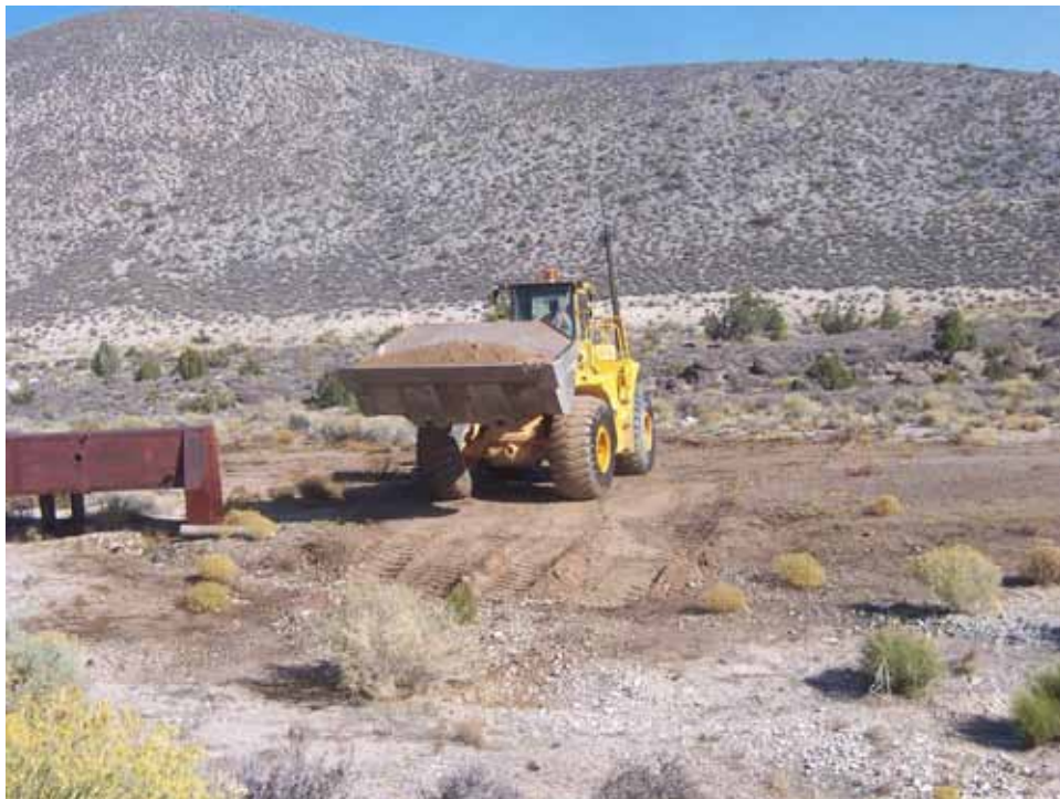
Photograph 26: CAS 12-59-01, Backfilled Arsenic- and Chromium-Impacted Soil Excavation, 10/19/2009
