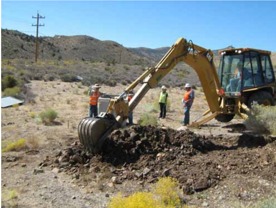
Photograph 1: CAS 12-59-01, Excavation of Chlordane-Impacted Soil, 09/15/2009
