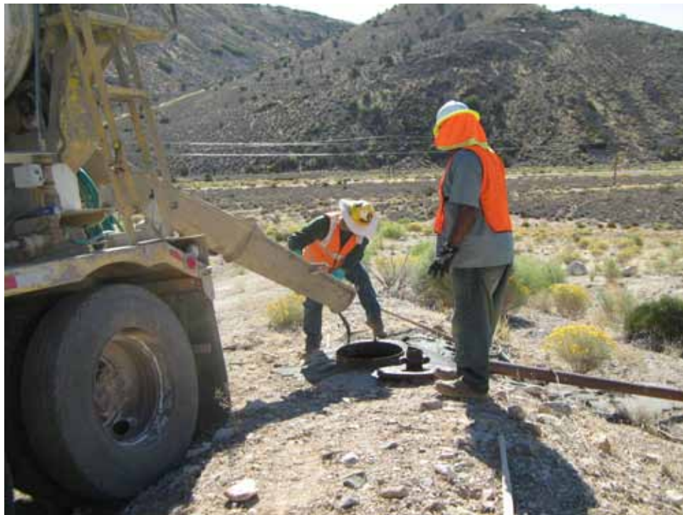
Photograph 20: CAS 12-59-01, Grouting South Tank, 09/24/2009
