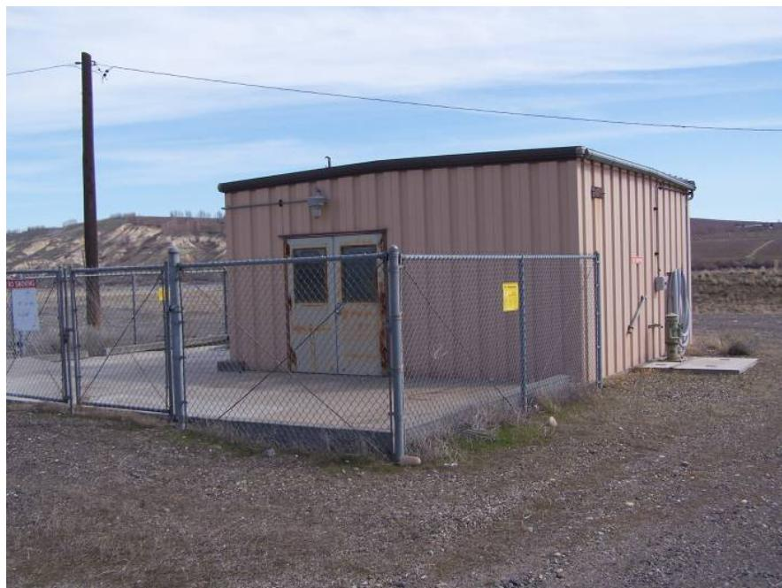
The 332 Building was a pre-engineered metal building on a 15.24 cm (6 in.) slab with footings. The building was 6.10 m (20 ft) by 6.10 m (20 ft) by 3.05 m (10 ft) in eve height. On the north and west sides of the building was a 0.15 m (0.5 ft) thick slab with spill curbing.
