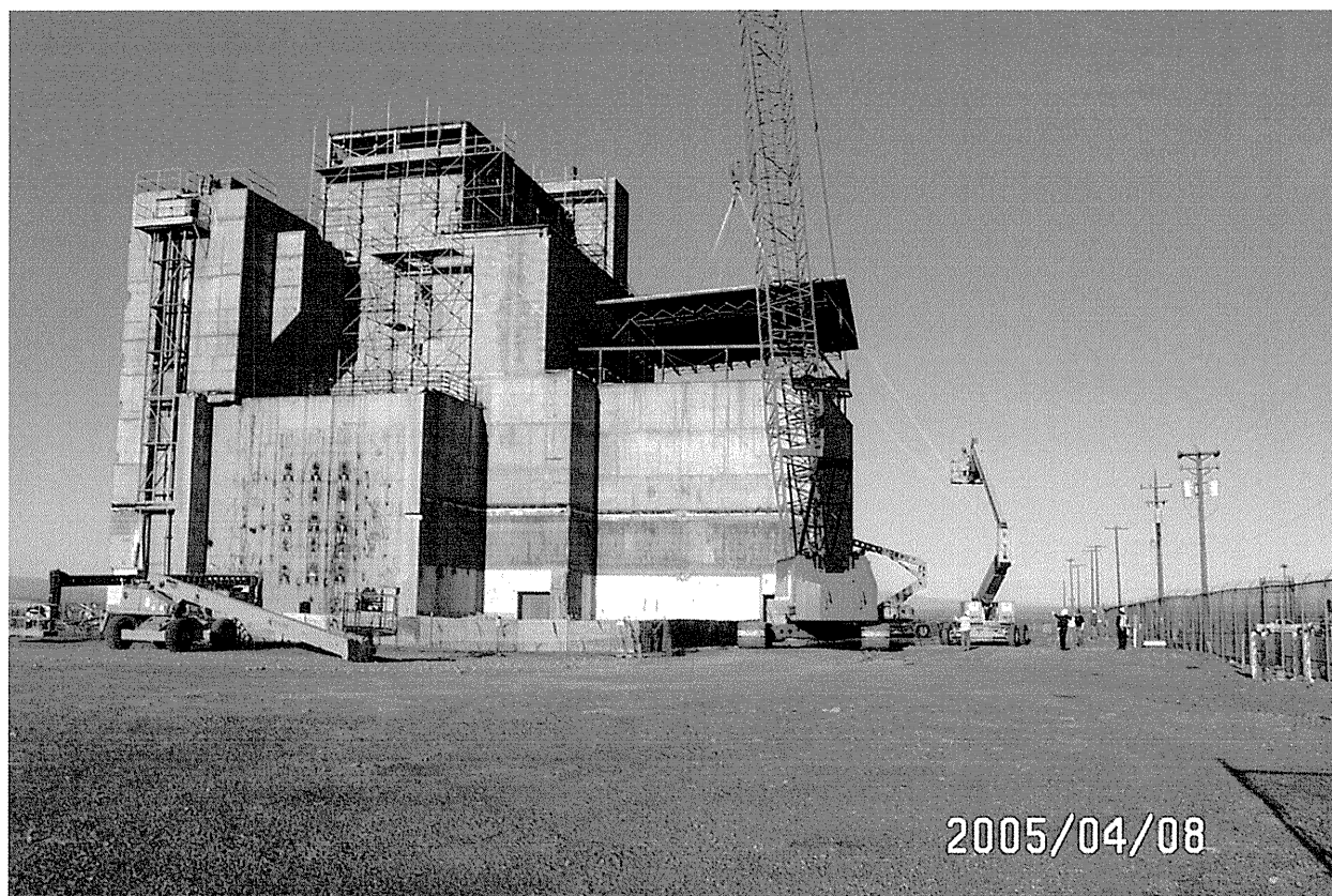
Figure 4-2. Photograph Showing Upper Reactor Roof Demolition in Progress.
