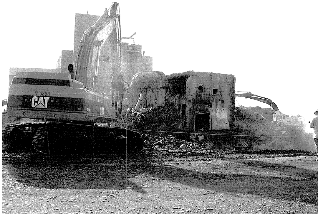
Figure 4-1. Photographs Showing Exhaust Fan Room and Exhaust Tunnels Demolition in Progress.
