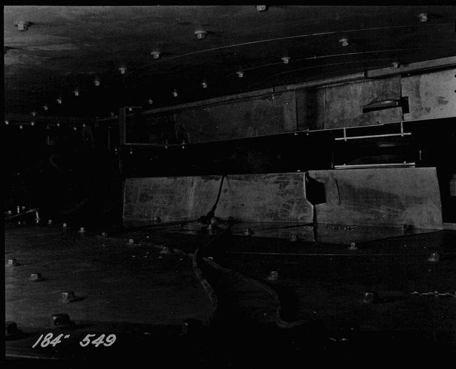
Figure 15a. View inside cyclotron facing the dee and showing the grounded "dummy dee".
