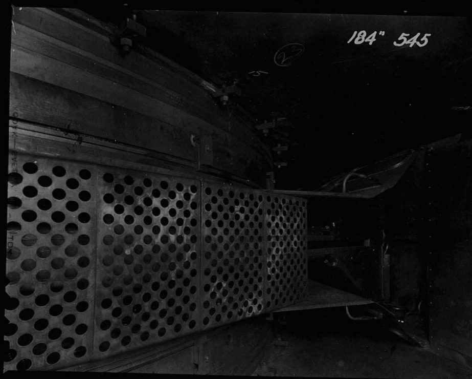
Figure 15b. View along edge of the dee showing rt discharge suppressing shields.
