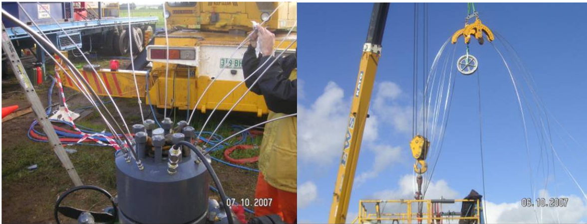
Figure 5. Assembling and deployment of the complete system was a complex and successful operation, these figures show the wellhead with flow tubes and cable connections, while on the right shows control of the u-tubes while inserting the integrated assembly
