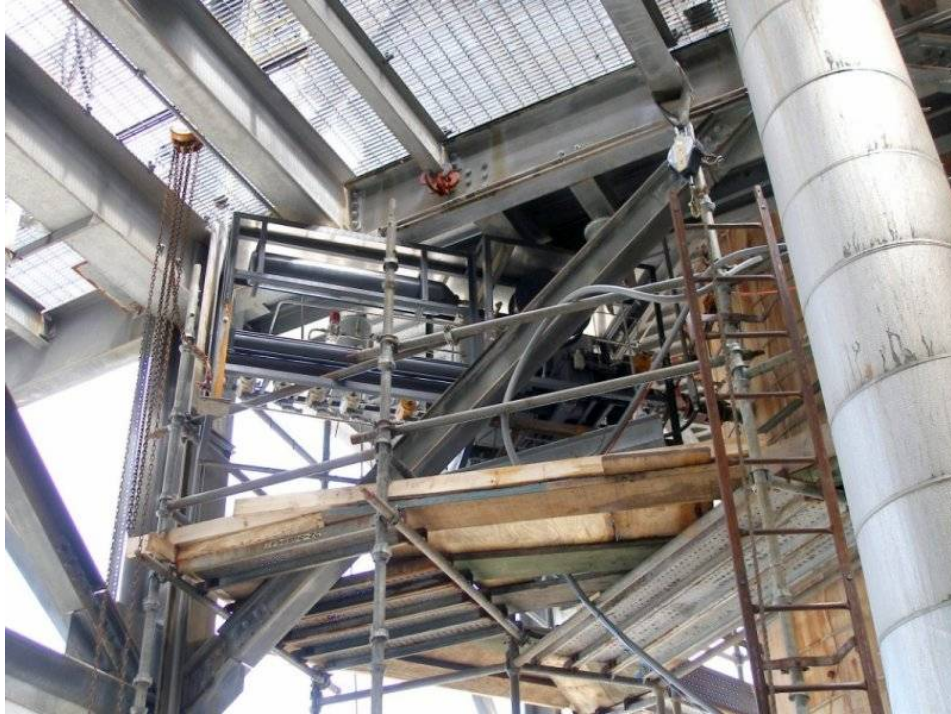
Figure 37. Generator unit mounted on the Wabash River gasifier
