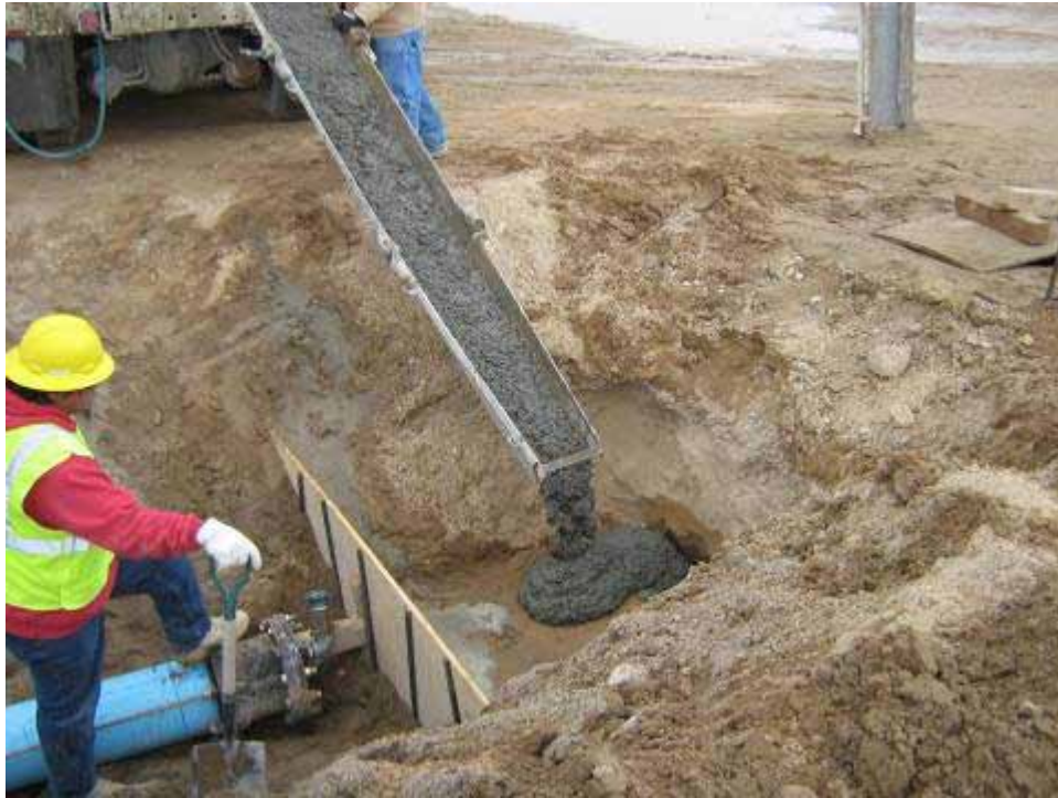
Photograph 17: CAS 06-19-03, Pouring Thrust Blocks for Water Line, 02/17/2009
