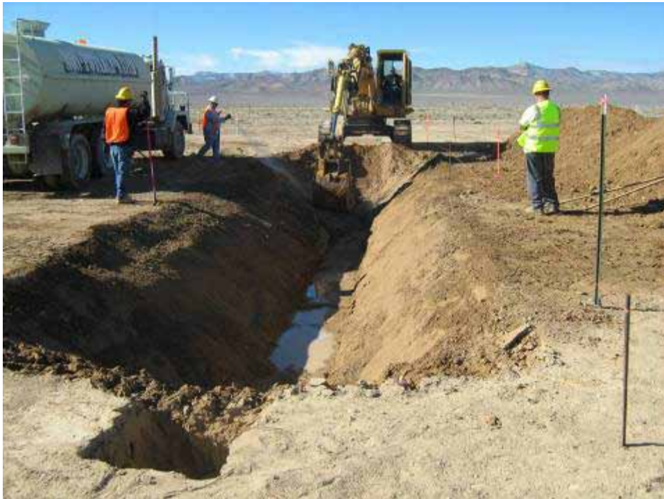
Photograph 10: CAS 06-19-03, Trench for New Water Line Location, 01/20/2009
