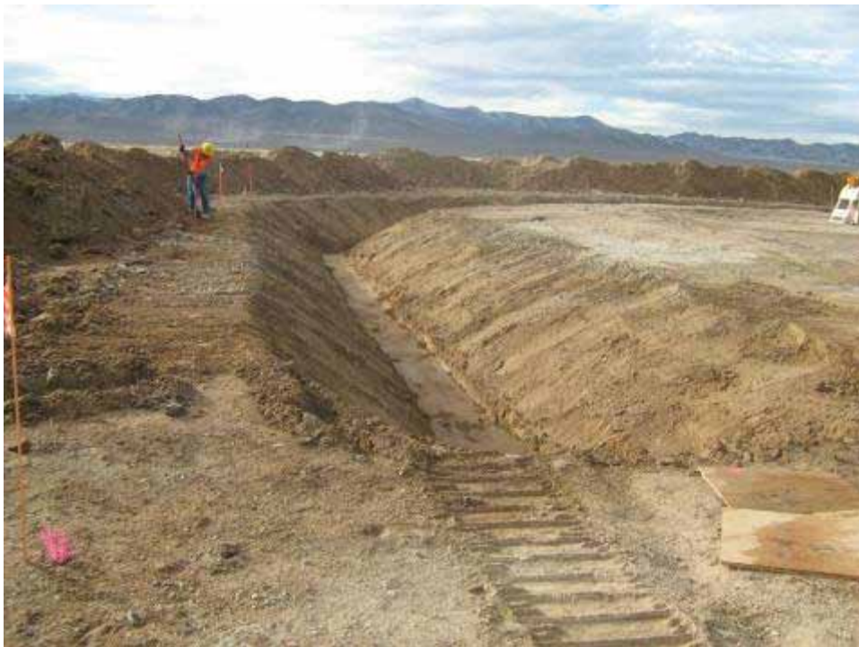
Photograph 12: CAS 06-19-03, Trench for New Water Line Location, 01/21/2009
