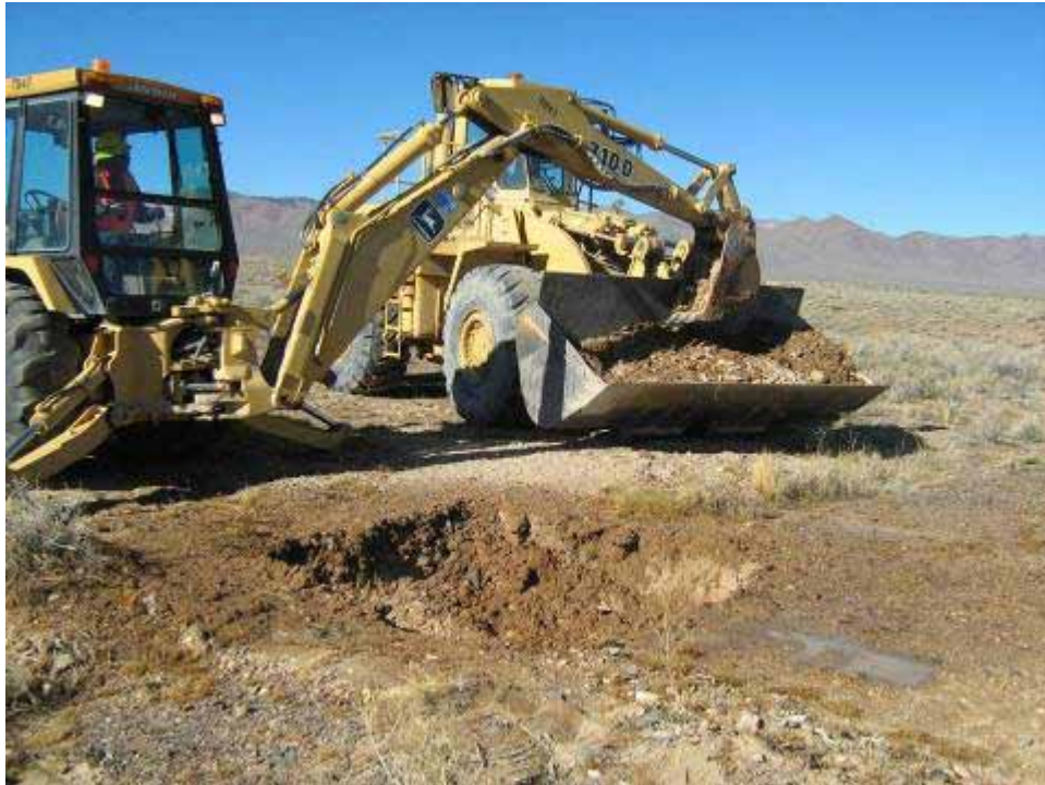
Photograph 3: CAS 04-99-01, Excavation of Radiologically Impacted Soil, 12/10/2008
