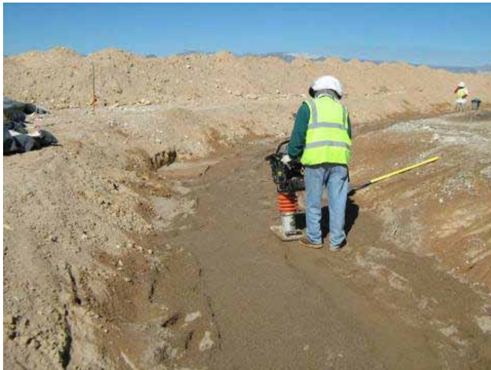
Photograph 18: CAS 06-19-03, Compaction of Soil over Water Line, 02/24/2009
