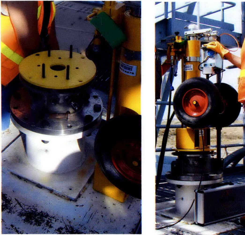
Figure 5. Riser Mounting Plate Connection to Spray Ring and Final Assembly.
