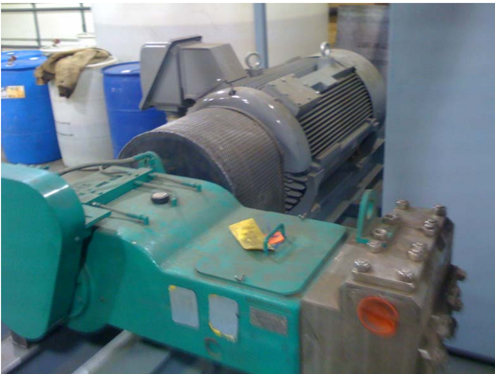
Figure 14 VFD Electric Driven HPSP, third view
