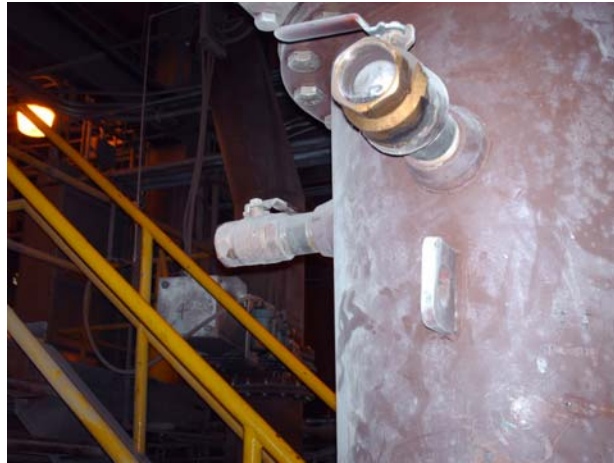
Figure 2.4. The perpendicular sampling ports.
