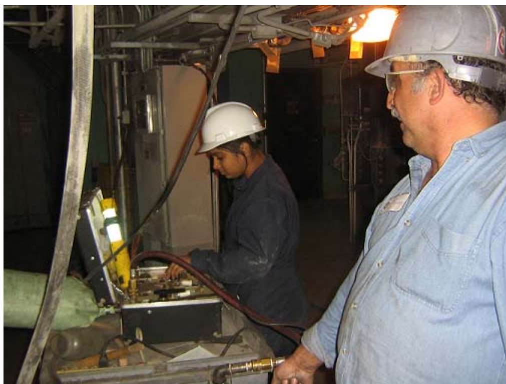
Figure 2.10. Frank Coen (GE Energy) and Rupali Panda (UAF) operating the Rotorprobe control box.
