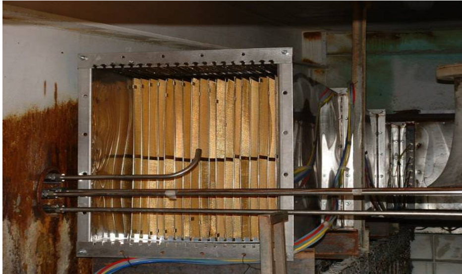
Figure 3-3. MerCAP™ Array Duct Section 1 Stanton Unit 10 Baghouse Compartment
