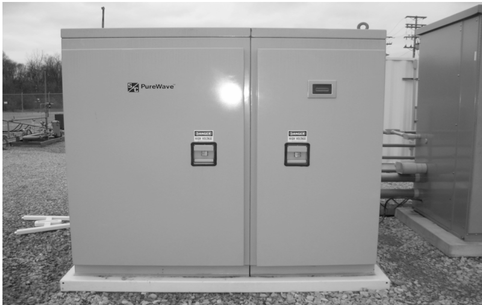
Figure 4. The Static Switch
