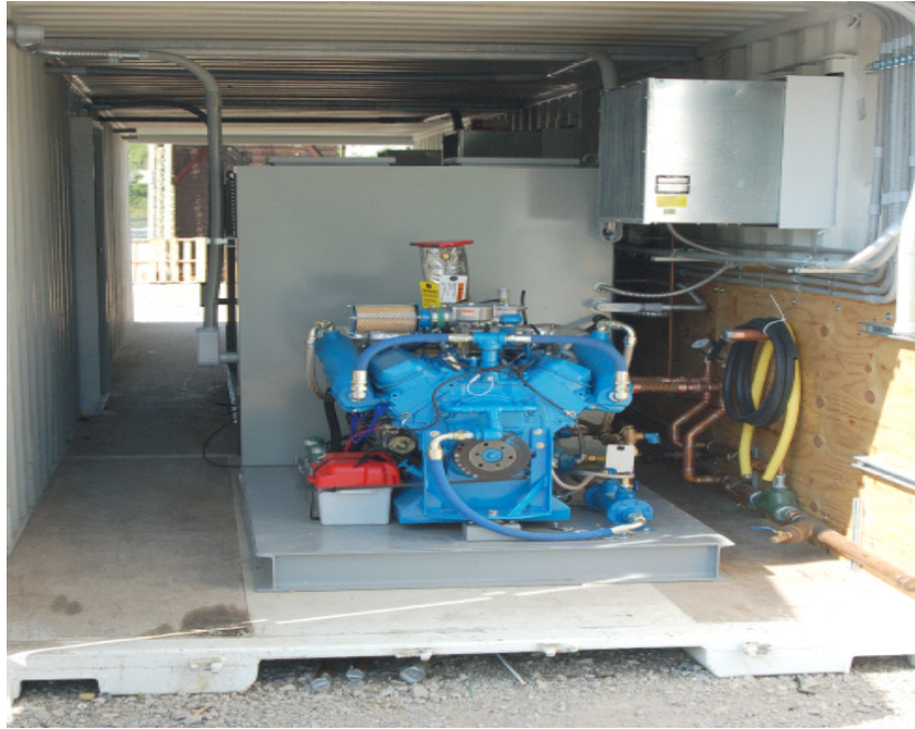
Figure 3. Tecogen Prime Mover with Inverter
