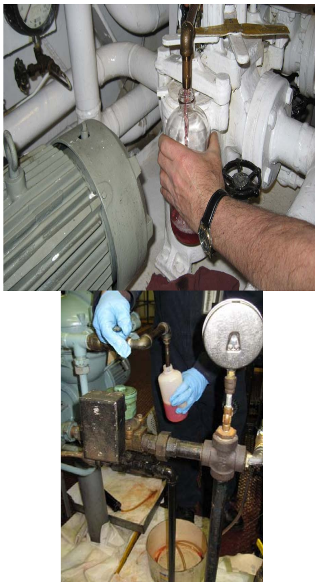
Figure 19. B5 samples being drawn on WSF vessels.
