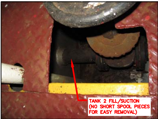
PHOTO 12-A FO STORAGE TANK 2 FILL/SUCTION
