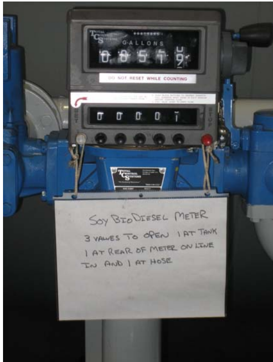
Figure 6. Meter to dispense soy biodiesel.
