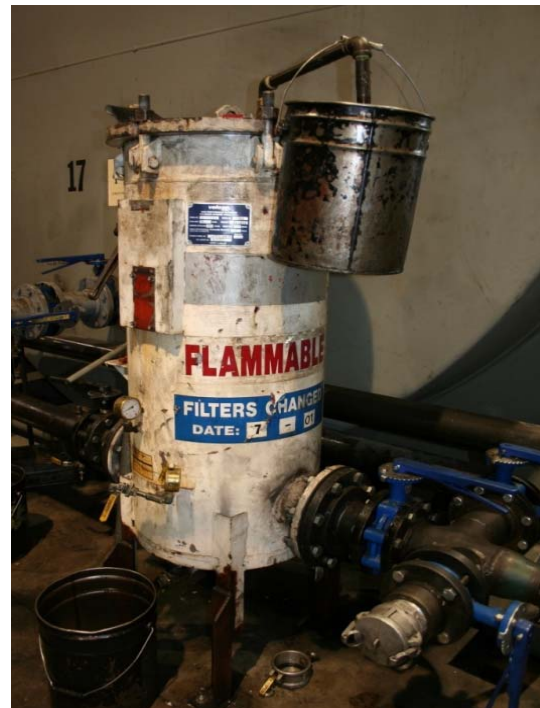
Figure 7. Filter to dispense soy biodiesel.
