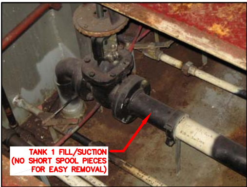
PHOTO 10-C FO STORAGE TANK 1 FILL/SUCTION
