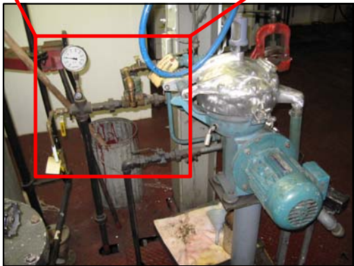
PHOTO 12-C EXISTING PURIFIER SAMPLE LINES (NO MODIFICATION REQUIRED)
