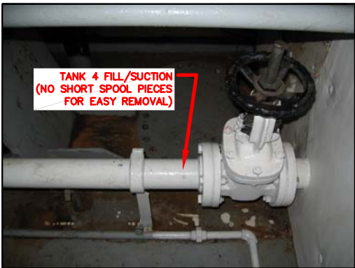
PHOTO 10-A FO STORAGE TANK 4 FILL/SUCTION
