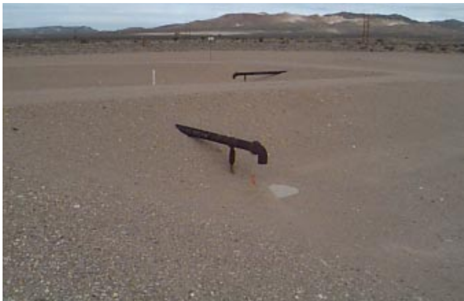
Figure 2-2 Photo taken on 09/18/97 facing northwest. The east lagoon is in the foreground. The iron outlet pipe can be seen in the west lagoon in the background and the iron overflow pipe connecting the two lagoons can be seen in the foreground. (IT, 1997b)
