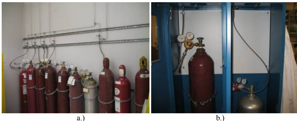
Figure 2: Process gas storage capabilities in the Advanced Materials Laboratory at BSU. a.) Photograph of the ultra high purity gas cylinder distribution manifold containing argon, nitrogen, 20% oxygen with a nitrogen balance, and 6.28% hydrogen with a nitrogen balance. b.) Photograph of the open volatile gas cabinet containing ultra high purity hydrogen and ammonia for gas storage and distribution.
