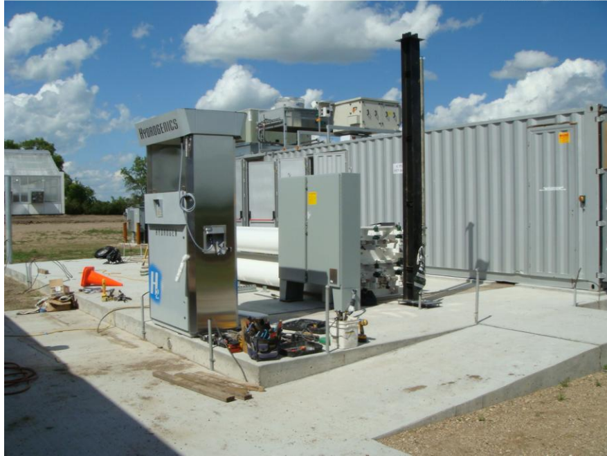
Figure 15. Photo of the gas control panel and hydrogen dispenser installed.
