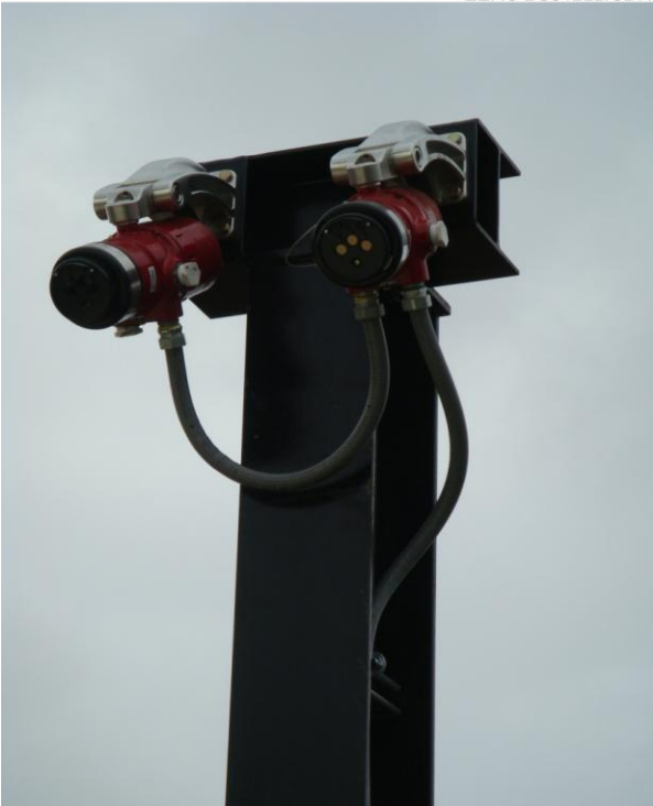
Figure 20. Photo of the infrared flame detection sensors.
