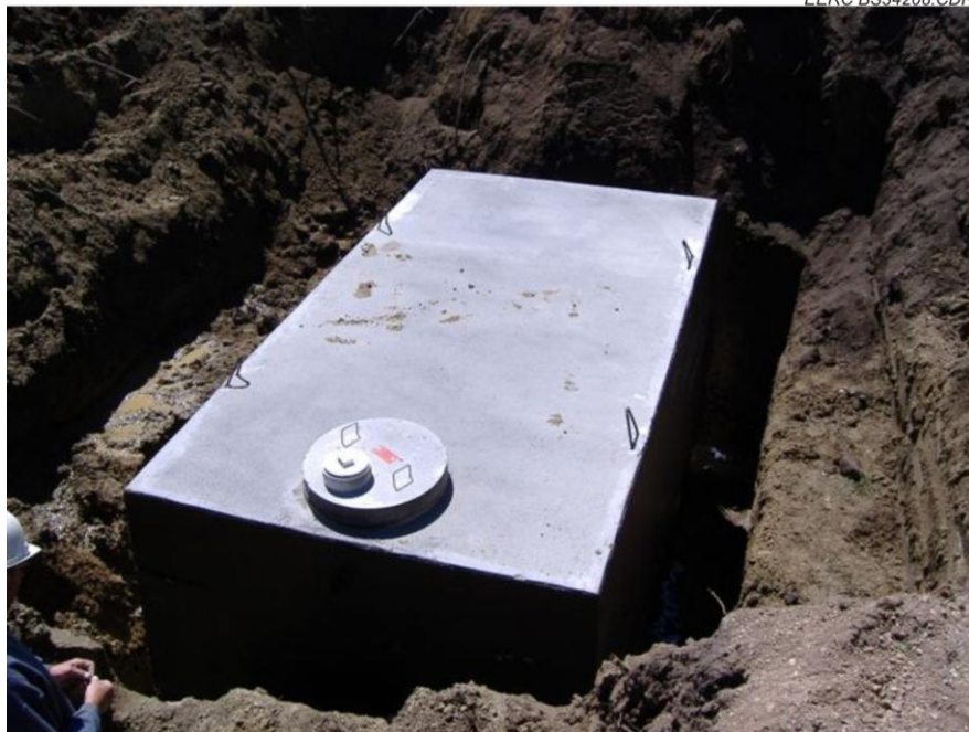
Figure 17. Photo of discharge tank installed.
