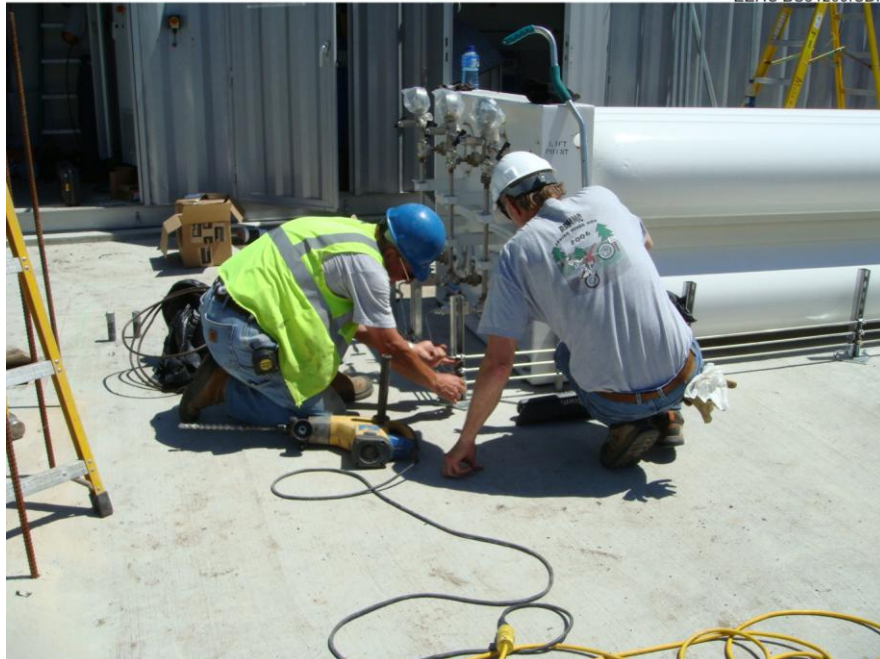
Figure 16. Photo of ICS personnel installing hydrogen piping.
