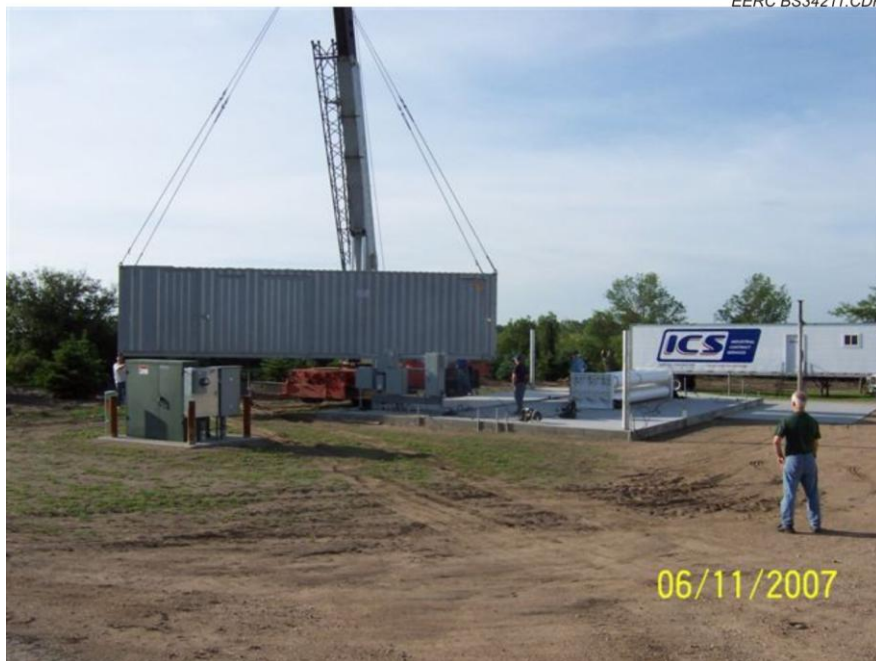
Figure 14. Photo of hydrogen system being set in place.
