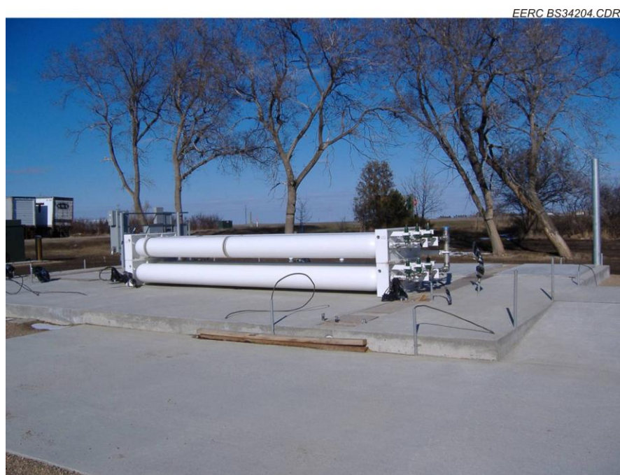
Figure 6. Photo of the hydrogen storage assembly.
