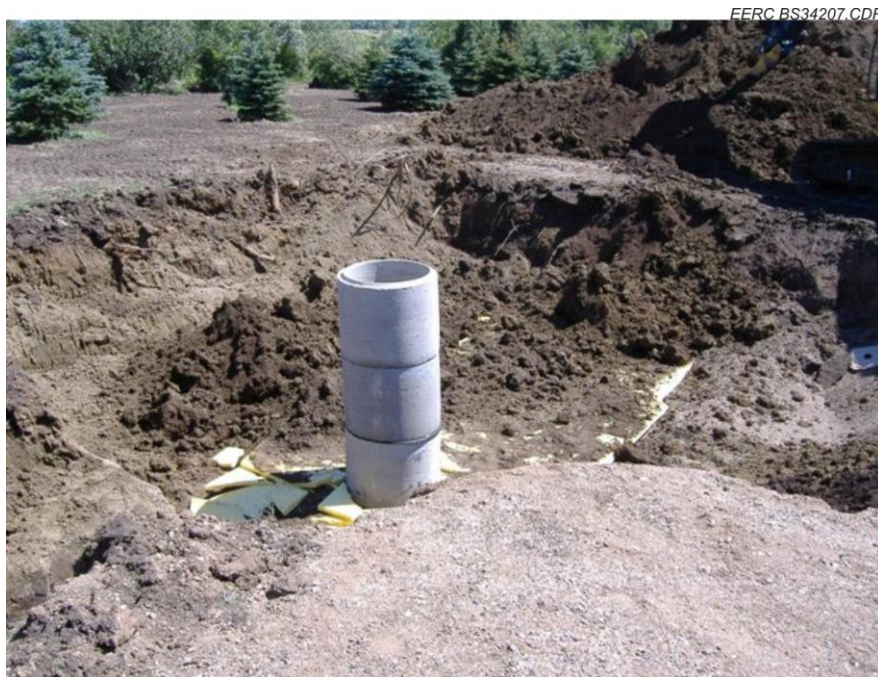
Figure 18. Photo of discharge tank access riser installed.
