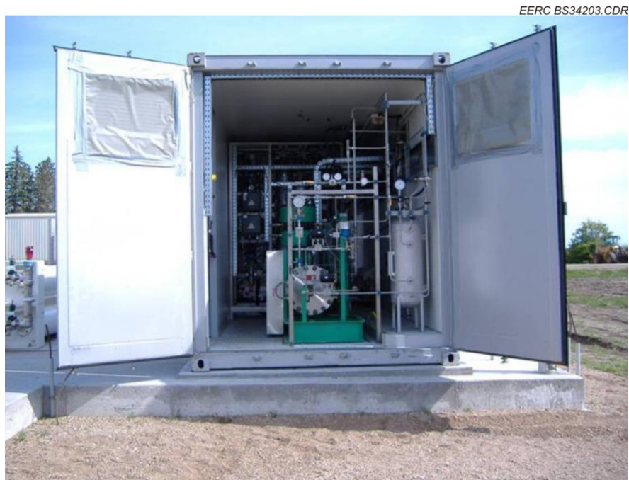
Figure 5. Photo of the hydrogen production area (hydrogen compressor in the foreground).
