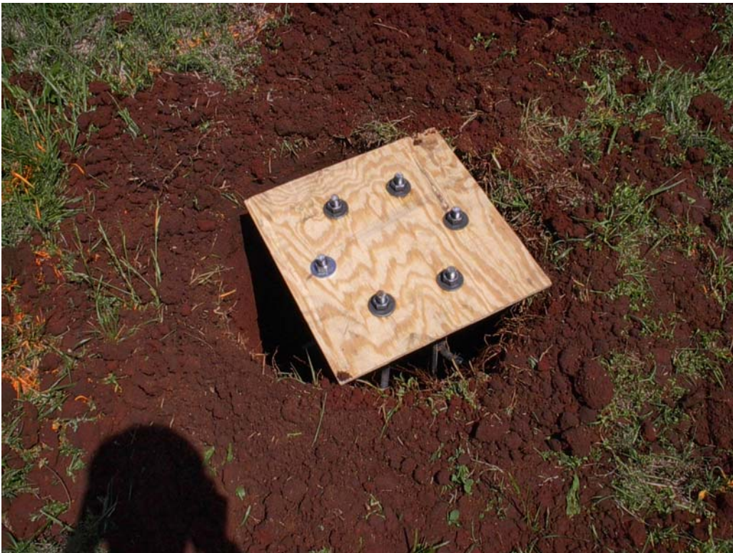
Rebar Cage Installed with J-Bolts Braced by Plywood
