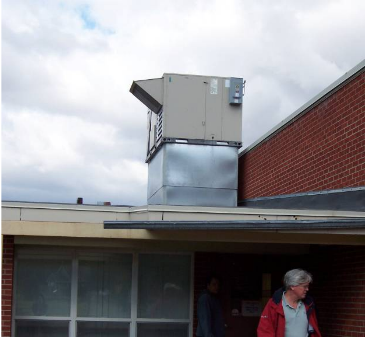
St. Ignatius (roof mounted propane heater)
