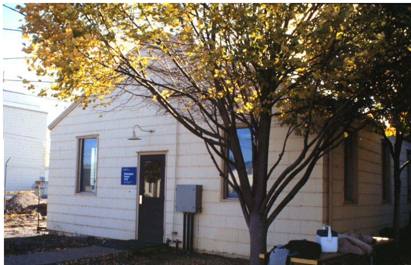
The facility was turned over for demolition in January 2007.
