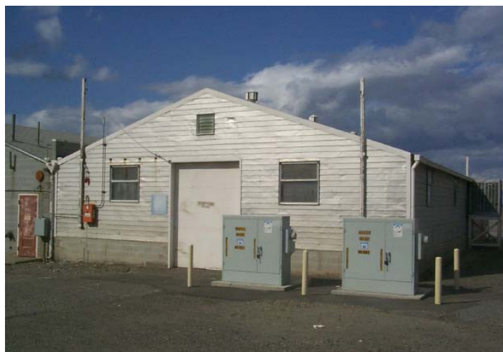
The 3731 Building was vacated and turned over for demolition in August 2005.
