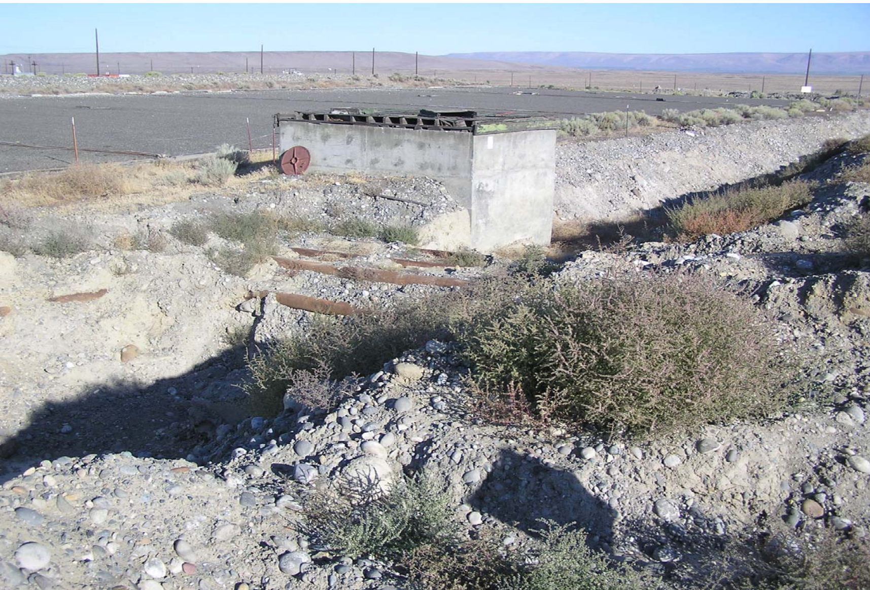
Photograph B-2. Exposed Pipelines in Excavation, East of 126-B-2.
