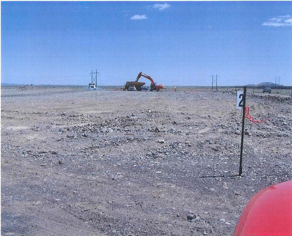
Photograph B-2. 118-C-1 Burial Ground (Beginning of Remedial Activities).
