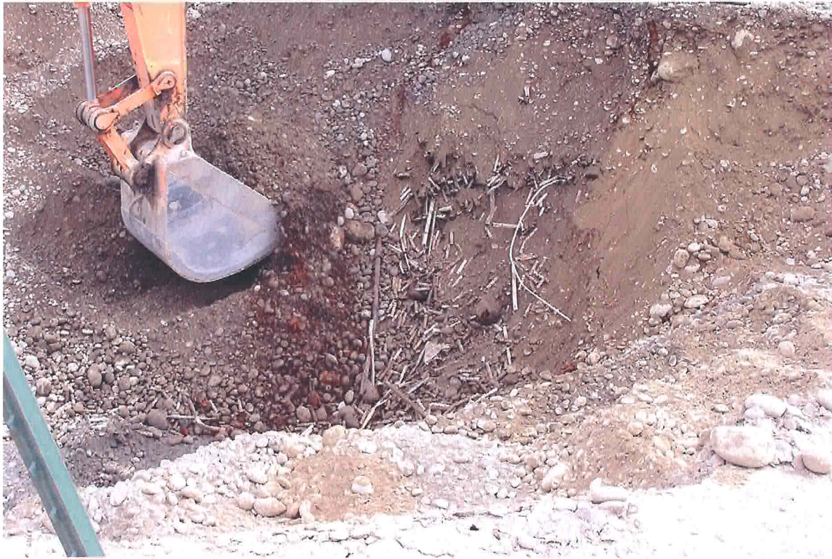
Photograph B-6. Excavation of Spacers and Soils at the 118-C-1 Burial Ground.
